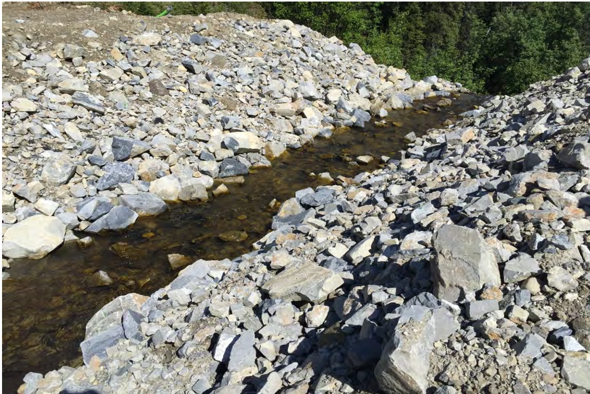
Photo 17: Channel through the North Creek Dyke following removal of the CMP culvert
