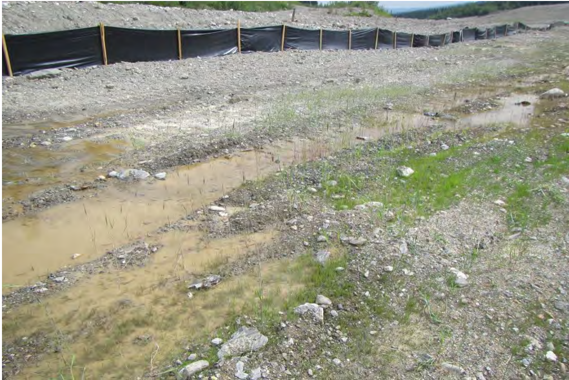
Photo 16: Silt fences for TSS management
