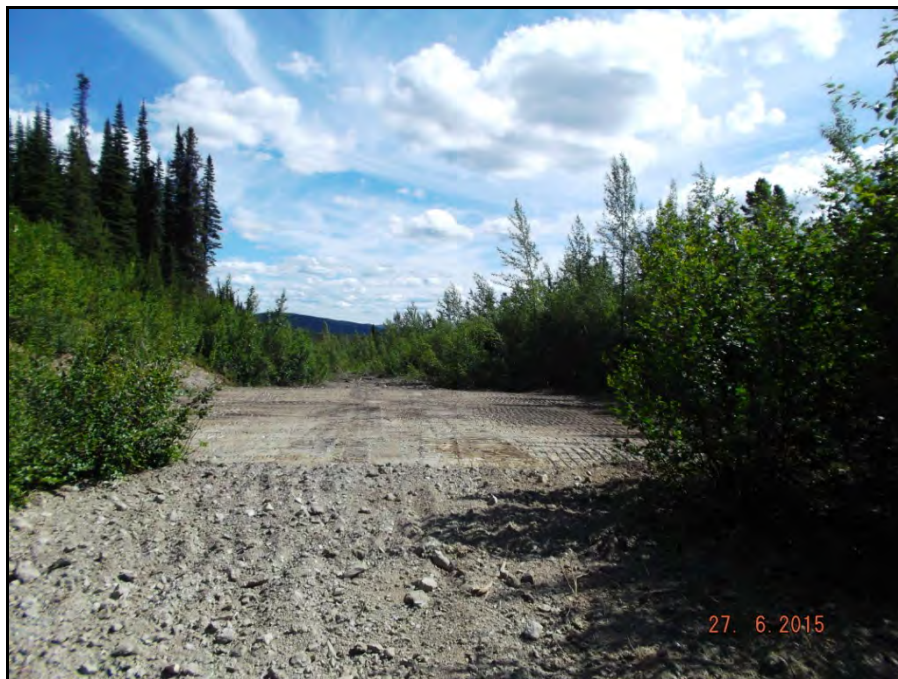
Photograph 10: Helipad for post-closure monitoring constructed near MH28/MH28-A during road decommissioning (road shown decommissioned at both ends) (June 27).
