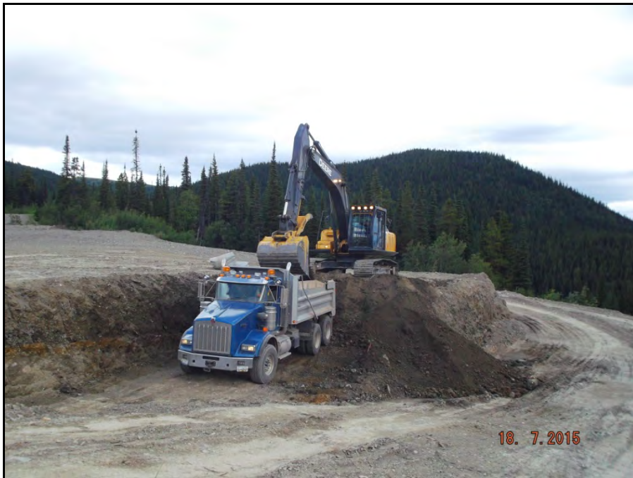
Photograph 18: Material from former mill camp facilities area being excavated and hauled to various capping locations around the mill area (July 18).
