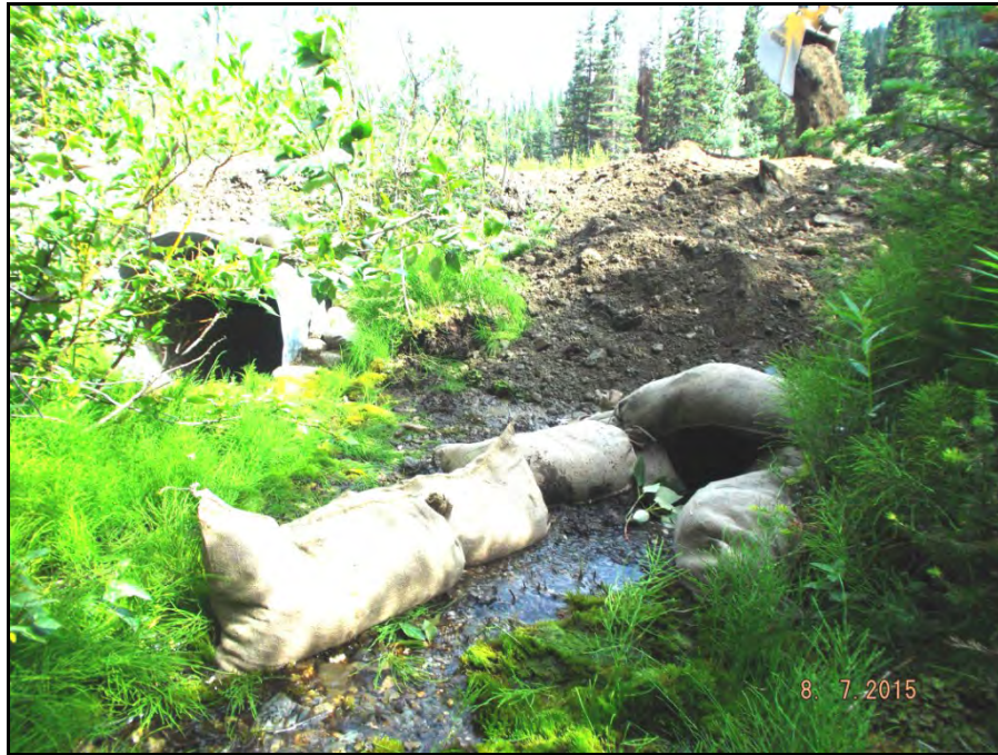
Photograph 15: Burnick Creek diverted into HDPE pipe using sand bags (right) to allow removal of culvert (left) in the dry (July 8).
