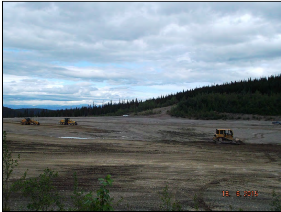
Photograph 7: Bulldozers and graders grading the surface of the North Pond after the grade had been raised and all ponded water had been pushed to the south (June 18).
