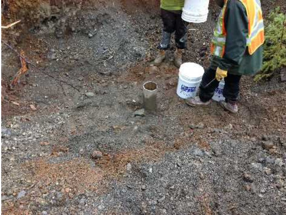
Photo 1: Water well TH01-90 cut down.
