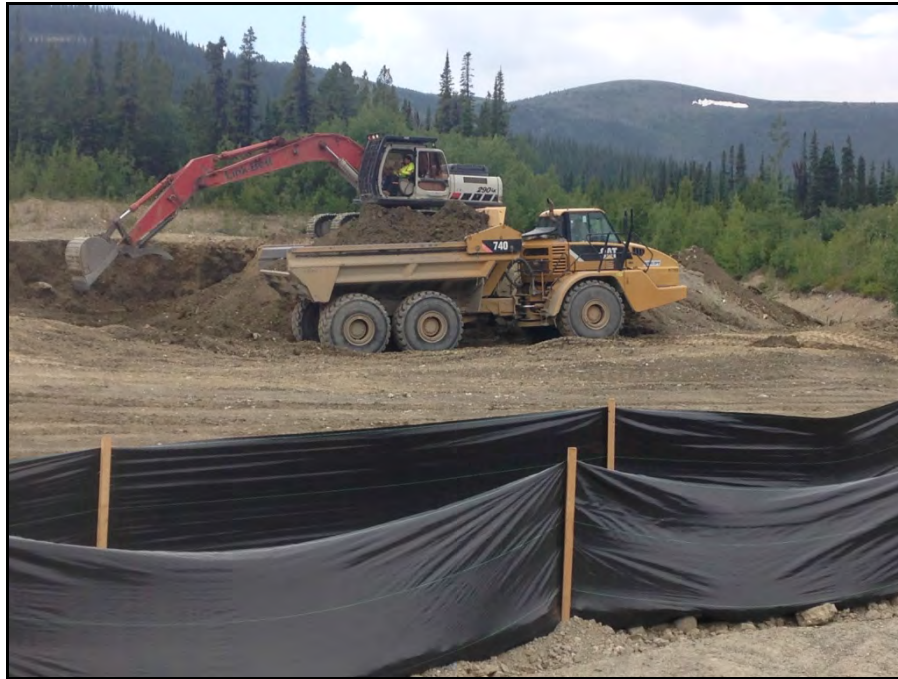
Photograph 9: Norcope loading rock truck at Borrow Pit “G” with former Reclaim Dam material for haul to Jewelbox for capping of the reclaimed waste rock dump surface (June 23).
