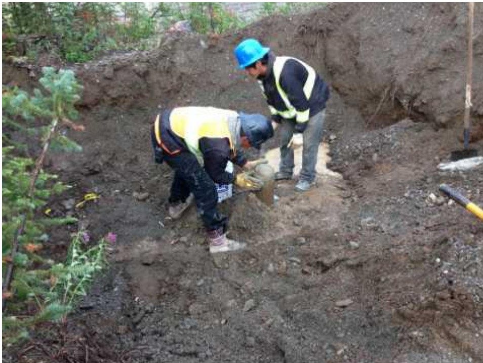
Photo 2: Lyon laborers installing grout cap for TH01-90.
