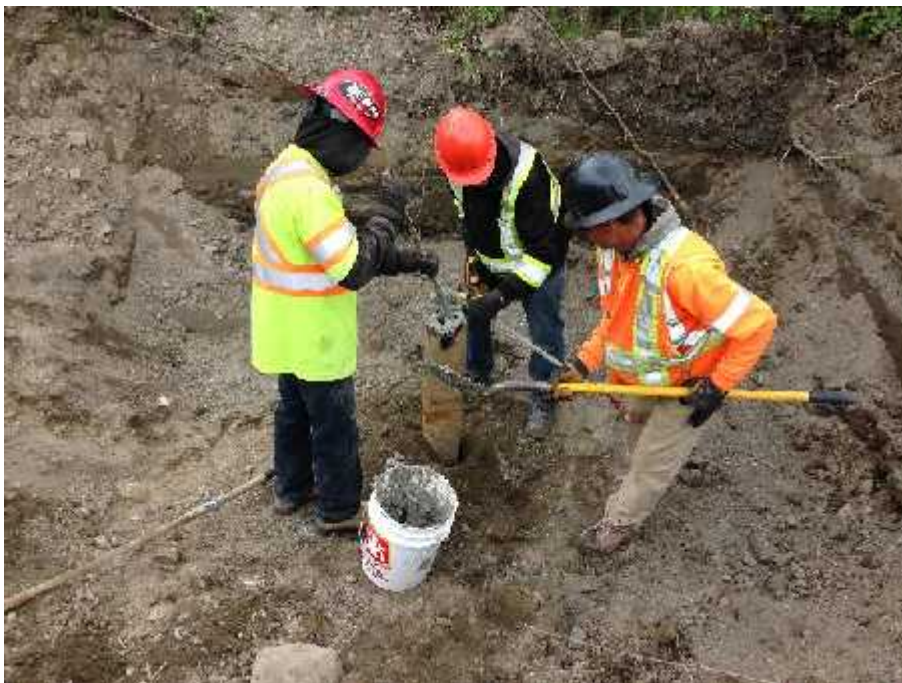
Photo 2: Lyon laborers installing grout cap of TH16-91.
