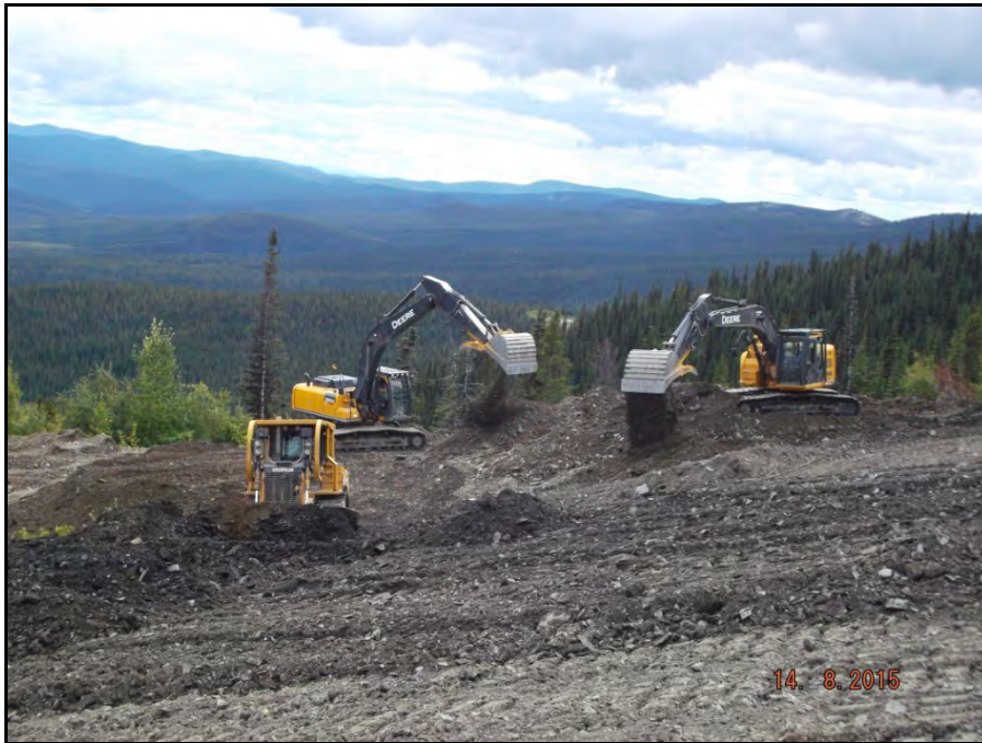
Photograph 30: Decommissioning of Jewelbox switchbacks, with two excavators and one bulldozer moving material up the slope (August 14).
