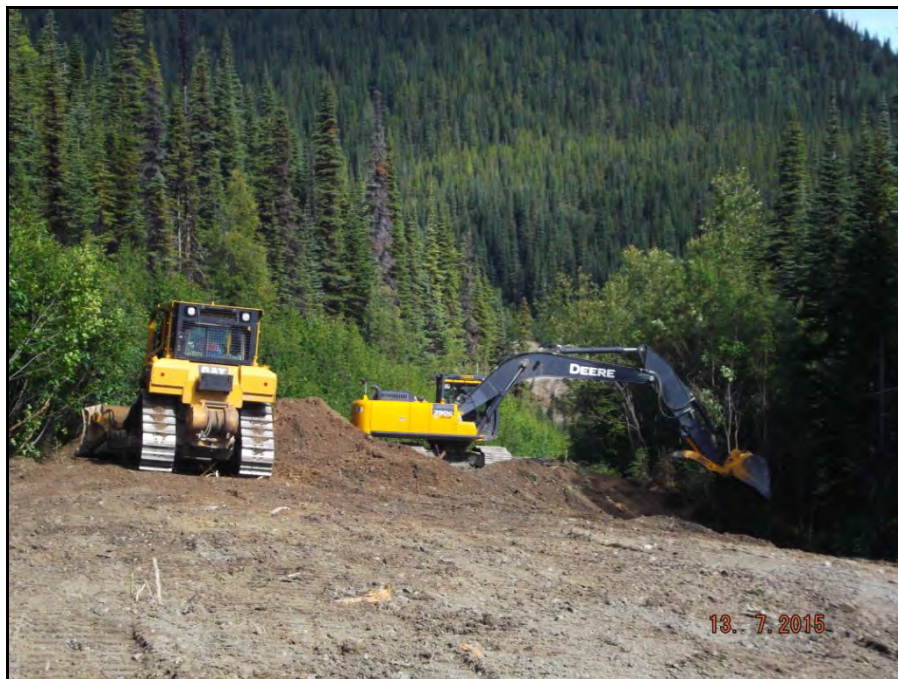
Photograph 16: Decommissioning of short access road with excavator bringing material up the slope and bulldozer shaping final surface (July 13).
