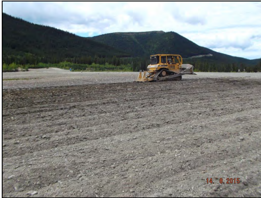
Photograph 31: Bulldozer with ripper attachment tilling soil at North Pond in preparation for alder tree planting (August 14).
