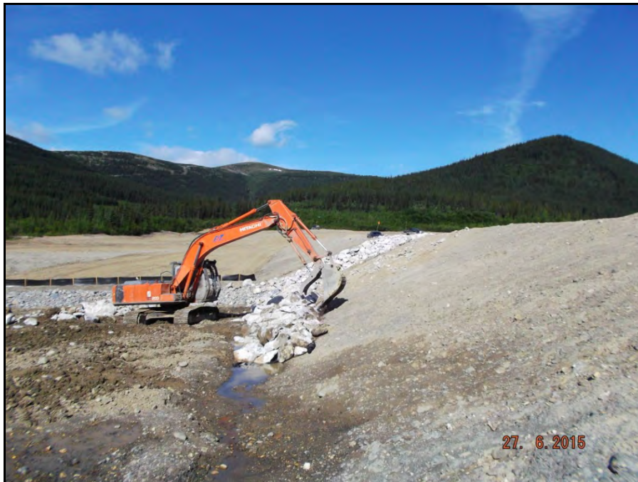
Photograph 4: Excavator placing rock from rock cofferdam along east downstream toe of SRS. Underlain geotextile was placed below rock material. Seepage seen running along toe was diverted away from toe following placement of rock fill (June 27).
