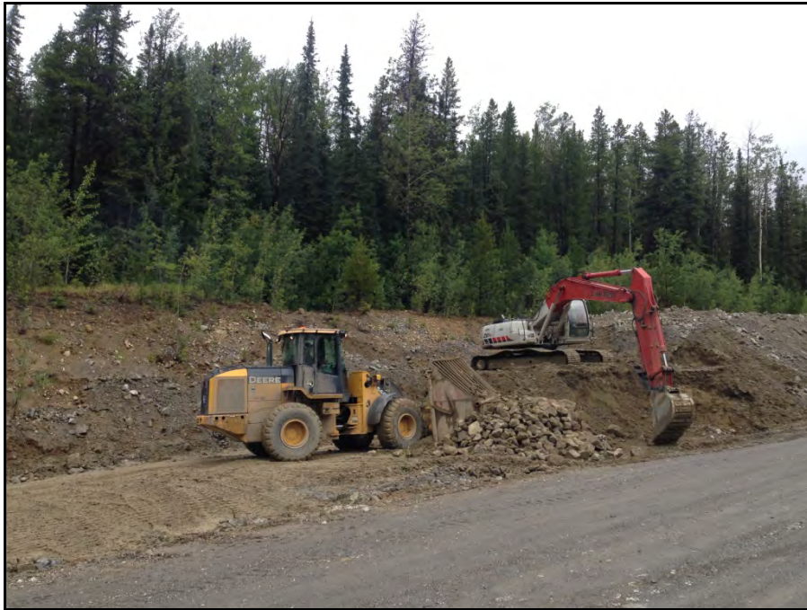
Photograph 19: Screening rock at km 17 quarry for use as erosion protection in site watercourses following culvert removal as part of road decommissioning (July 22).
