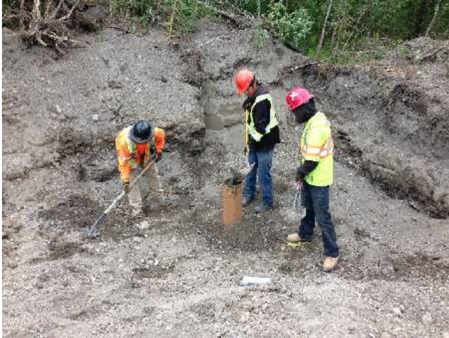
Photo 1: Lyon laborers shoveling sand into TH23-91.
