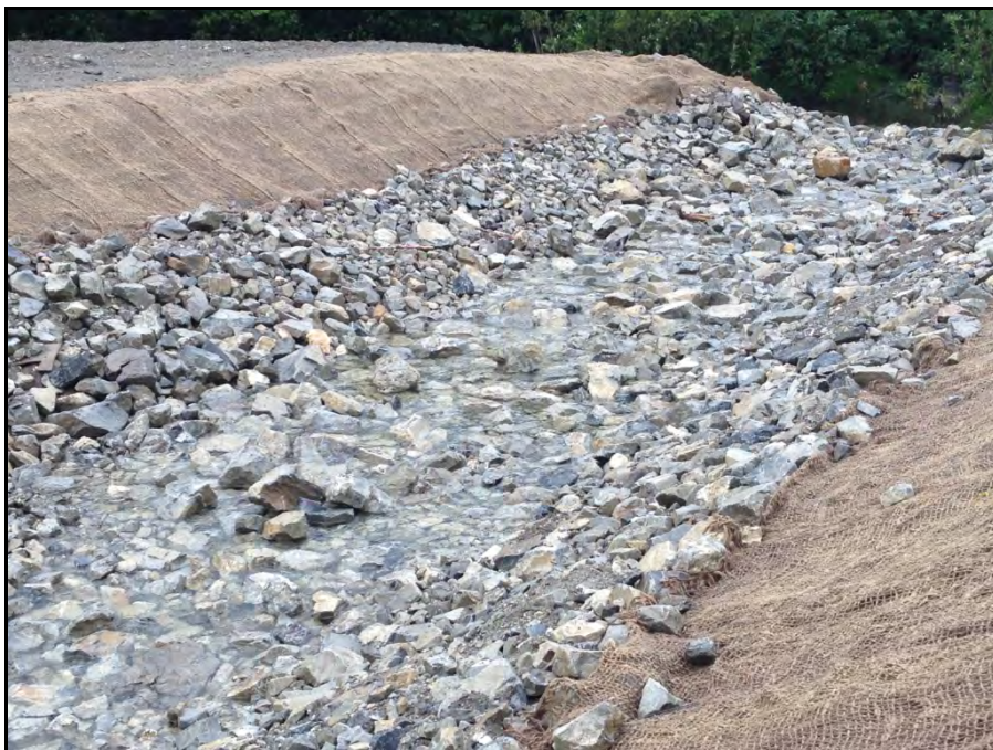
Photograph 20: Photo taken at Camp Creek crossing along short access road (MH-04 sample point) following road decommissioning and culvert removal. Erosion protection installed including rolled erosion control blanket on upper portion of slopes (July 22).
