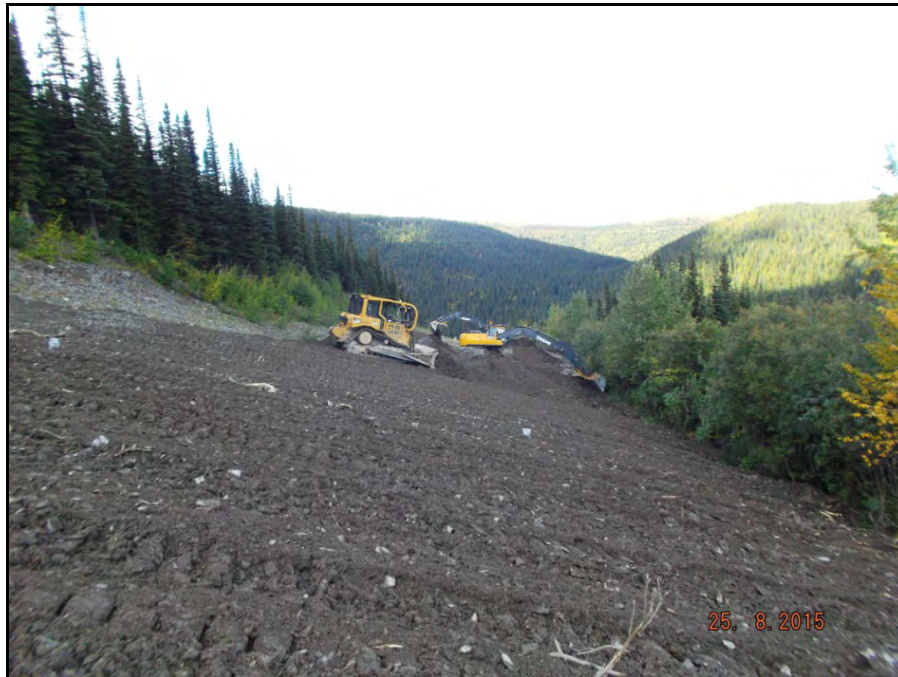
Photograph 34: Decommissioning of Jewelbox switchbacks, with two excavators bringing clean material up the slope and one bulldozer shaping the slope (August 25).
