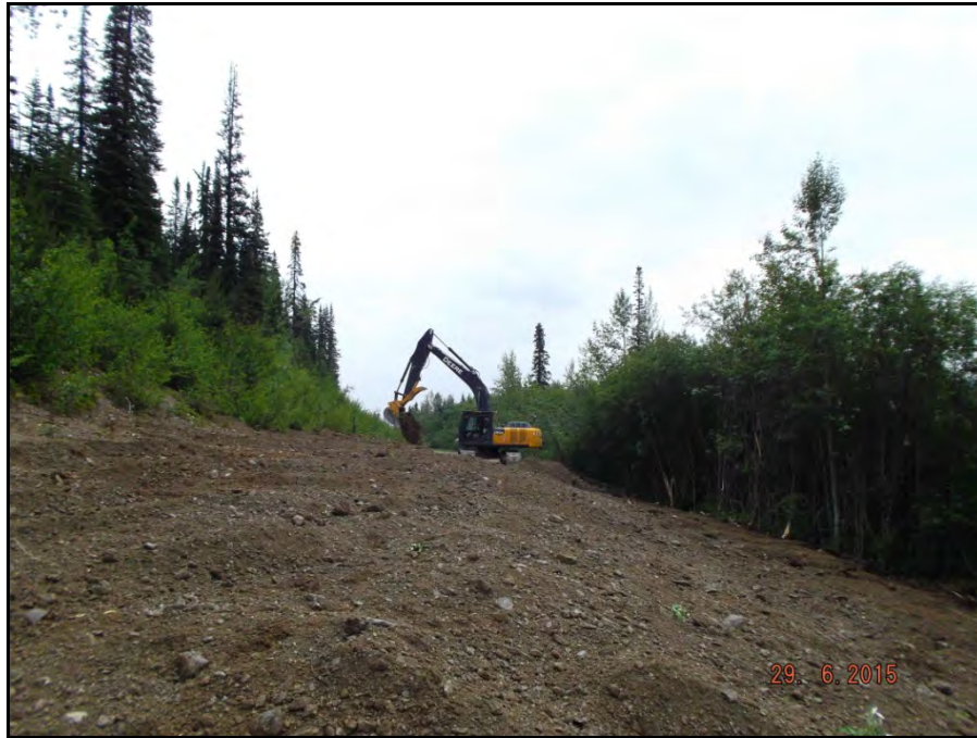
Photograph 11: Decommissioning of former South Dam east access road (June 29).
