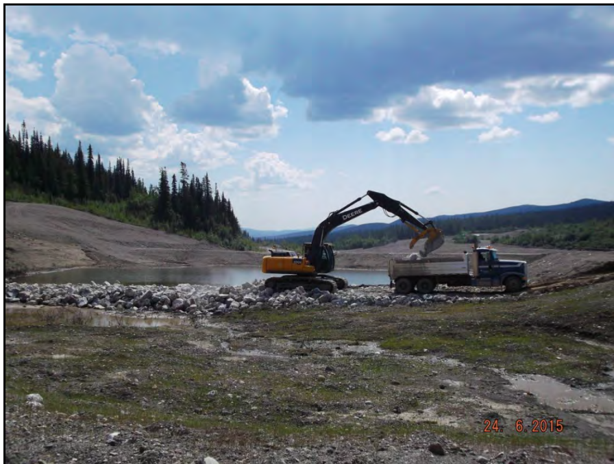
Photograph 2: Excavator removing top layer of rock from rock cofferdam in South Pond and placing in truck to haul to spillway and SRS to repair spring damage (June 24).
