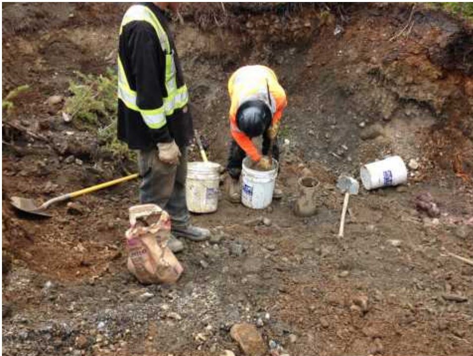
Photo 2: Lyon laborers mixing grout for capping TH05-90.
