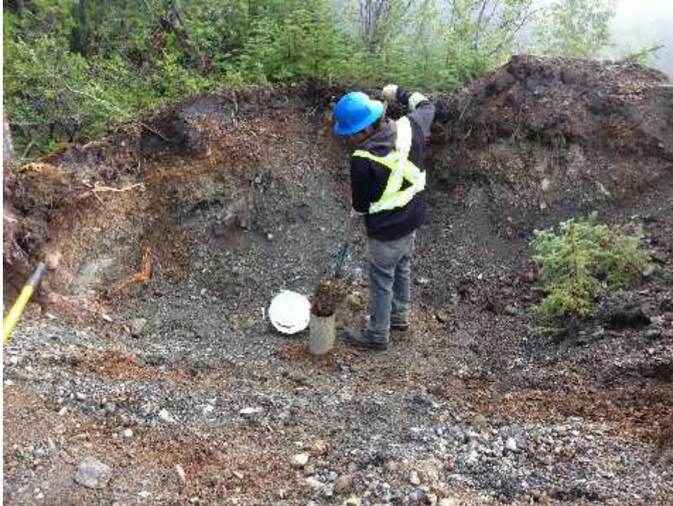
Photo 1: Lyon laborer shoveling sand into TH05-90.
