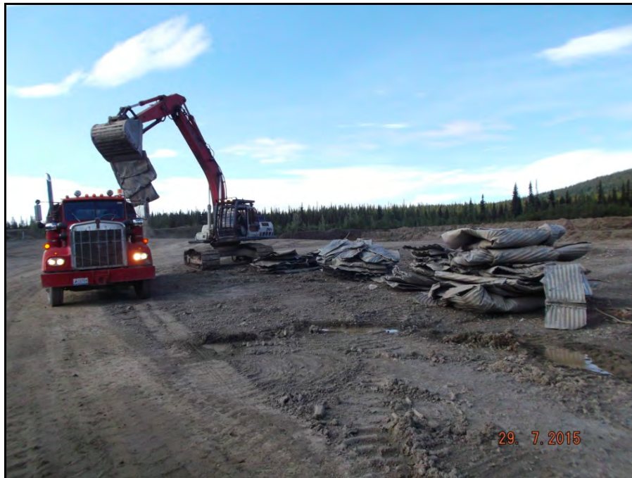
Photograph 24: Culverts from road decommissioning being crushed and loaded into truck for hauling to Watson Lake landfill (July 29).
