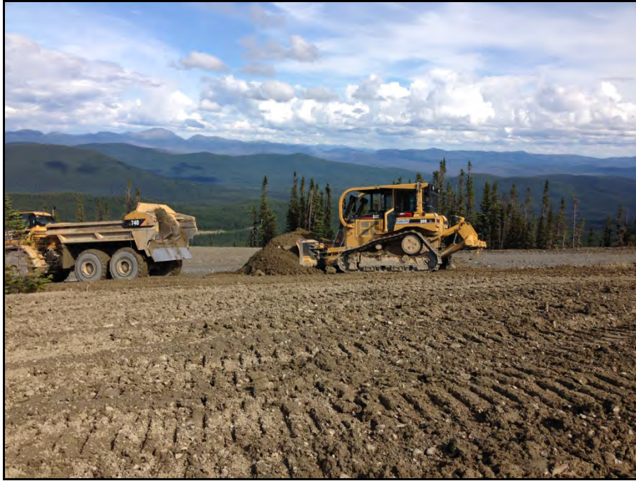
Photograph 21: Norcope placing minimum 200 mm thick lift of capping material across Jewelbox waste rock dump surface (July 23).
