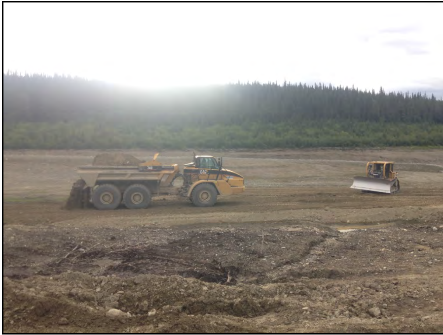
Photograph 27: Material from Borrow Pit “G” stockpile being spread as capping material across area in South Pond (August 03).
