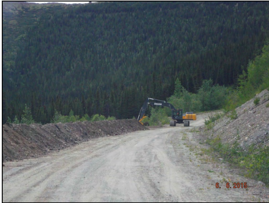
Photograph 5: Excavator constructing berm along long access road in preparation for hauling material from Borrow Pit "G" to Jewelbox for capping of the waste rock dump (June 6).
