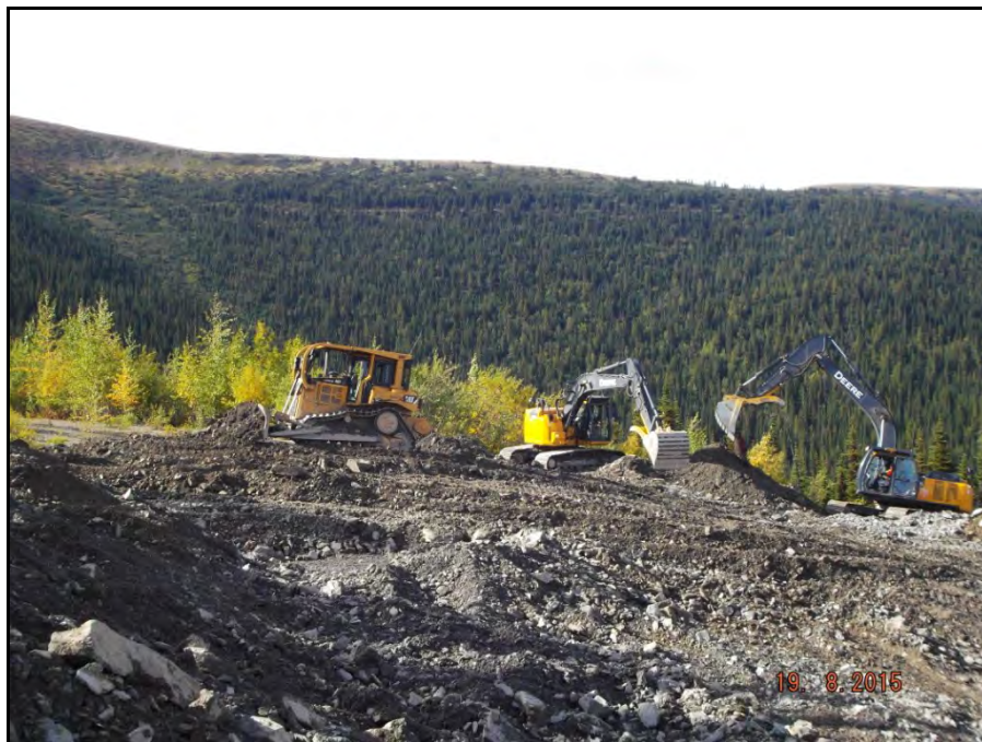
Photograph 32: Decommissioning of Jewelbox switchbacks, with two excavators and one bulldozer moving clean material up the slope (August 19).
