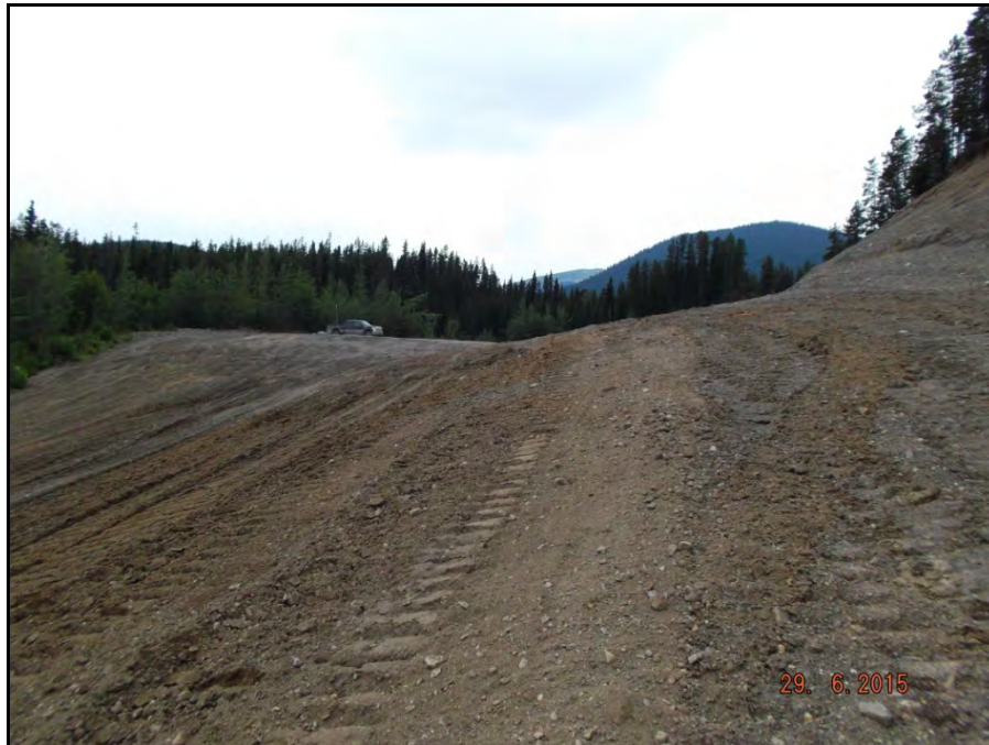
Photograph 12: Completed re-sloping / reshaping of gravel pit (north of landfill) (June 29).
