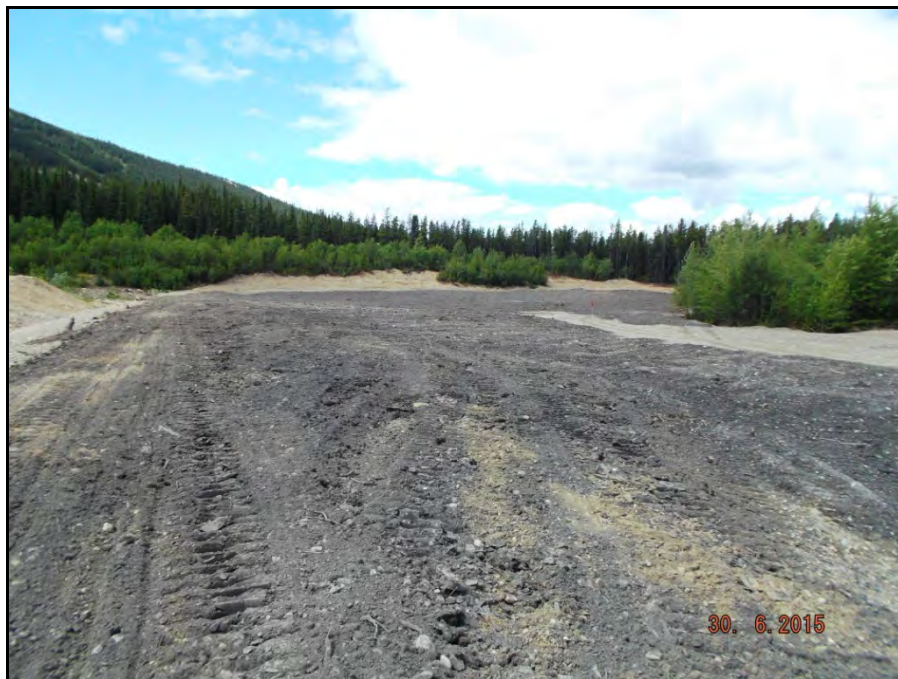
Photograph 14: Organic material stockpiled at landfill in 2014 spread across surface (June 30).
