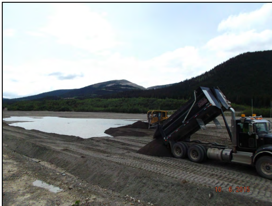
Photograph 6: Gravel from pit north of the landfill being dumped and spread at northeast corner of North Pond to raise the grade of the cover, push ponded water to the south, and promote drainage from the surface (June 10).
