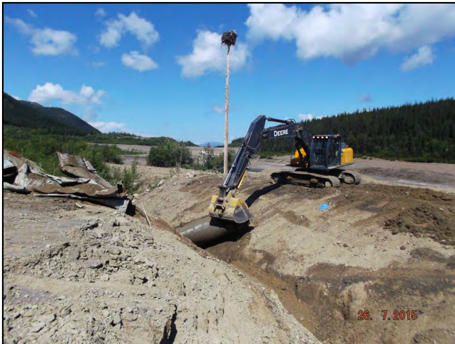
Photograph 22: Decommissioning of Camp Creek Diversion culverts and fill material (July 26).
