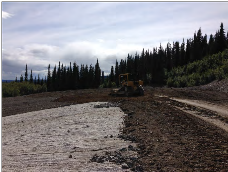
Photograph 26: Capping of former crusher area with material excavated from former mill camp facilities area. Rolled erosion blanket in photo was placed along the crusher slope (left) in 2014 (July 29).
