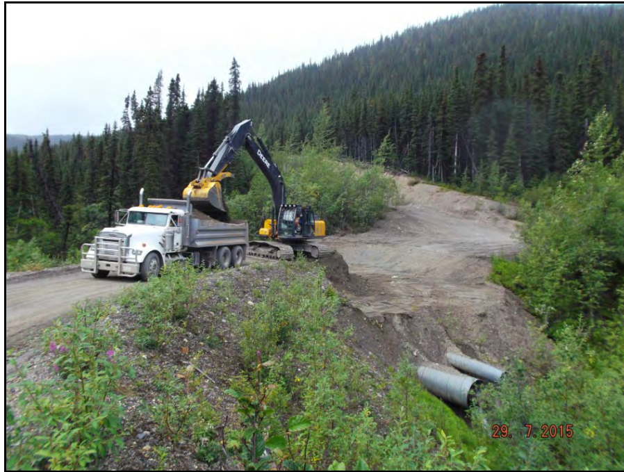
Photograph 25: Road decommissioning near North Creek crossing along Burnick 1200 access road (July 29).
