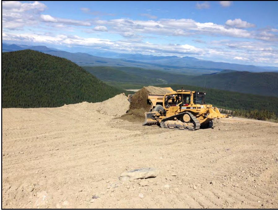
Photograph 17: Norcope spreading clean sand and gravel across reclaimed Jewelbox waste rock dump (July 16).
