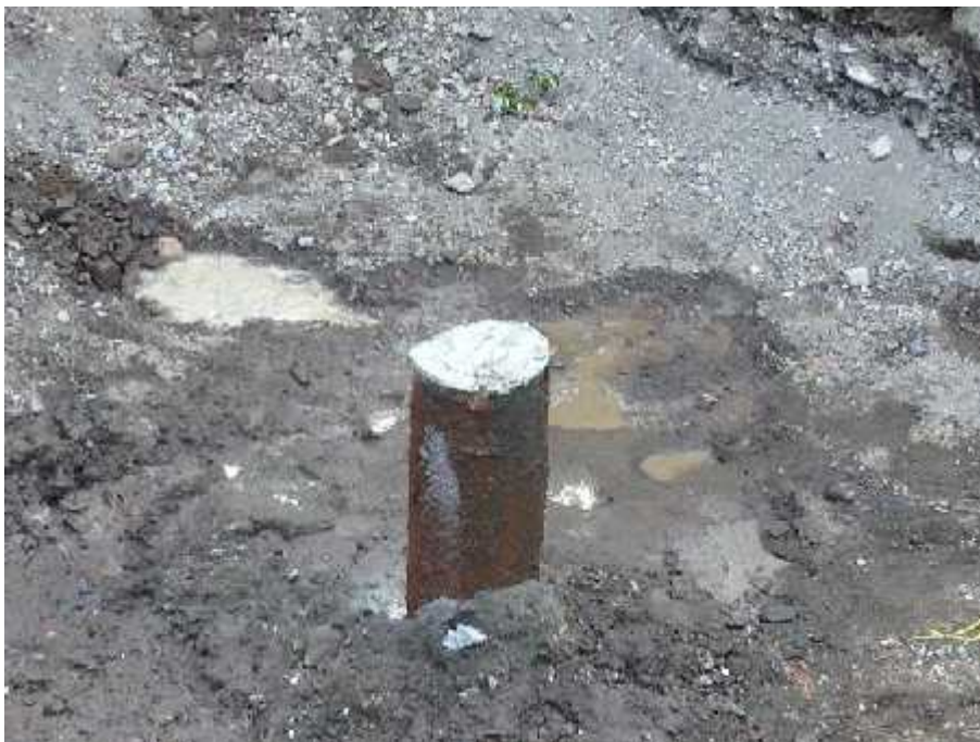
Photo 2: Grout cap of TH23-91.
