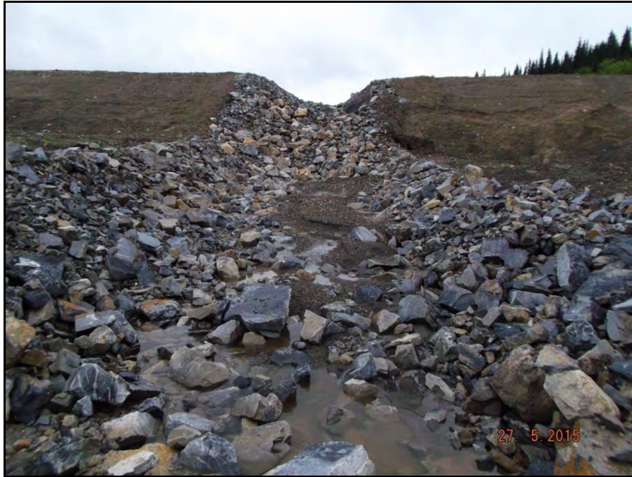
Photograph 1: Photo taken during spring inspection showing erosion on east downstream toe of SRS (right of photo) with sediment in channel and sloughing within spillway causing rock migration (May 27).
