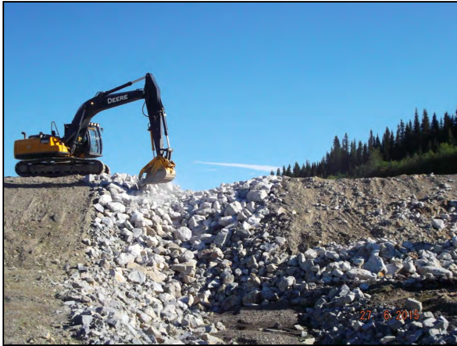
Photograph 3: Excavator placing additional rock in spillway and along east (right) downstream toe of SRS (June 27).
