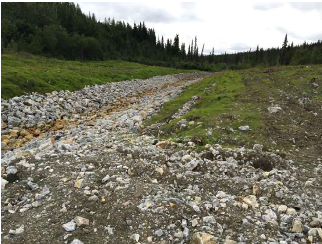
Photo 18: View Downstream of the Camp Creek Drainage Channel
