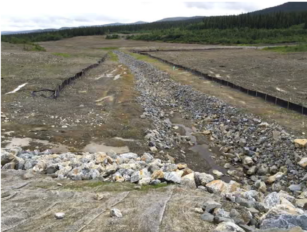
Photo 16: View downstream of the South drainage channel
