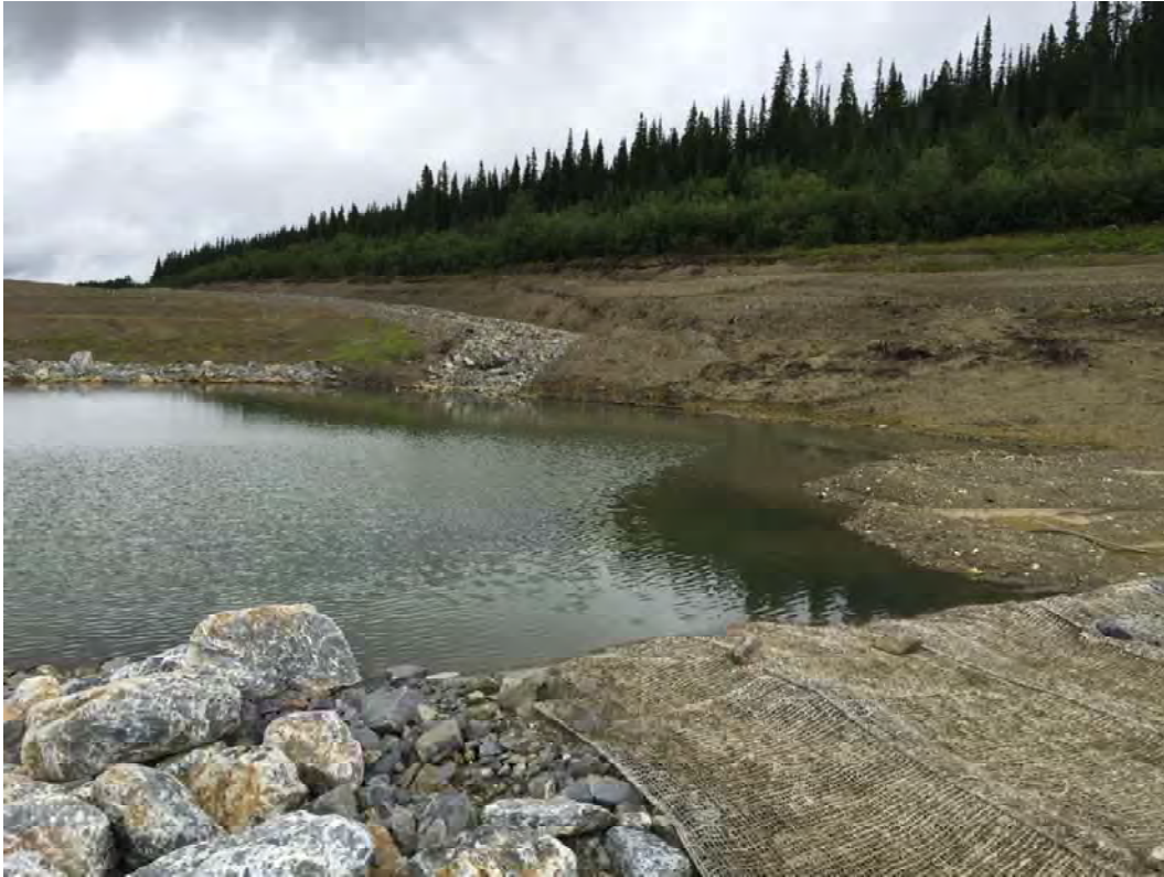
Photo 15: Sediment Pond and outlet from the North Drainage channel in background
