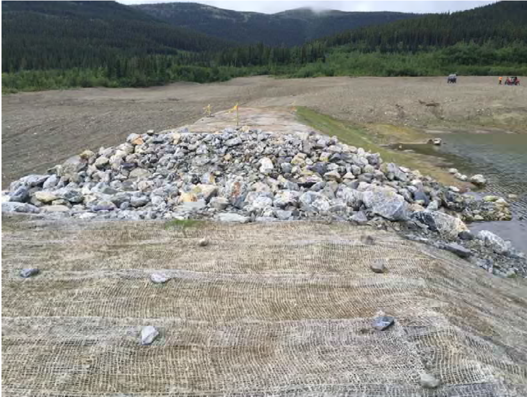
Photo 11: Spillway at Sediment Retaining Structure
