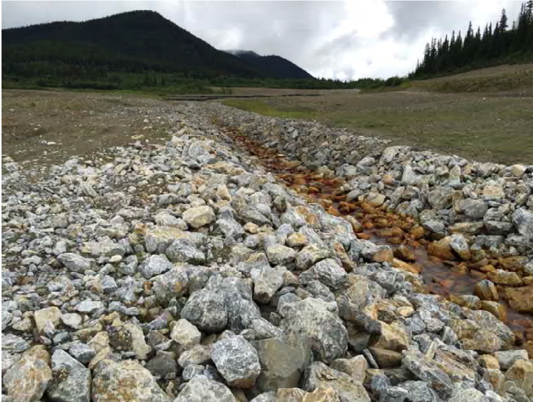
Photo 17: View upstream of the Camp Creek drainage channel
