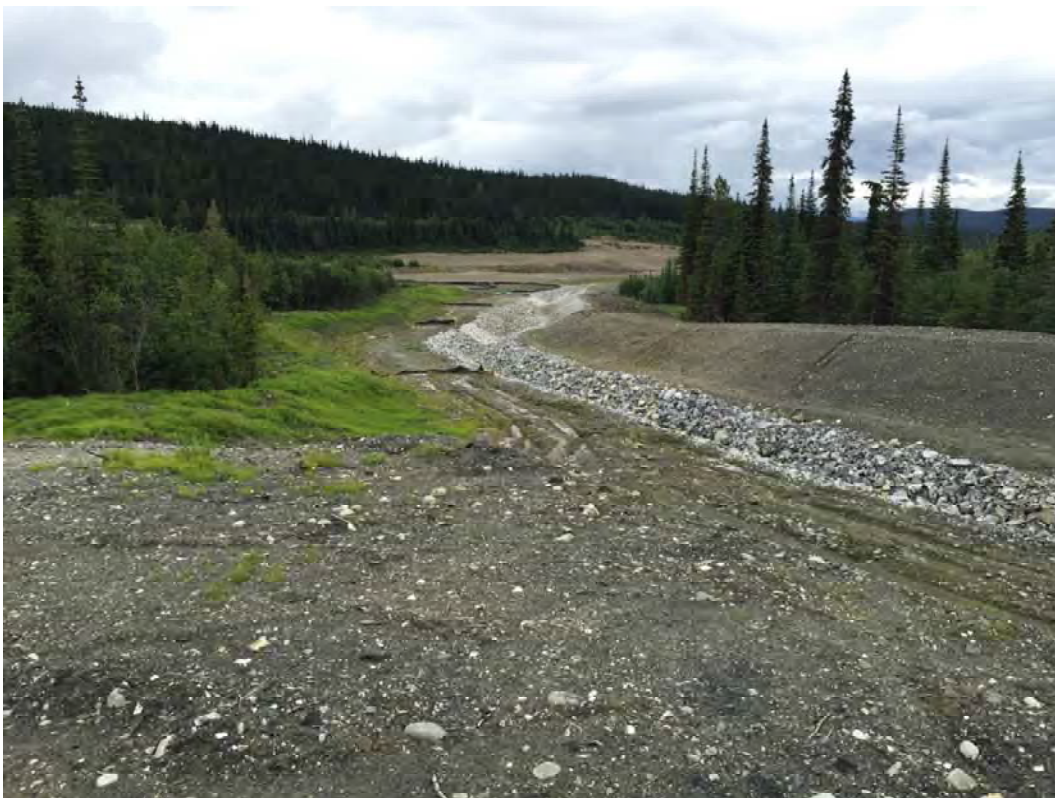
Photo 20: View downstream of the Camp Creek Drainage Channel
