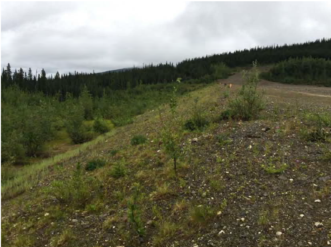
Photo 2: View East along the Downstream Face of the North Dam
