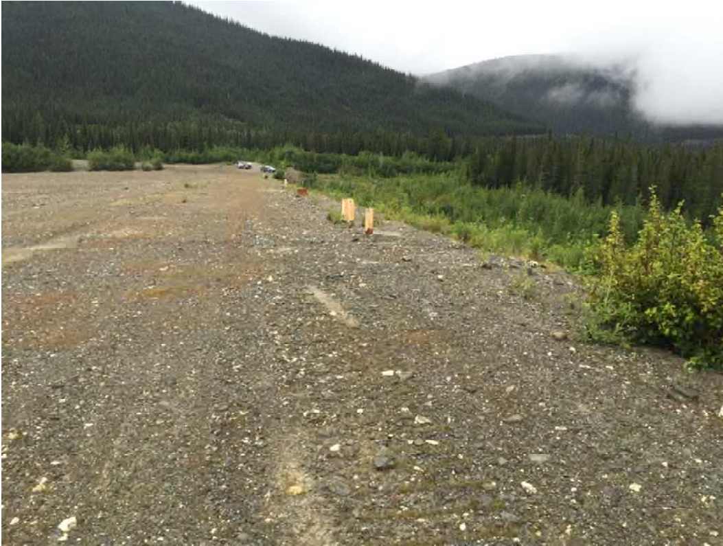
Photo 1: View West along the North Dam Crest
