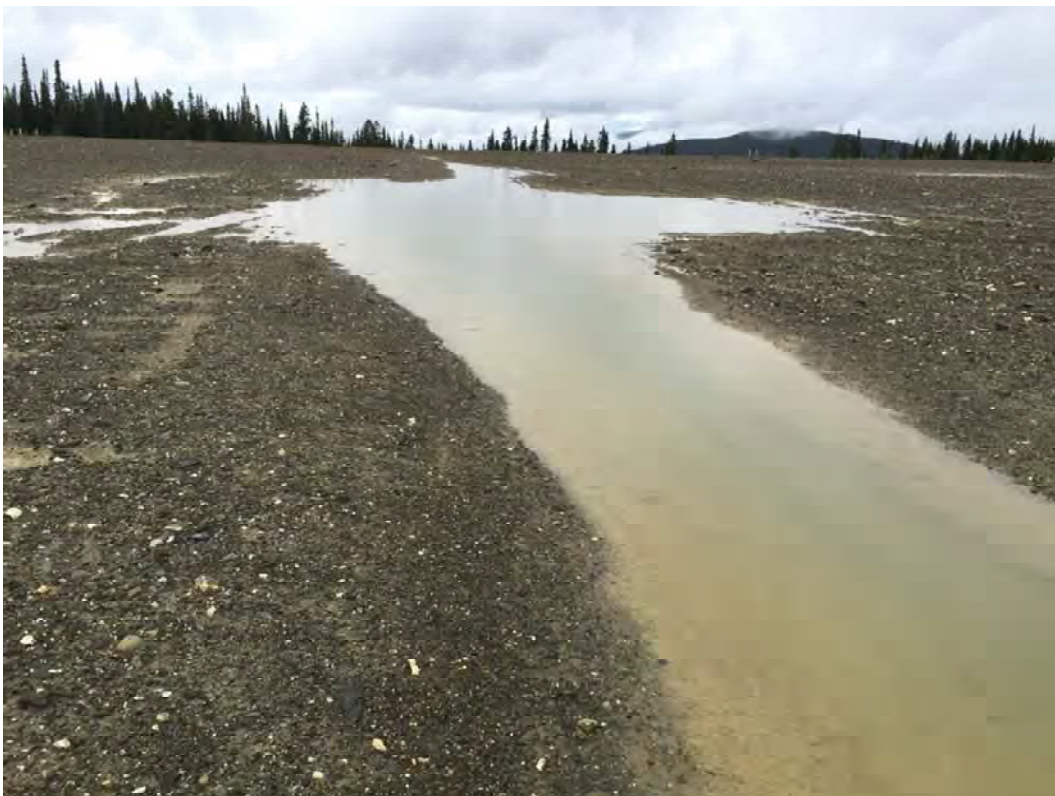
Photo 6: Ponding in the Central Drainage Channel within the Till Cover
