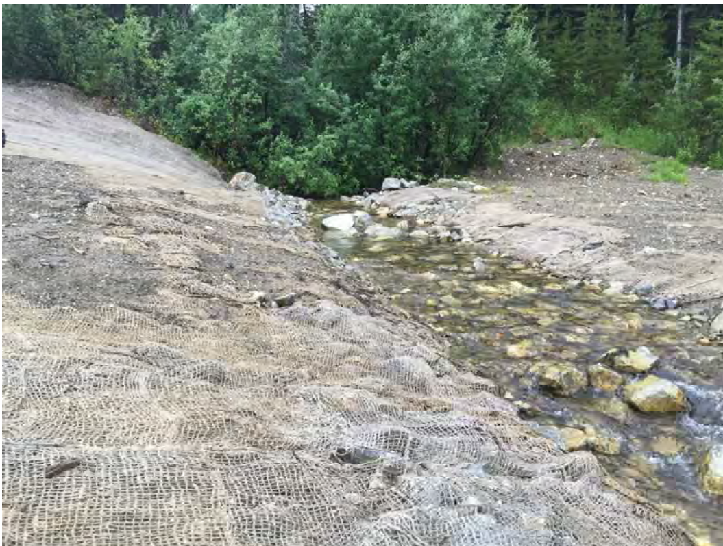
Photo 10: Riprapped Channel at the Second Crossing of North Creek s
