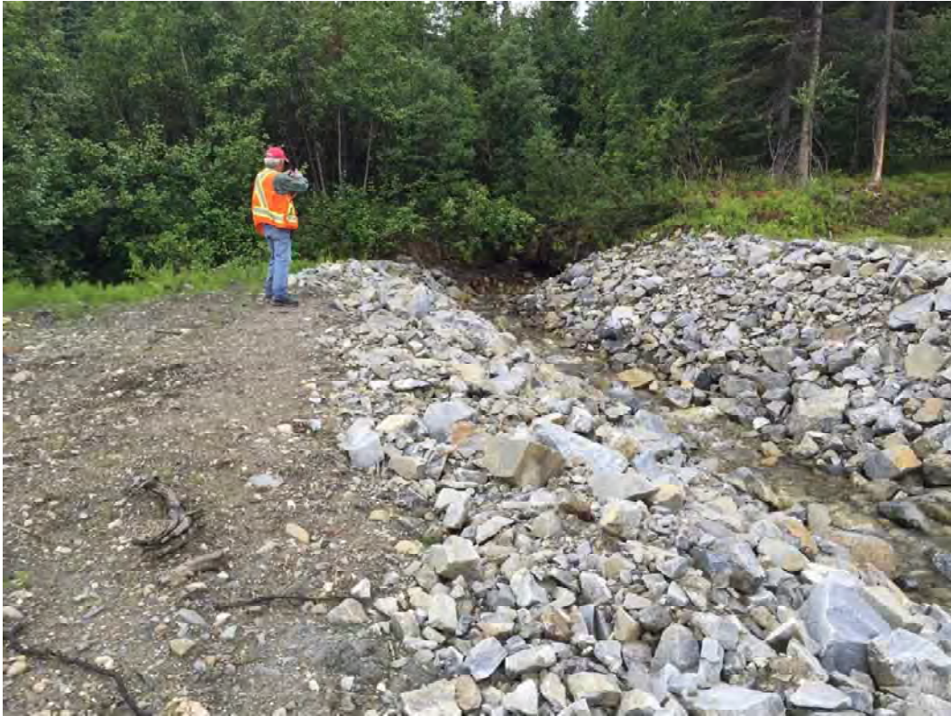
Photo 19: Inlet of Camp Creek into the Camp Creek drainage channel
