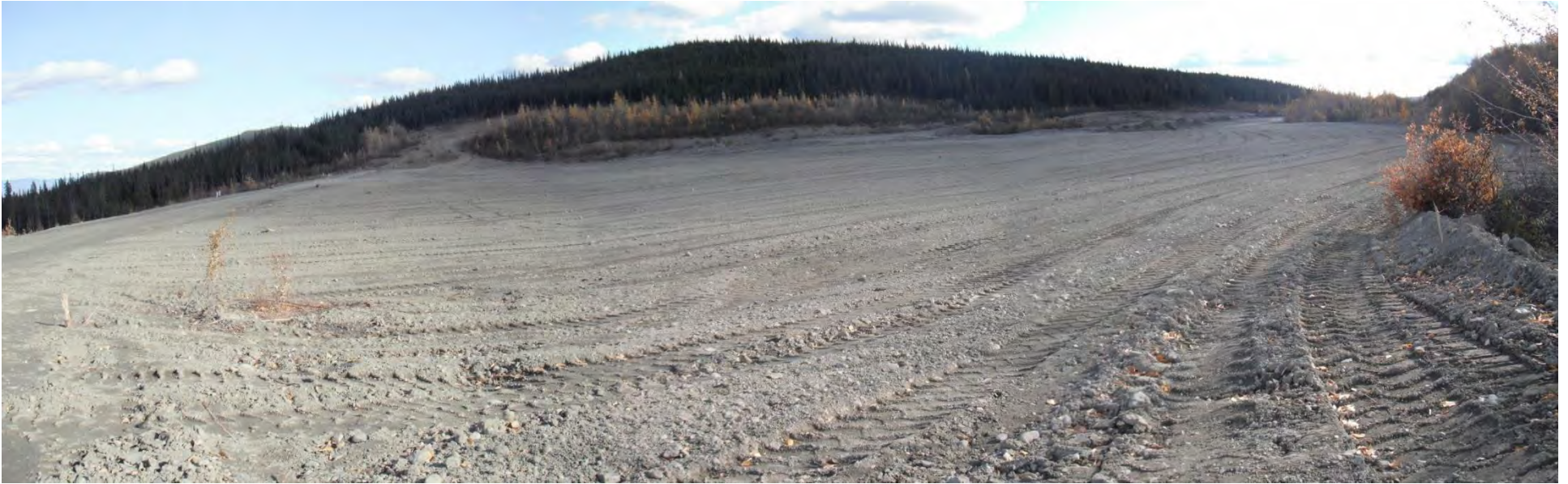
Photo #111: Capped tailings on North Pond, September 2014.
