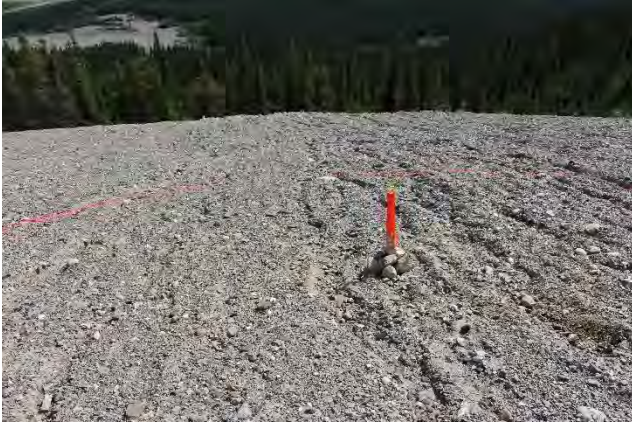
Photo #13: 2016, looking downslope
