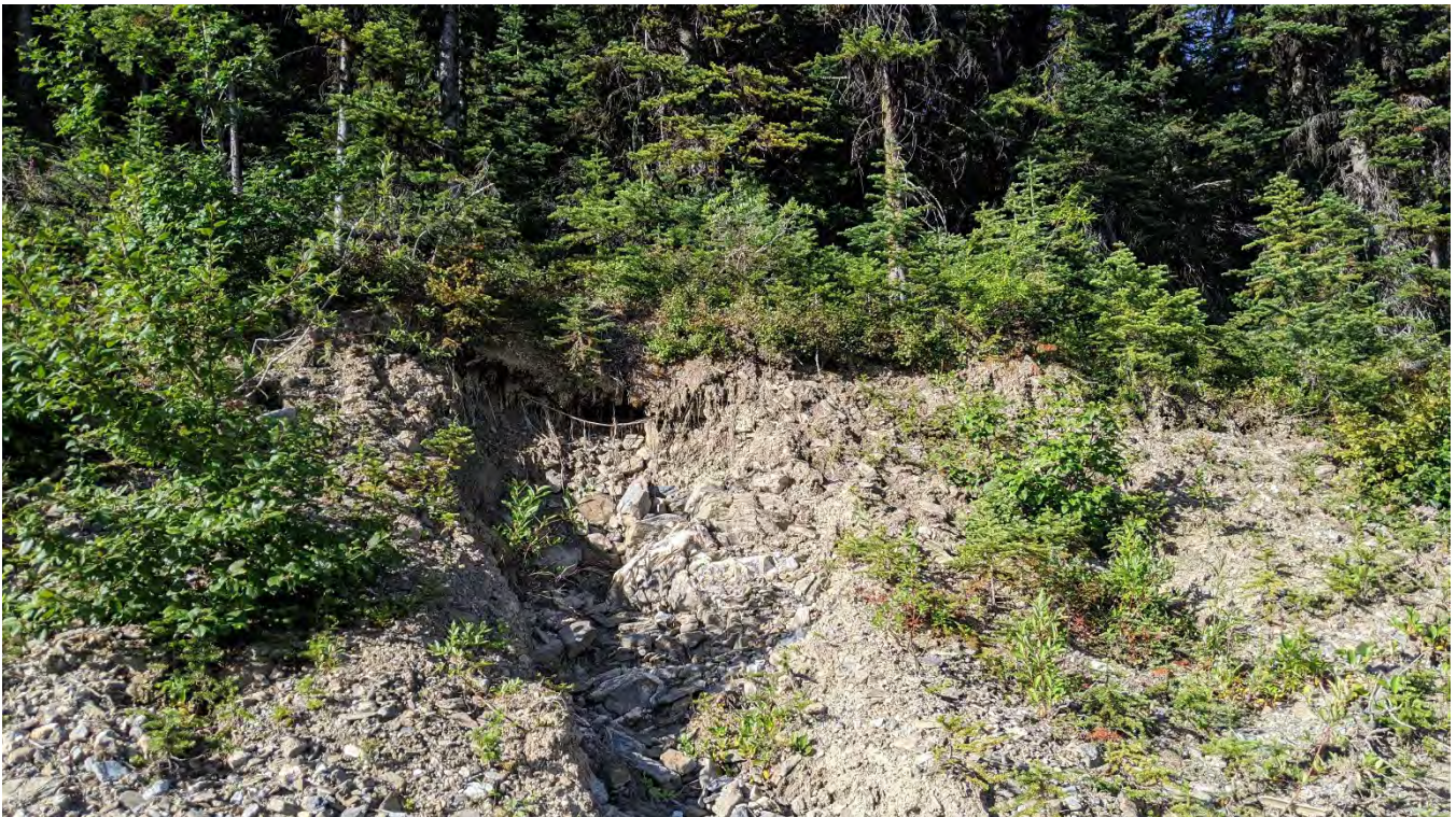
Photo WR-02: Erosion gully across the decommissioned access road to the Jewelbox Waste Rock Dump.
