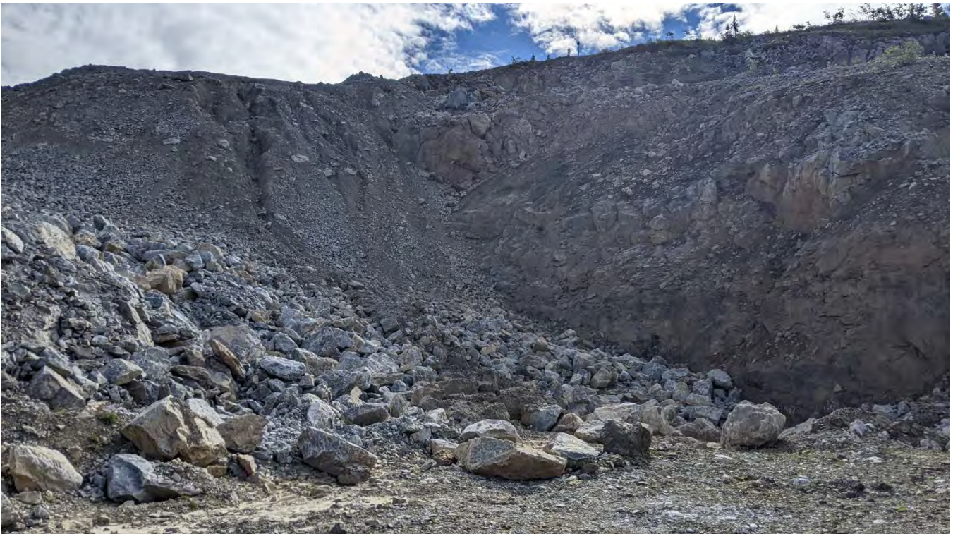
Photo WR-16: Backfill at the 1380 Portal below Main Zone Waste Rock Dump.
