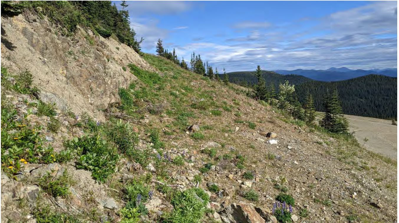
Photo WR-11: Fill placement above the 1408 Portal looking north.
