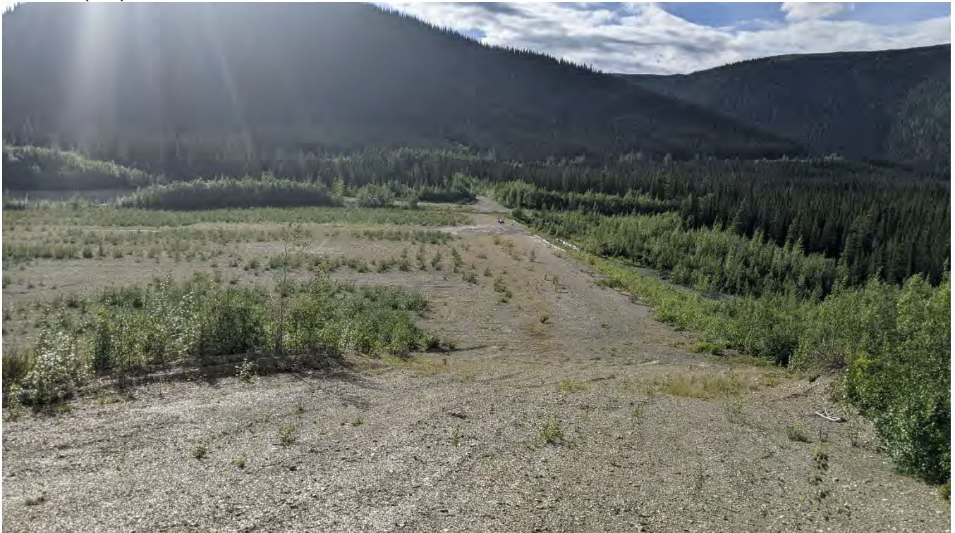
Photo ND-04: North Dam looking west.
