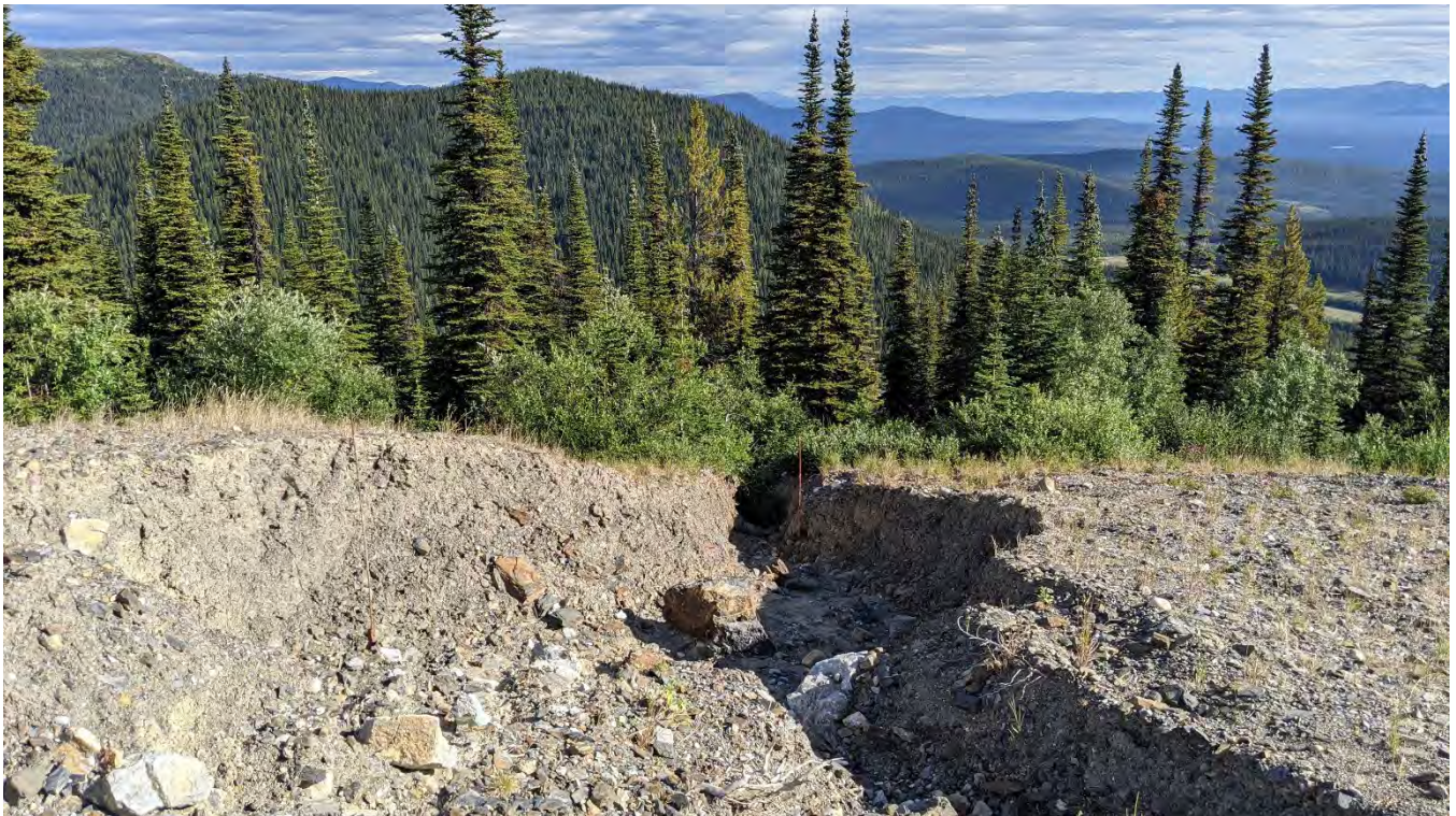
Photo WR-04: Erosion gully at the base of the Jewelbox Waste Rock Dump looking downslope. The gully has eroded down to bedrock.
