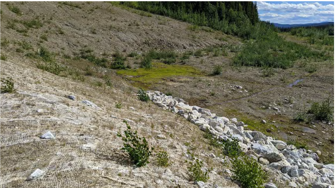
Photo SRS-06: Downstream face of the SRS on the east side of the spillway looking southeast.
