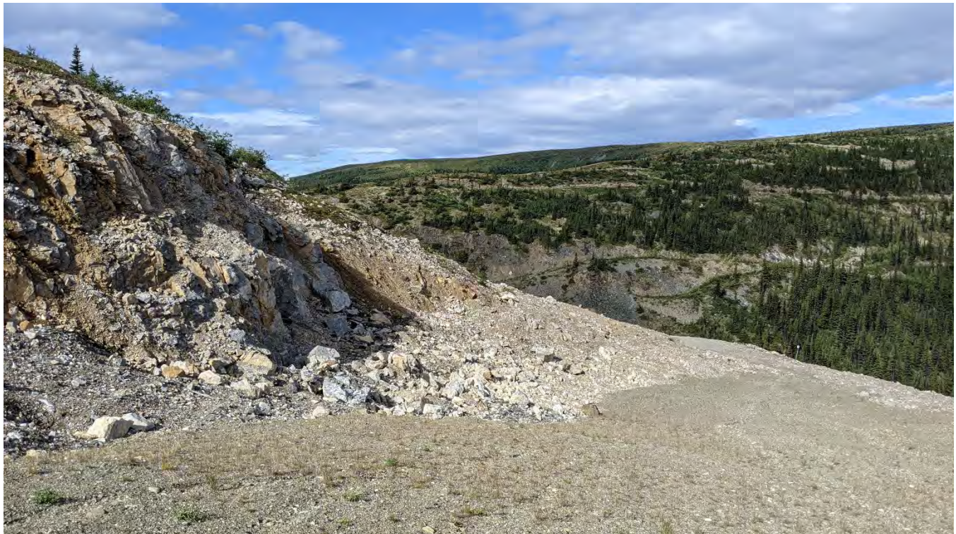
Photo WR-14: Jewelbox Pit wall looking west.
