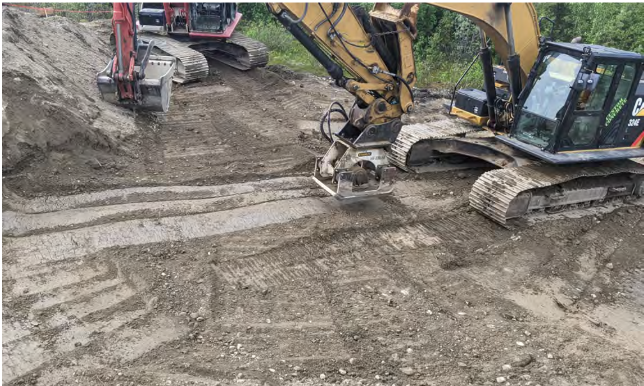
Photo 8: Compaction of Sand and Gravel in 0.3 m lifts (June 24, 2022).
