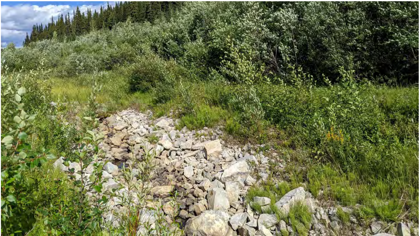
Photo DC-04: North Diversion Channel looking upstream.
