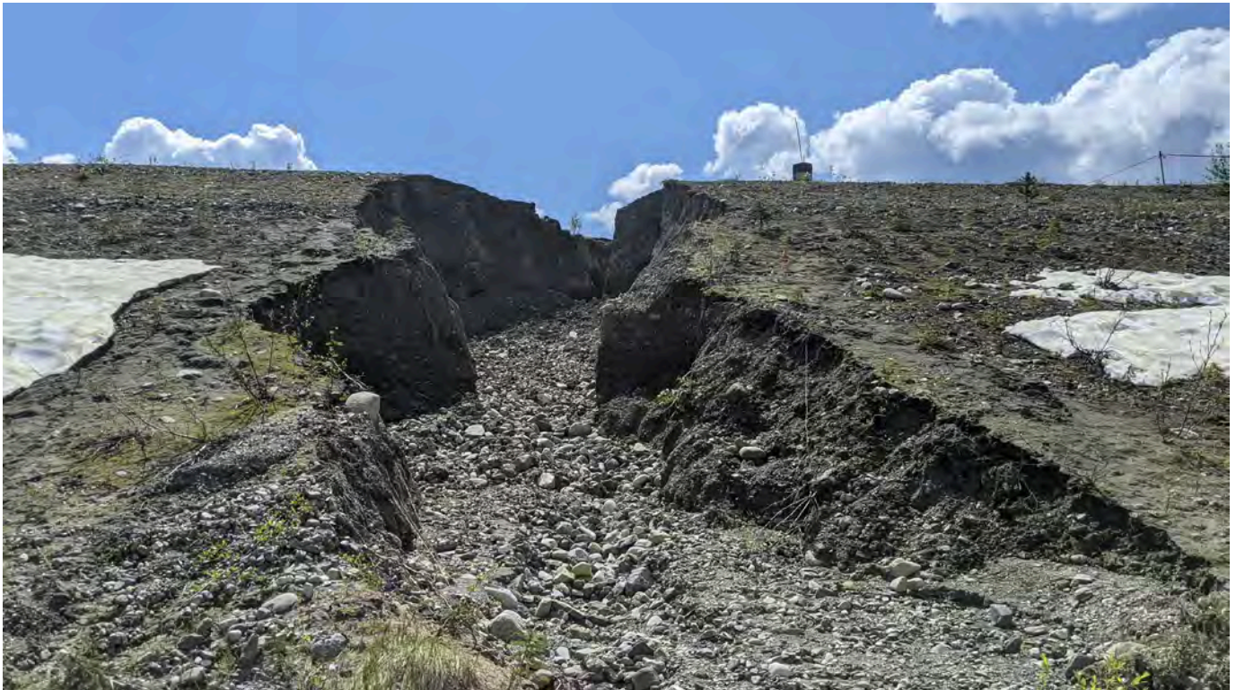
Photo 2: Erosion Gully looking upslope (June 21, 2022).
