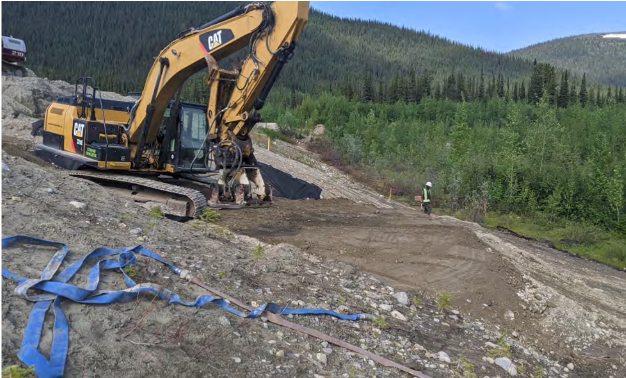
Photo 9: Till placement (June 26, 2022).
