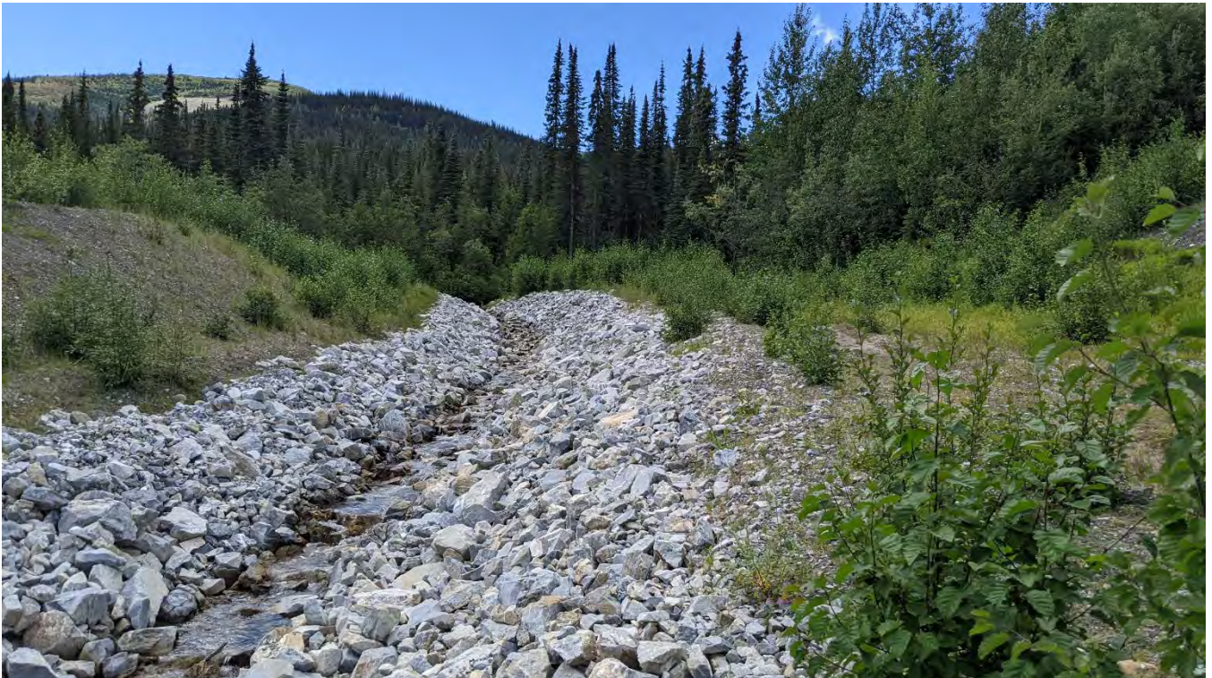
Photo DC-02: Camp Creek looking upstream.
