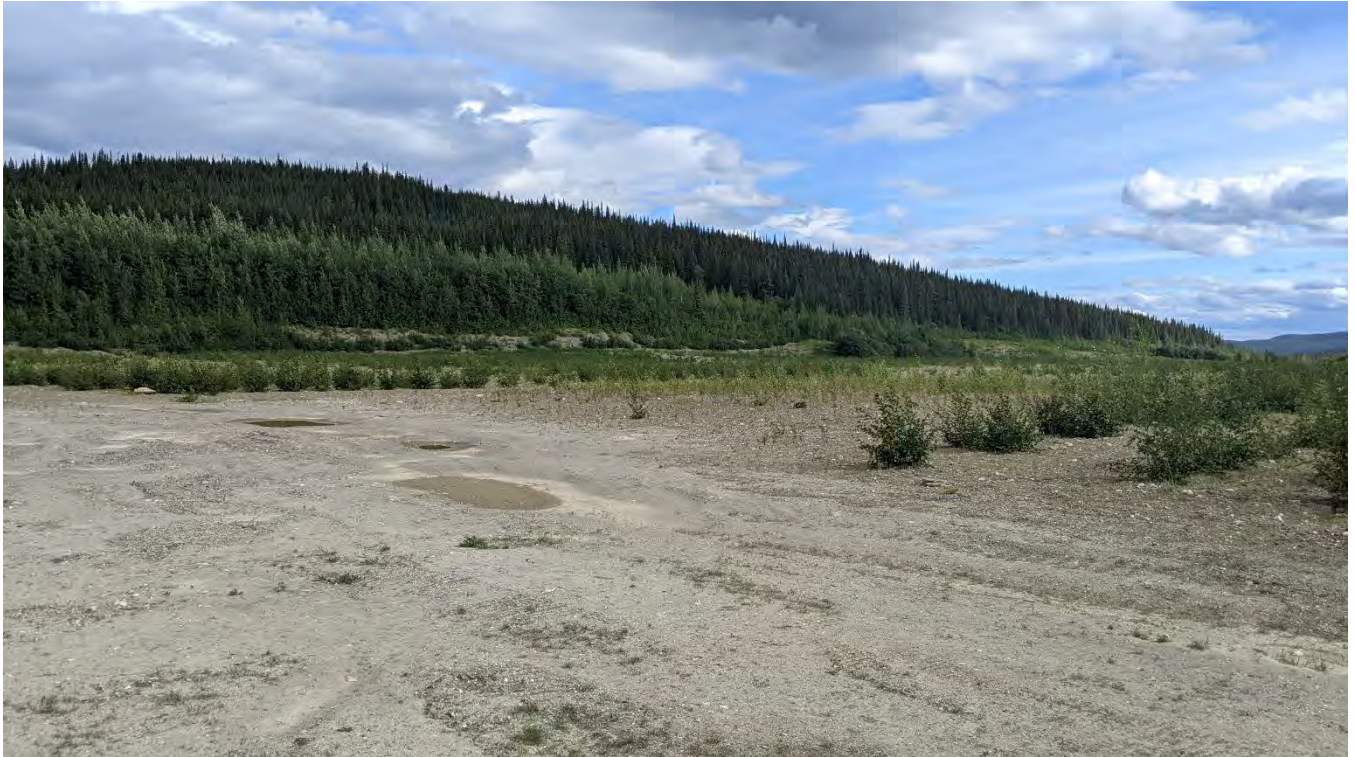
Photo TC-01: North Dam crest and tailings cover south of the erosion gully repair area.
