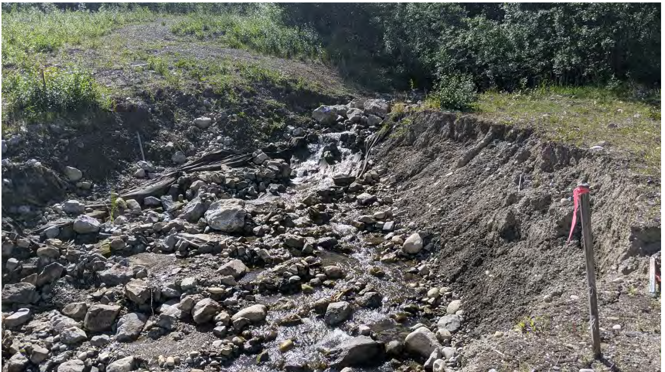
Photo NC-06: On-going channel and bank erosion at the upstream end of the lower decommissioned access road crossing of North Creek to the landfill area.
