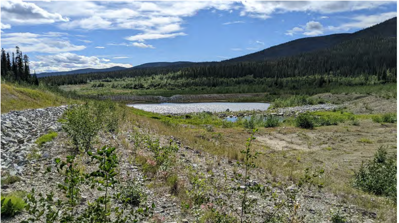
Photo SRS-01: SRS and pond looking south. The North Drainage Channel is located at the left side of the photo.
