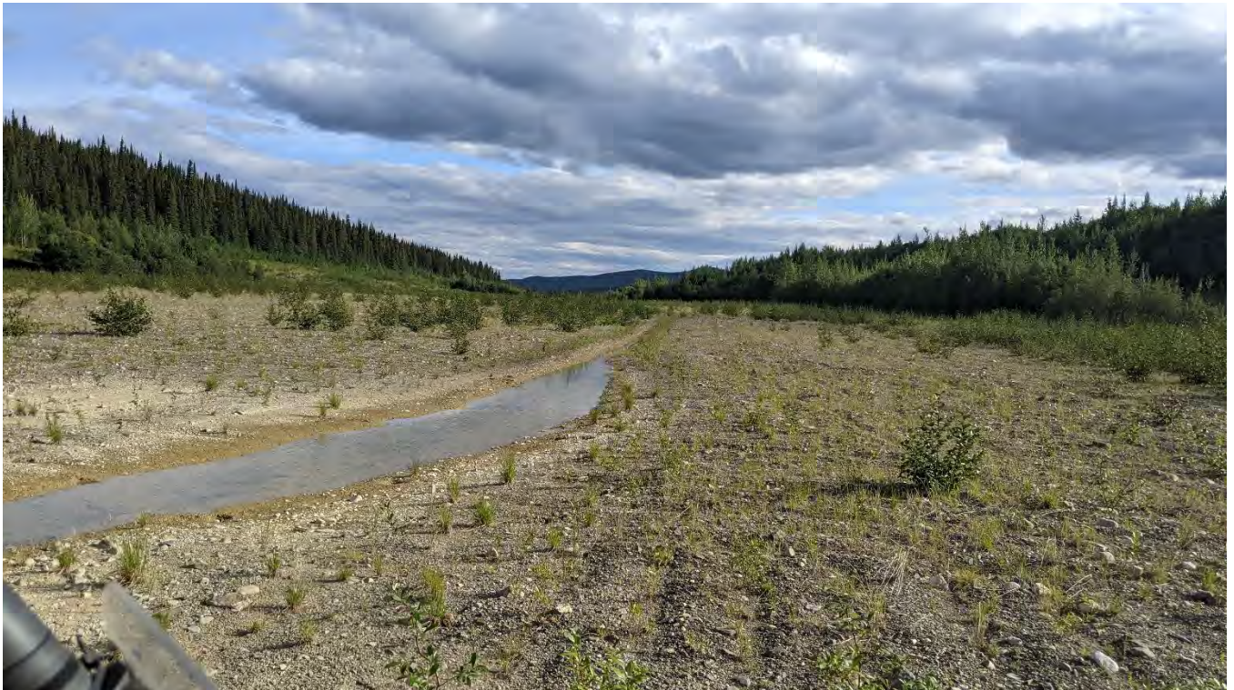
Photo TC-03: Main drainage swale that flows south through the middle of the tailings cover.
