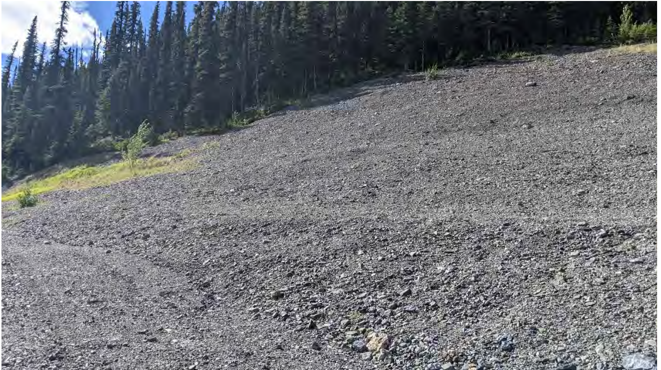
Photo WR-17: Regraded Burnick Waste Rock Dump at the 1200 Portal.
