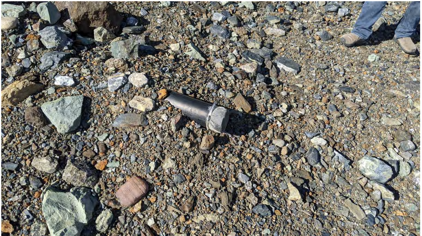
Photo WR-20: 1300 Portal drainpipe.
