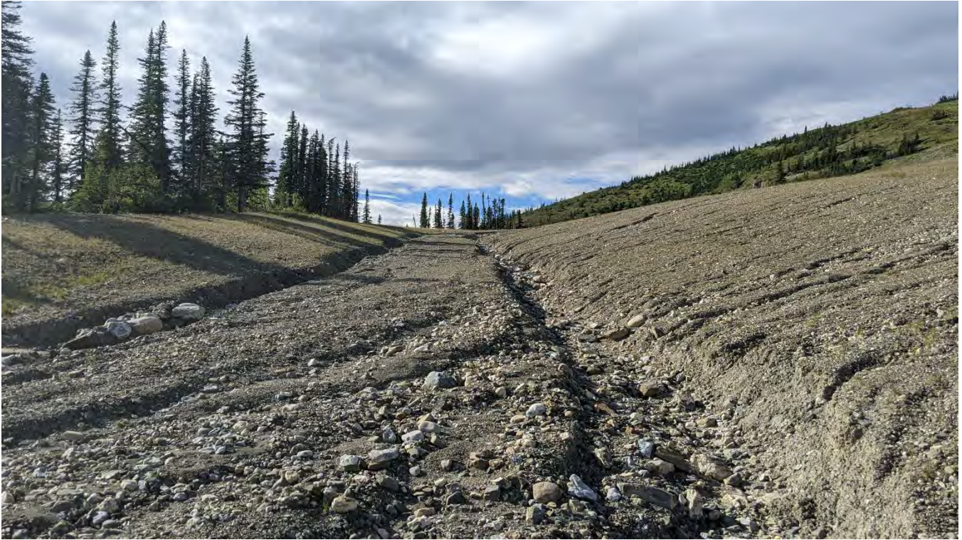
Photo WR-05: Erosion gully at the base of the Jewelbox Waste Dump looking upstream.
