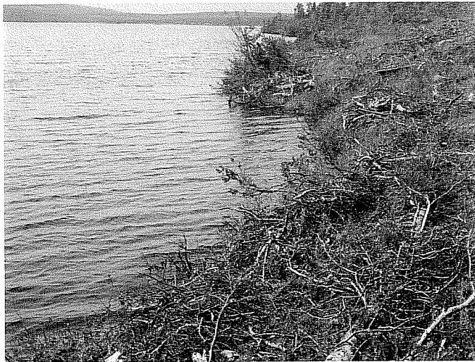
Photo7: Vegetative sediment berm
