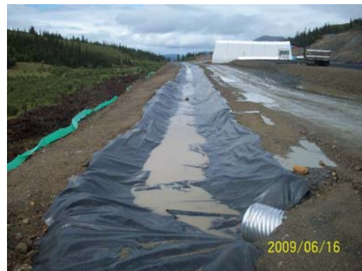
Photo 12: Looking NW at the alignment along Collection Ditch 3.
