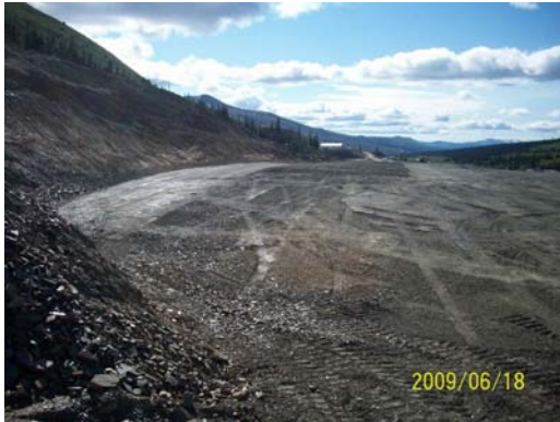
Photo 3: Looking SE at cut slope for Fuel Storage and Generator Pads.
