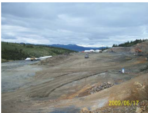
Photo 1: Looking W at excavation and fill placement at the Mill Site.
