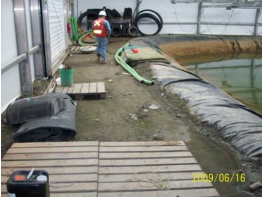
Photo 5: Looking NE from the western corner of Sump 1. Notice the settlement along the perimeter.
