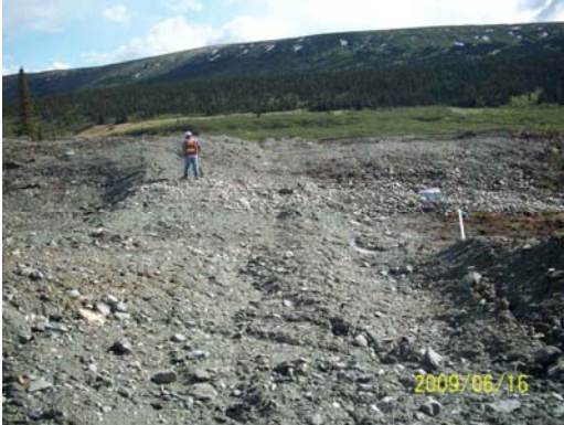
Photo 27: Looking SE at the buried CSP culvert alignment of Ditch A.
