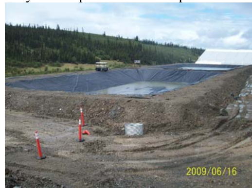
Photo 10: Looking west at Sumps 4 and 5. Sump 5 is empty.
