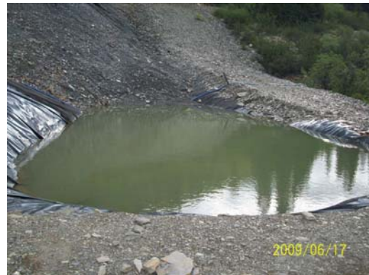
Photo 20: Looking east at the runoff collection sump for the waste rock end of the stockpile area.
