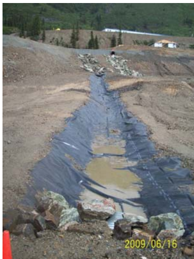
Photo 11: Looking East at the lower portion of Collection Ditch 2.
