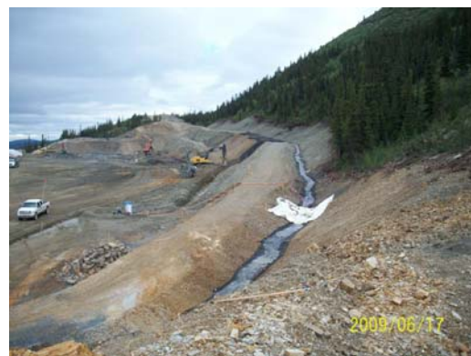
Photo 2: Looking NW at excavator repairing downslope of Ditch 1.
