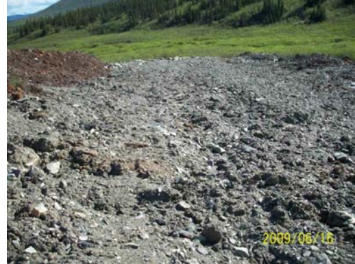
Photo 28: Looking south at the buried CSP culvert alignment of Ditch B.
