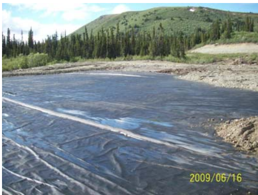
Photo 21: Looking north at the LTF.
