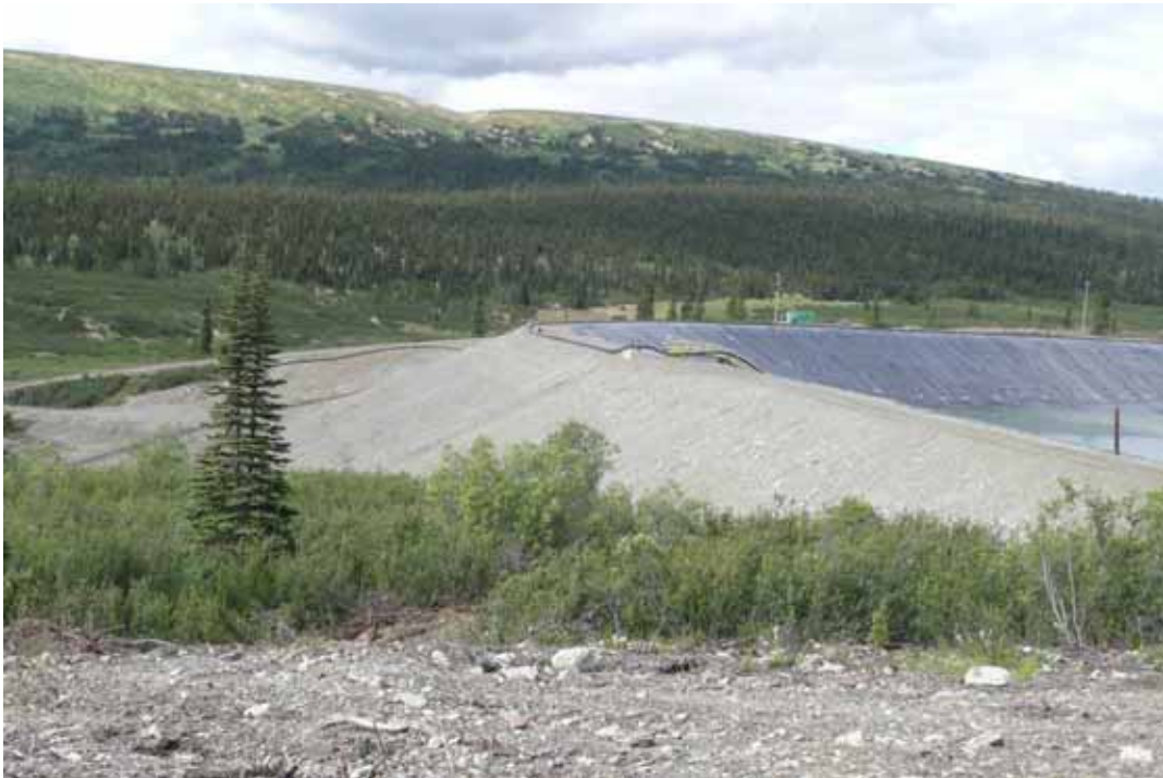
Photo 41 View of downstream slope of dam, from the left abutment
