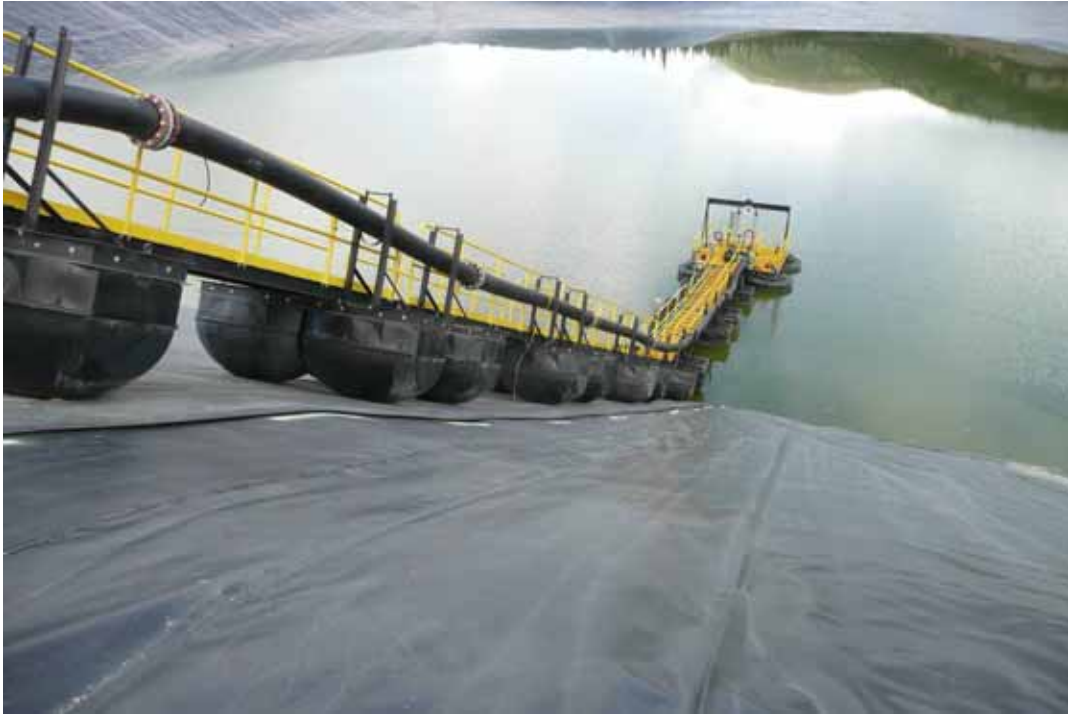
Photo 22 Access ramp to pump barge – note protective liner layer
