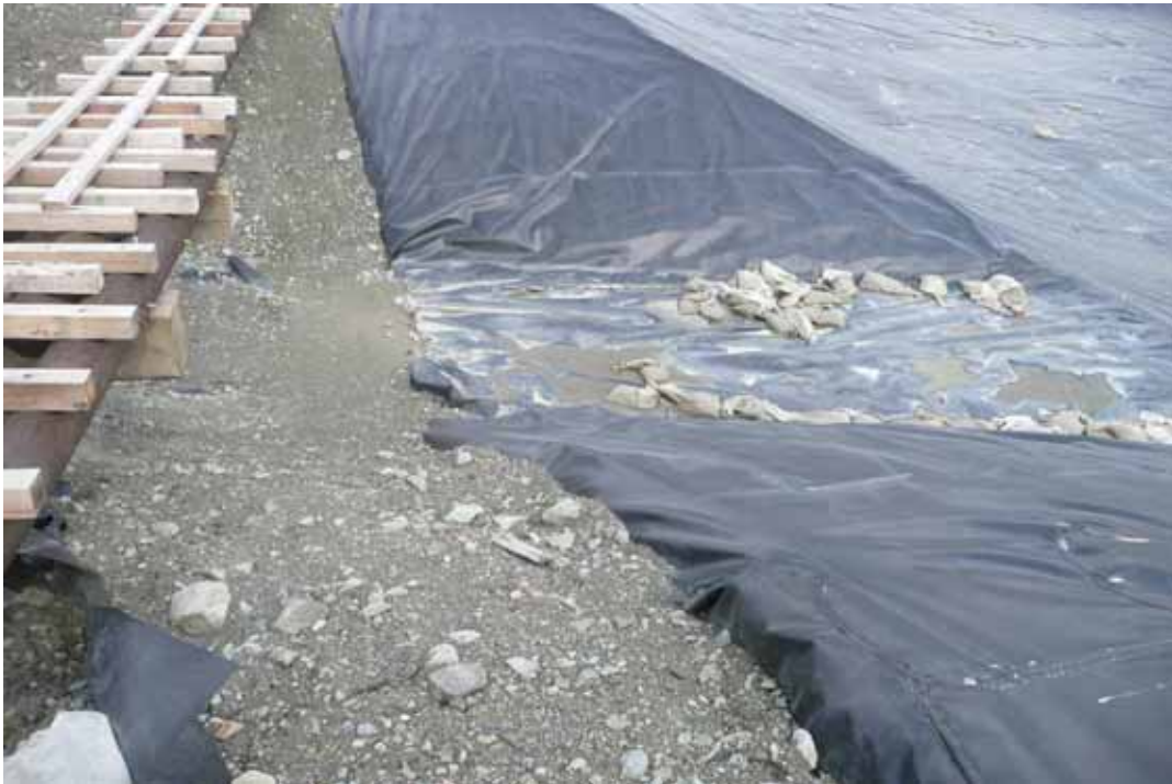
Photo 35 Emergency spillway inlet – note pipeline bridge across spillway
