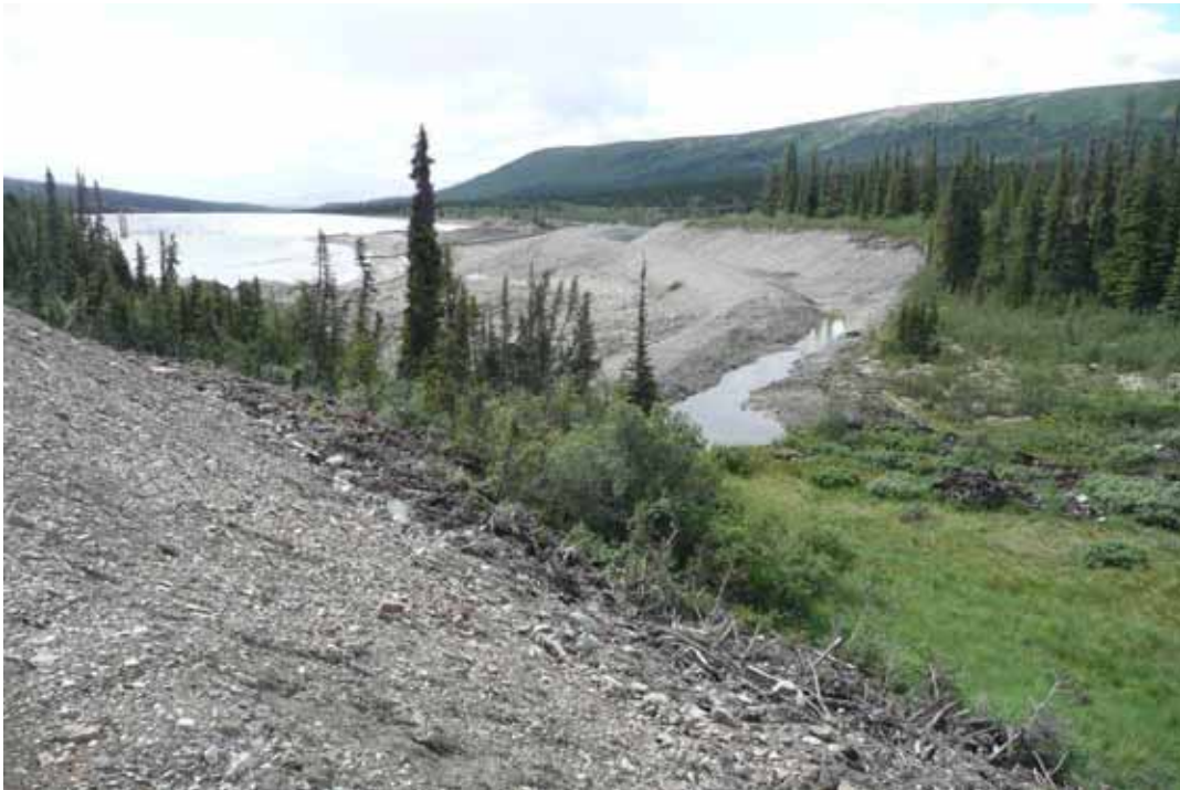
Photo 37 View of Ditch A from upstream end of impoundment
