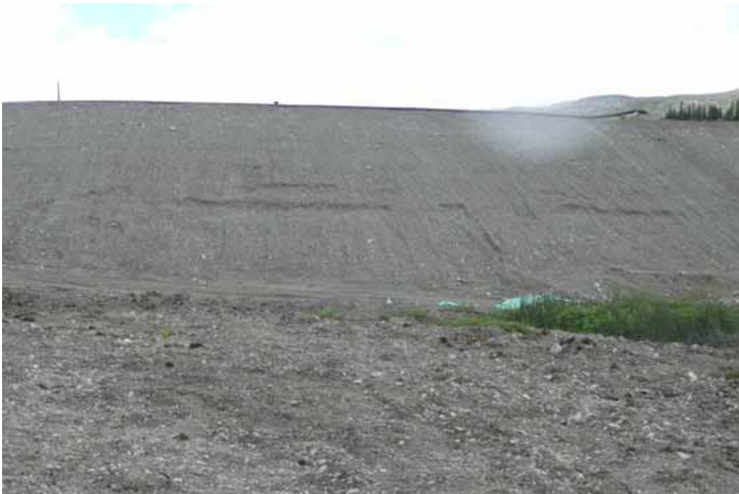
Photo 27 View of downstream slope of dam – note darker layers
