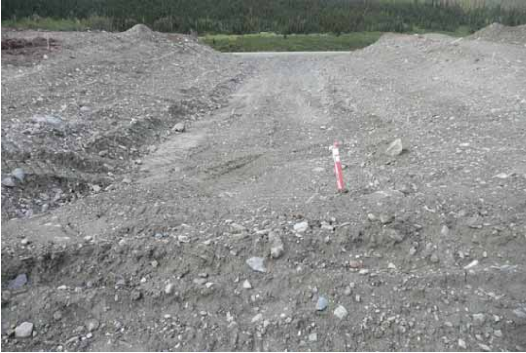
Photo 36 Emergency spillway outlet towards road area
