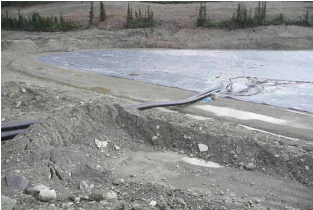
Photo 5 View from west side of impoundment, looking north
