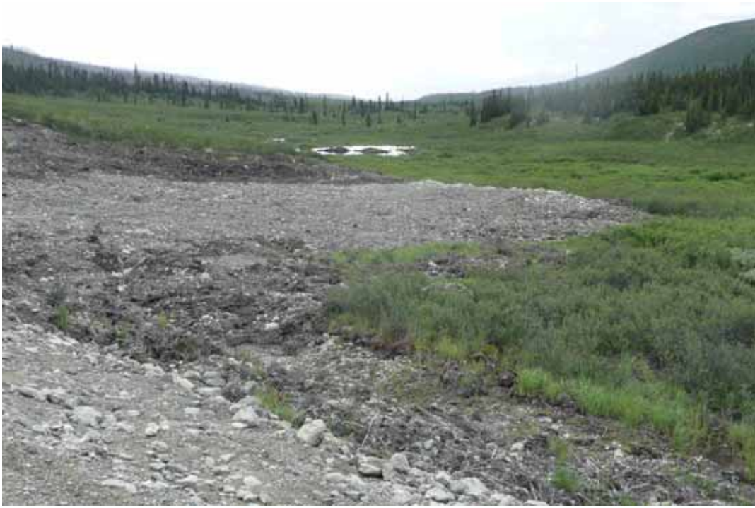
Photo 32 Outlet from Ditch B culvert
