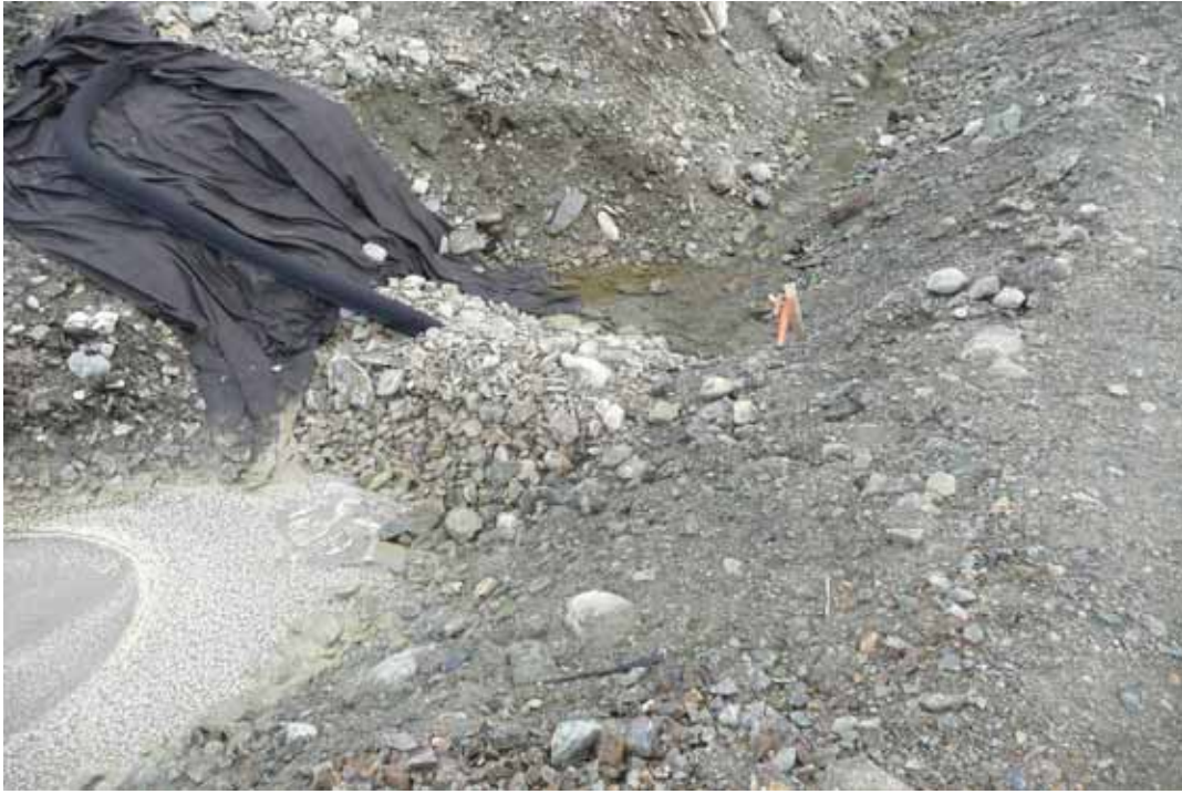
Photo 8 Inlet to the underdrains at the upstream end of the impoundment
