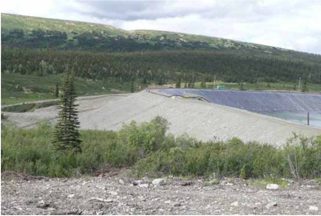
Photo 40 View of dam from left abutment
