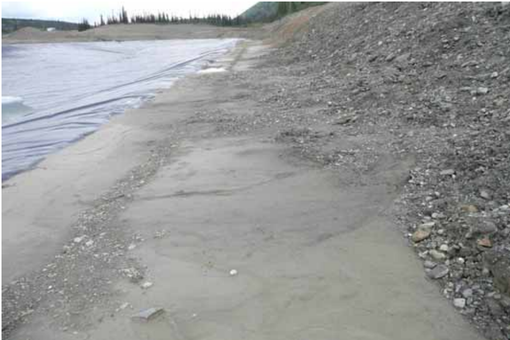
Photo 13 View of perimeter road on the east side of the impoundment
