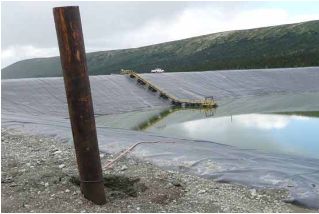
Photo 14 View of main dam and reclaim barge looking southwest
