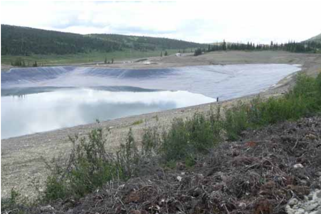
Photo 20 Impoundment – view from left abutment
