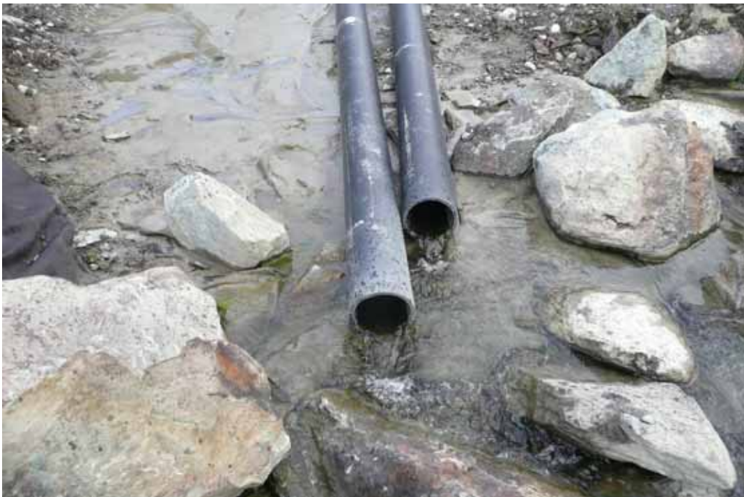
Photo 25 Underdrain pipes at toe of the dam – flow approximately 10 L/s
