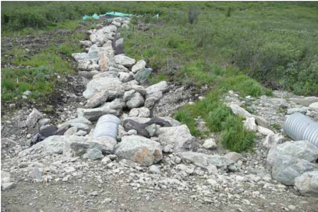
Photo 30 Seepage dam spillway culvert outlet
