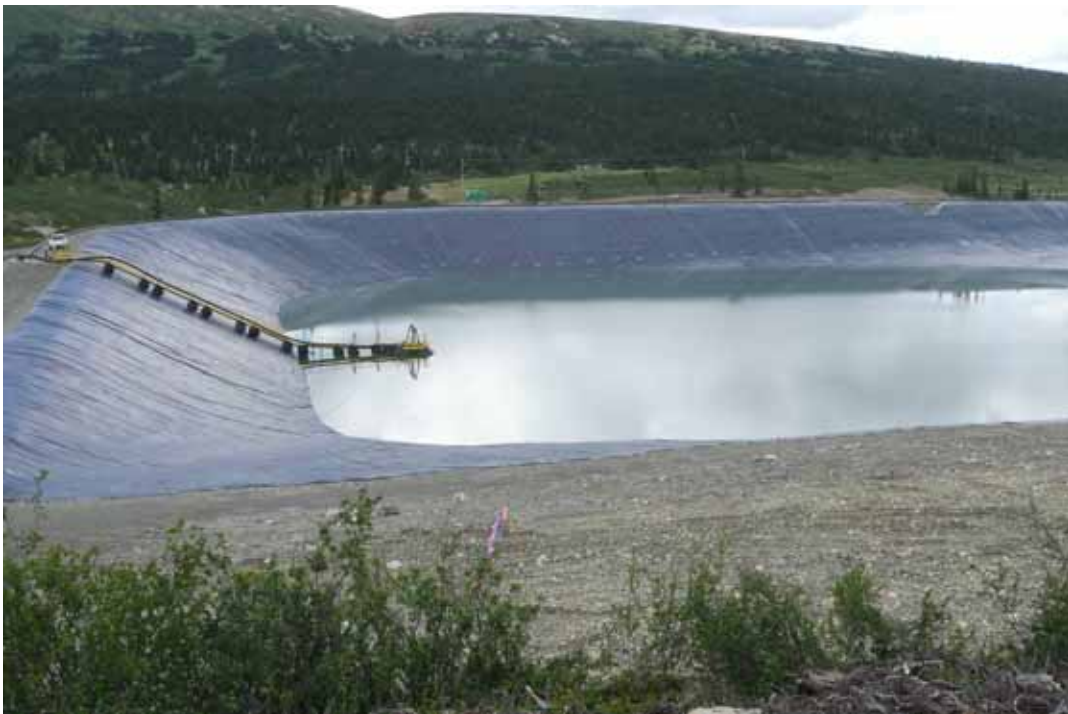
Photo 21 Impoundment – view from left abutment
