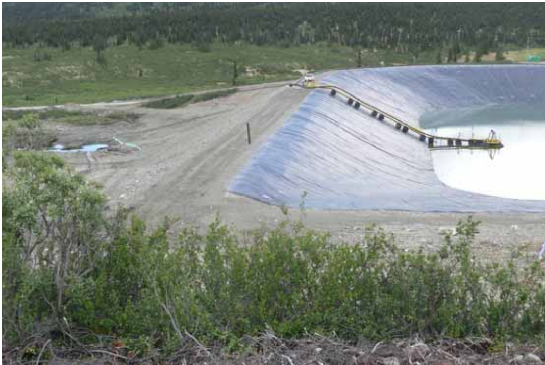
Photo 19 Main dam – view from left abutment
