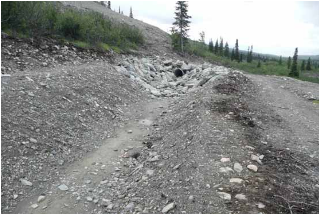
Photo 18 Ditch B – outlet to culvert
