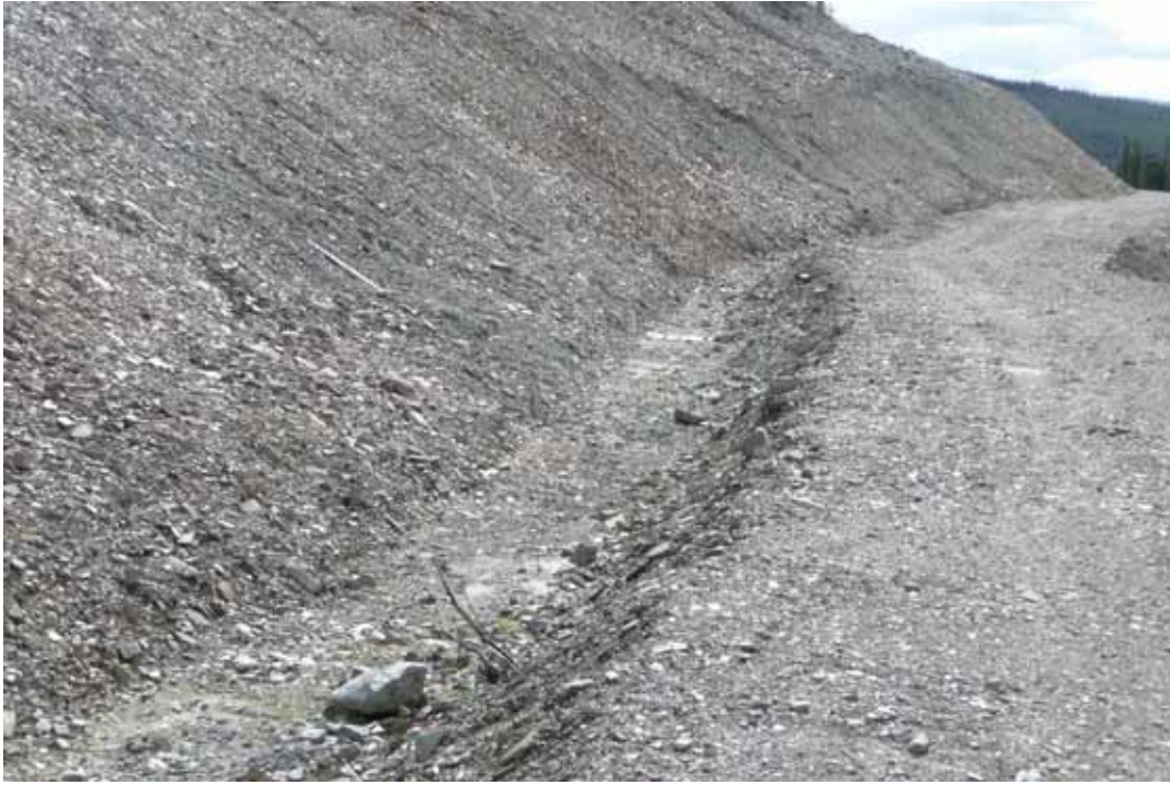
Photo 38 View of Ditch B
