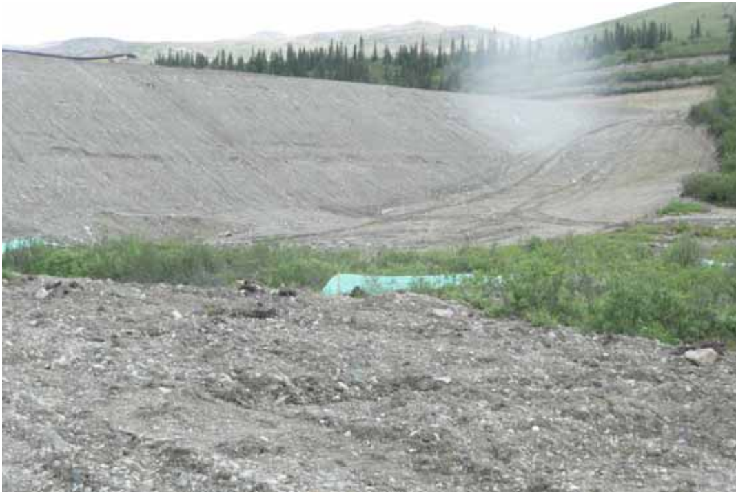
Photo 28 View of downstream slope of dam
