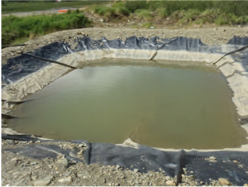
Photo 20 Looking at the LTF sump. (July 10, 2012)
