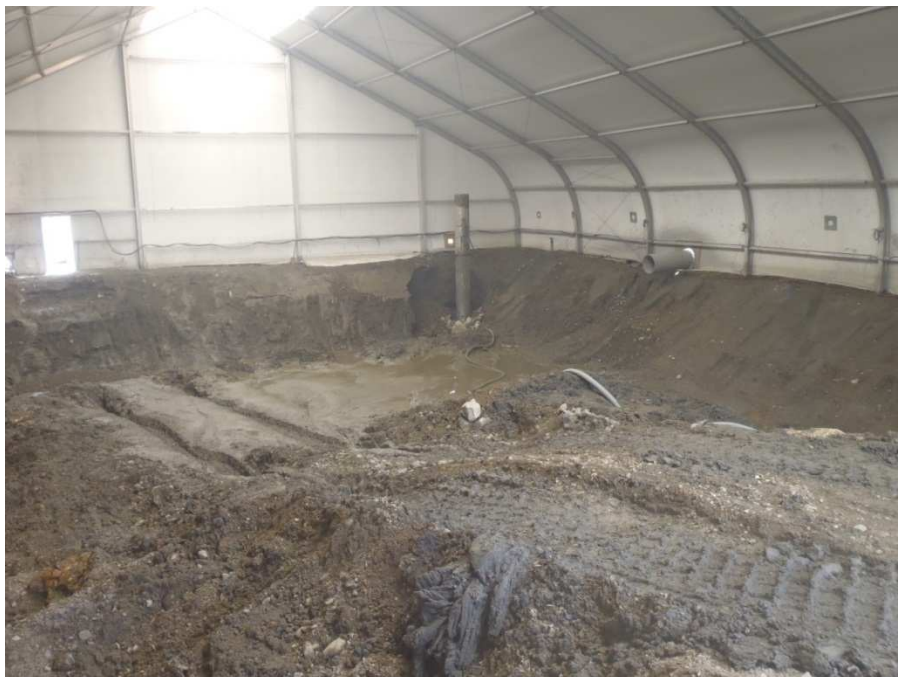
Photo 7 Sump 2 being reconstructed. (July 9, 2013)
