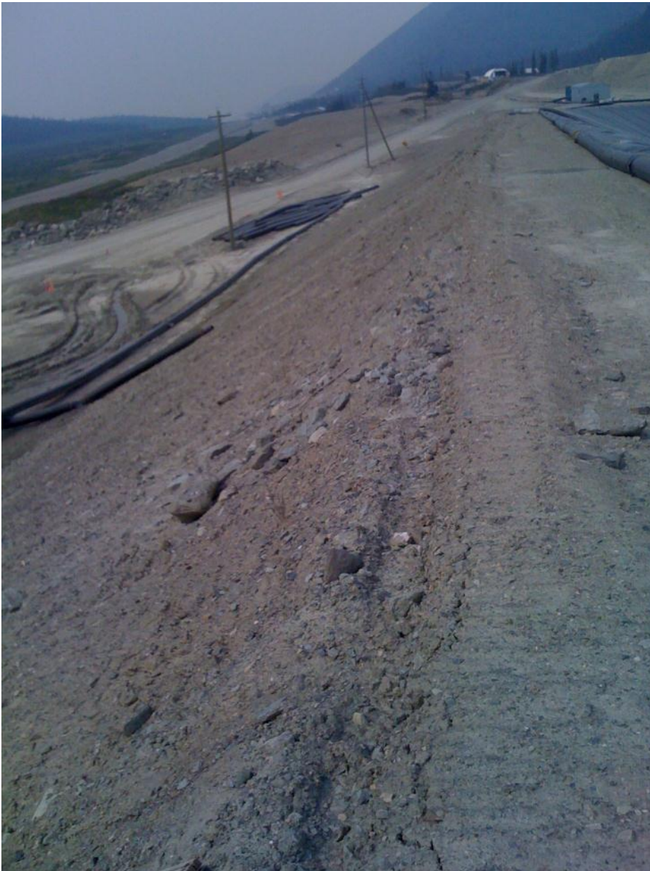
Photo 11 View of west dam downstream face, looking north
