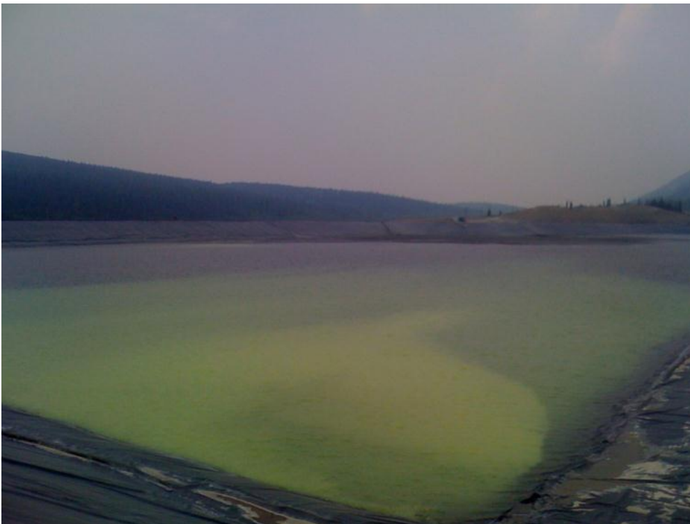
Photo 7 Impoundment from east abutment looking north
