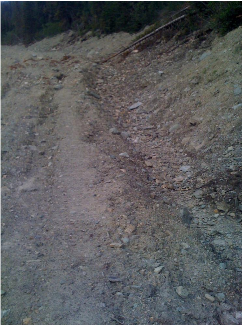
Photo 32 Waste Rock Stockpile – Diversion Ditch
