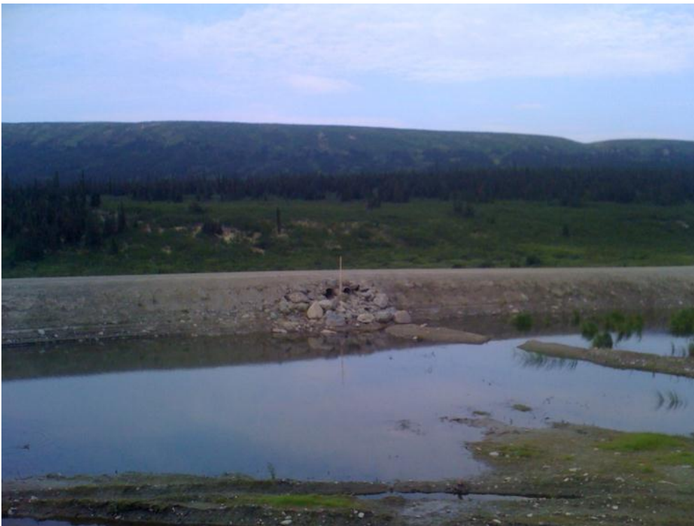
Photo 30 Seepage dam spillway culvert inlets
