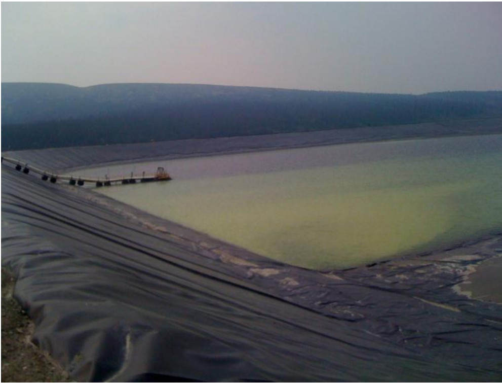
Photo 4 Dam upstream face
