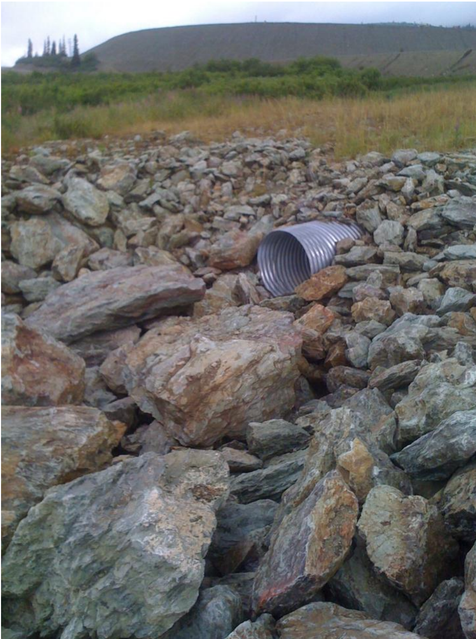
Photo 24 Outlet from Ditch B culvert
