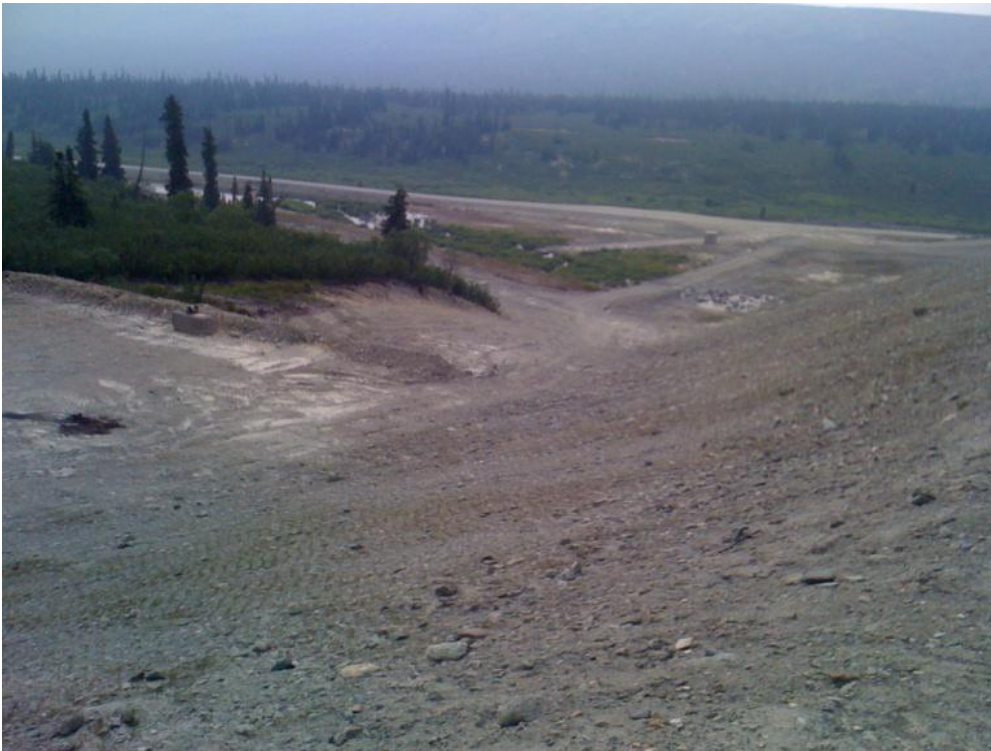
Photo 27 Seepage pond area from Tailings Dam
