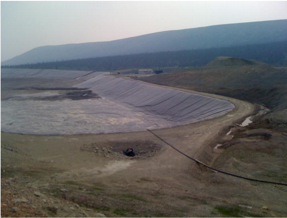
Photo 25 Inlet to the underdrain – flow from upstream
