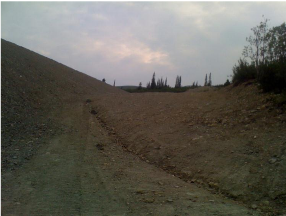
Photo 17 Seepage collection ditch at downstream toe of dam (no flow)
