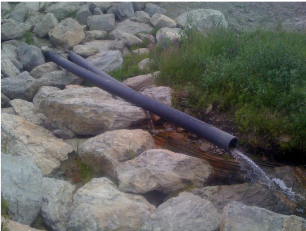
Photo 26 Underdrain Outlet – flow to Go Creek
