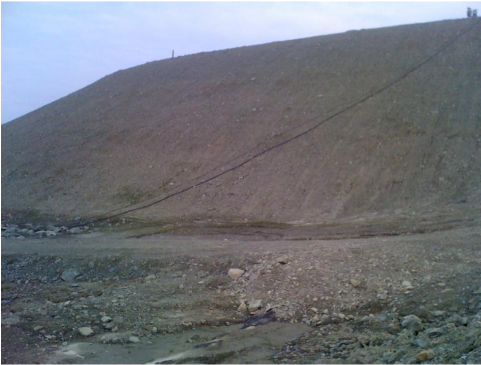
Photo 18 Downstream dam face
