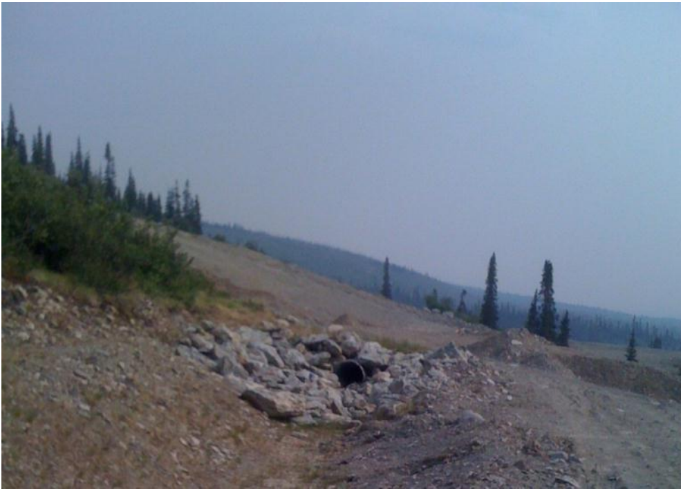
Photo 23 Ditch B – culvert inlet
