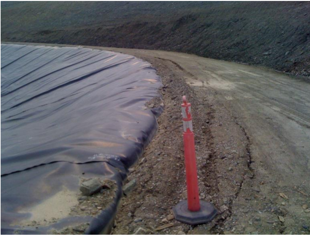
Photo 16 Cracks at North End of impoundment
