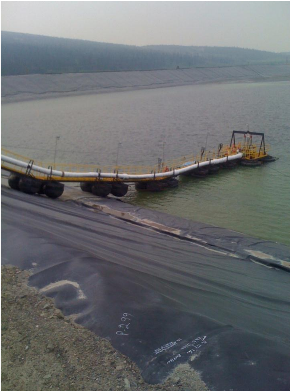
Photo 10 Reclaim pump barge
