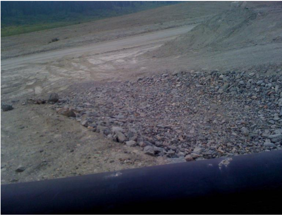
Photo 13 Stage 2 spillway channel, from dam crest
