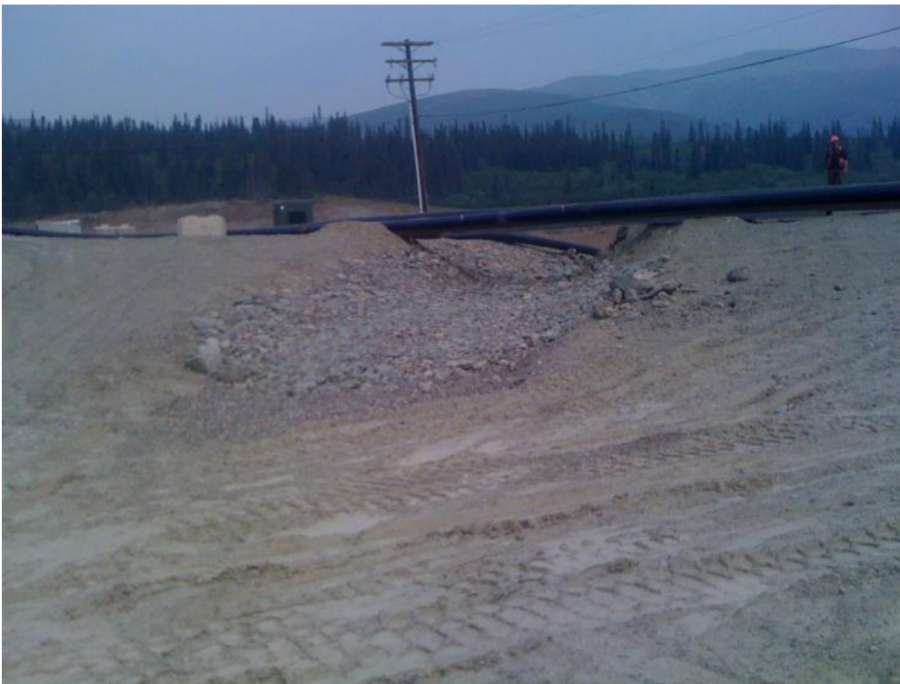
Photo 14 Stage 2 spillway channel, from Mine Haul Road
