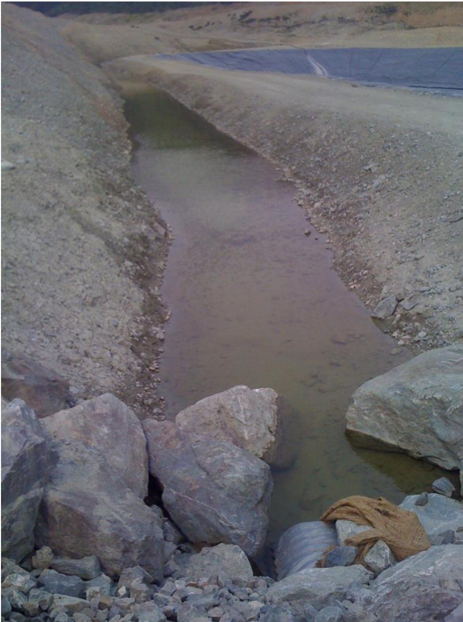
Photo 20 View of Ditch A from culvert inlet
