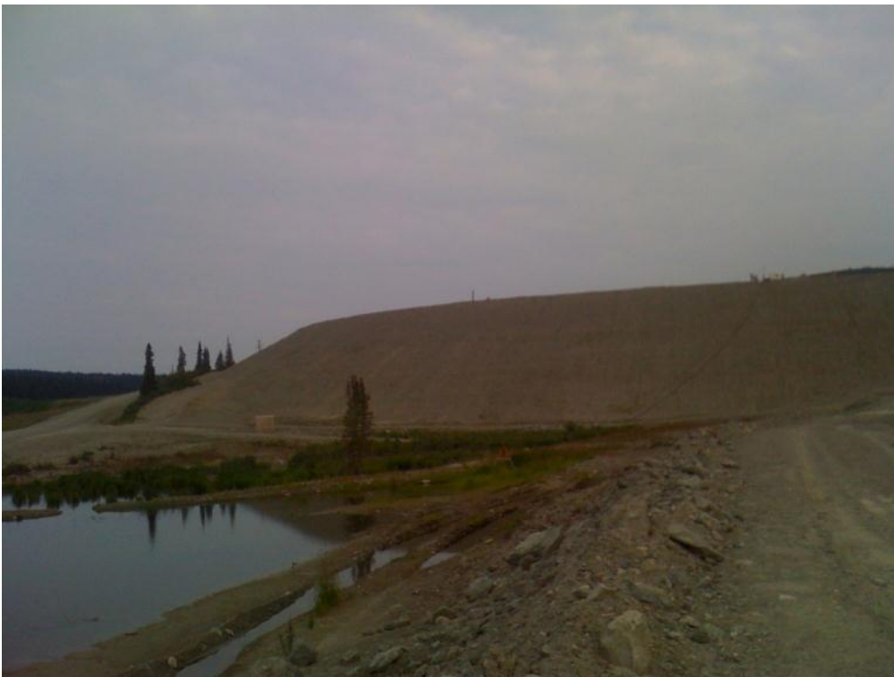
Photo 19 South downstream dam face
