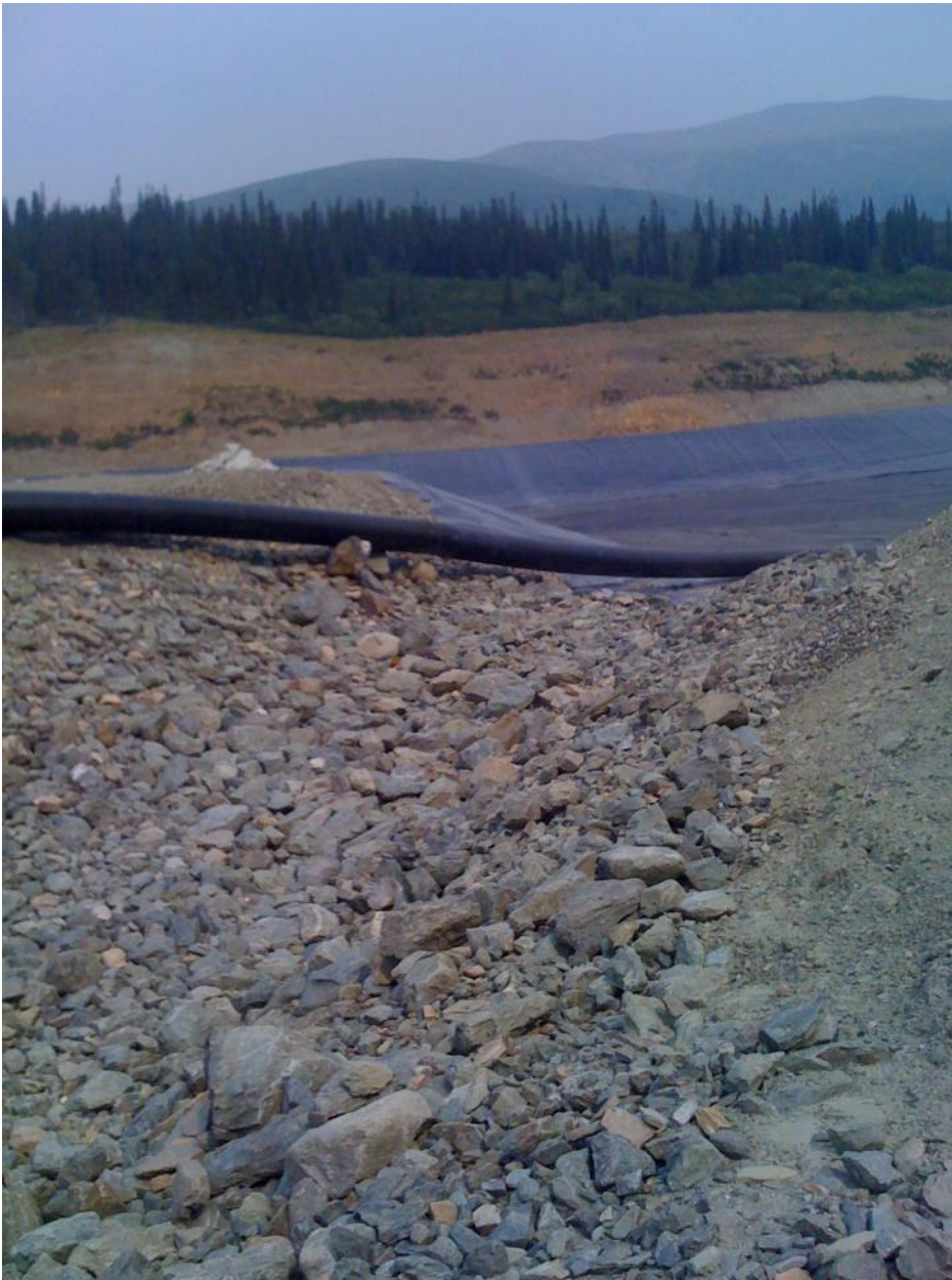
Photo 12 Stage 2 spillway at dam crest
