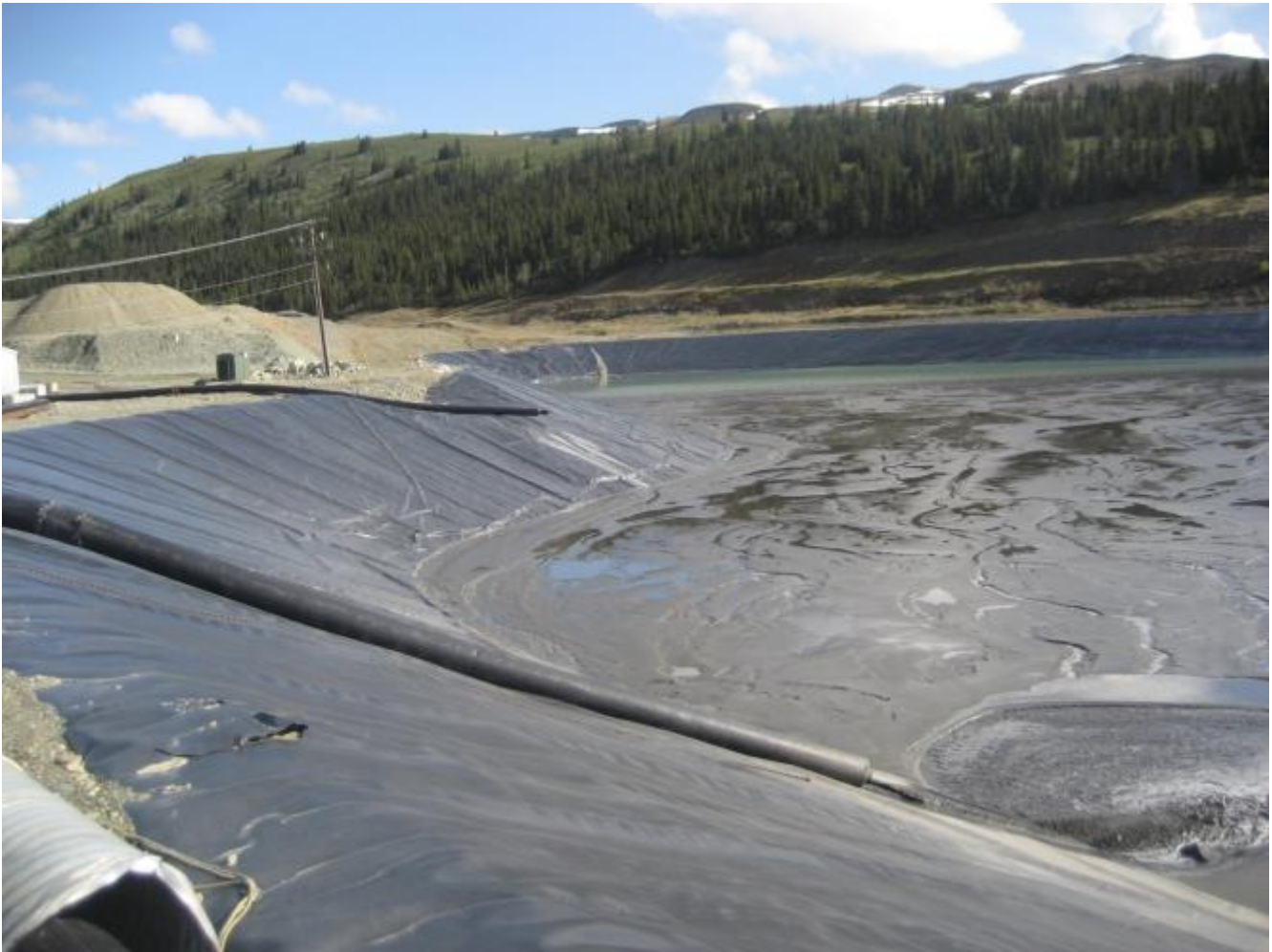
Photo 4 View from west side of impoundment, looking north
