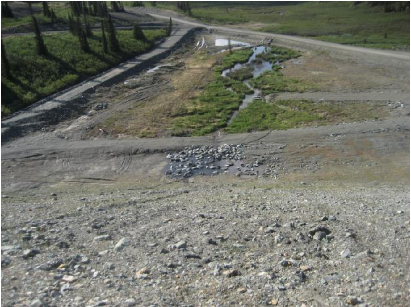
Photo 28 Seepage Collection Basin
