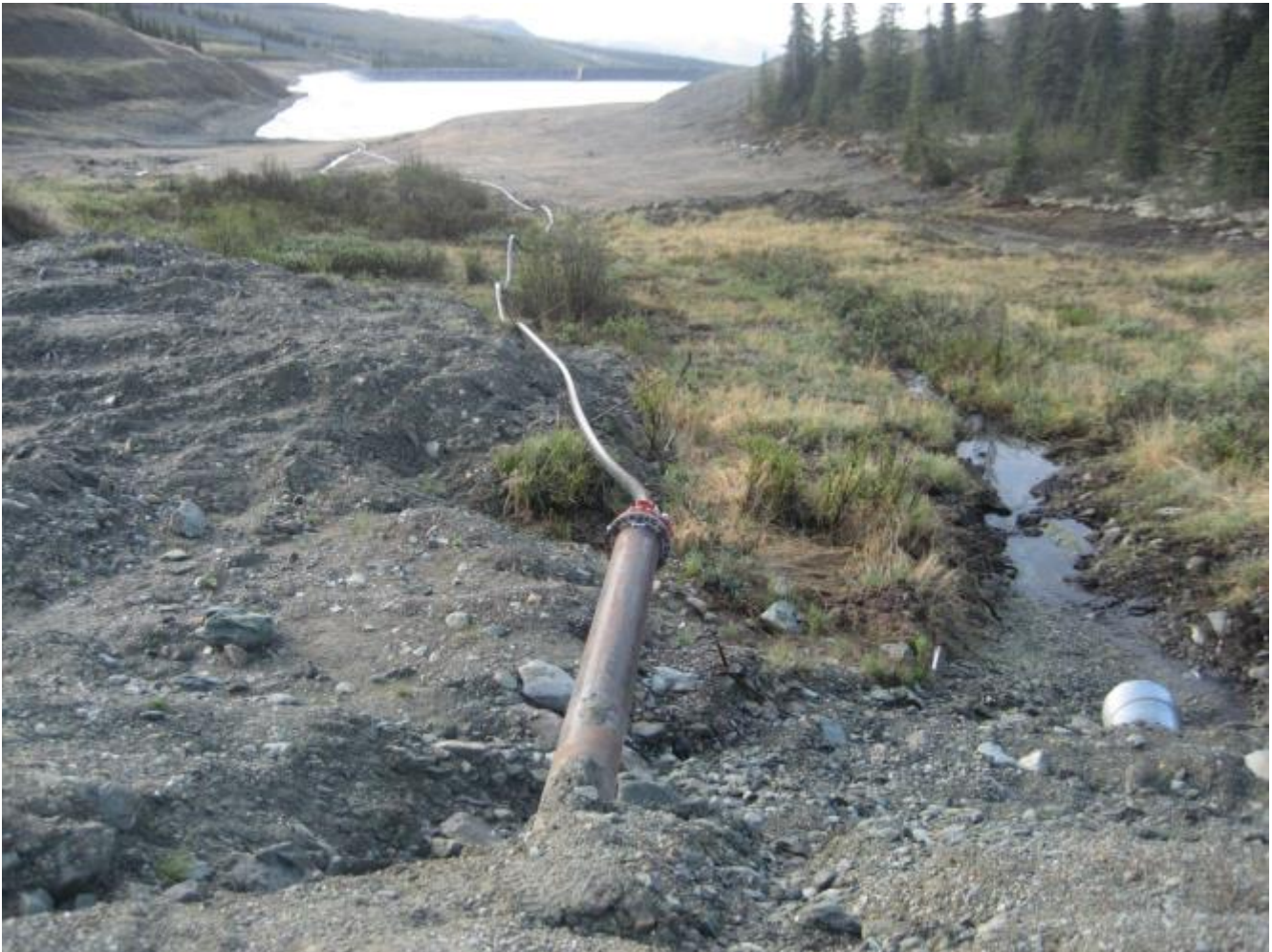
Photo 32 Waste Rock Seepage and Underdrain outlets
