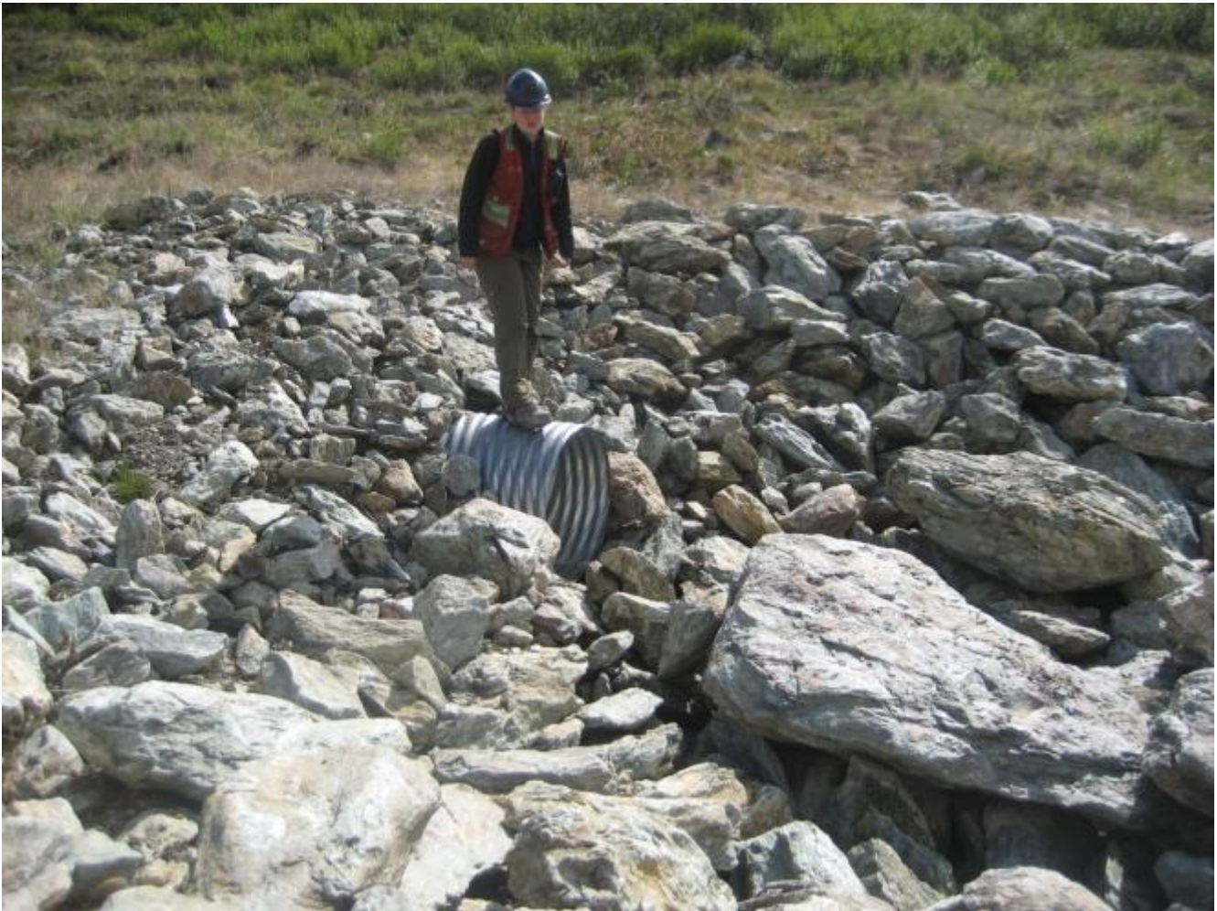
Photo 19 Diversion B culvert outlet
