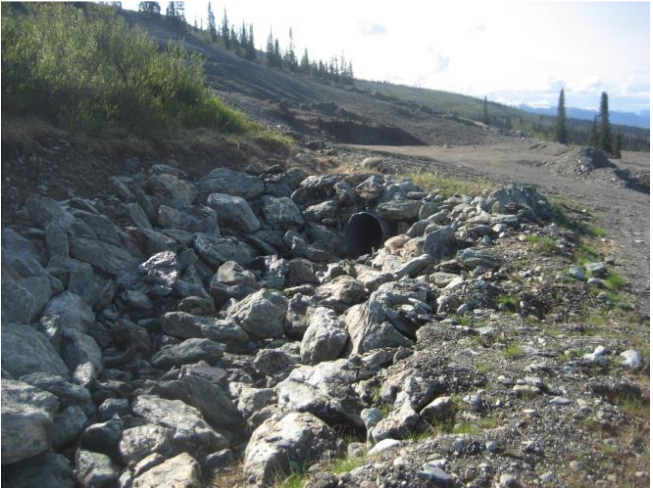
Photo 18 Diversion B culvert inlet
