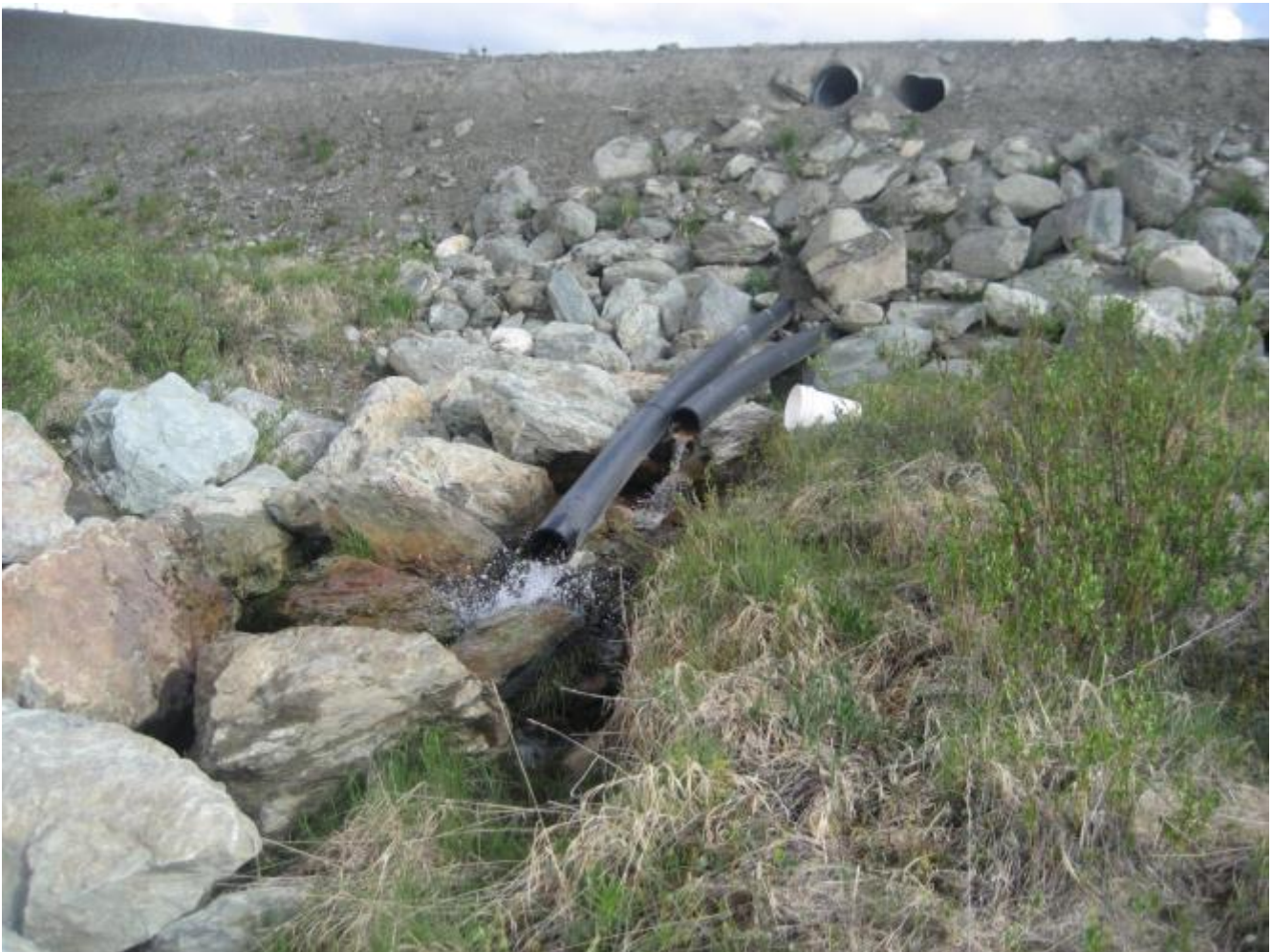
Photo 14 Underdrain outlet
