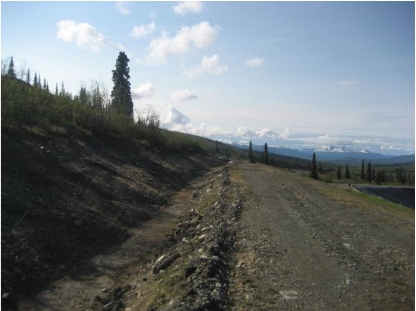
Photo 17 Diversion B looking downstream
