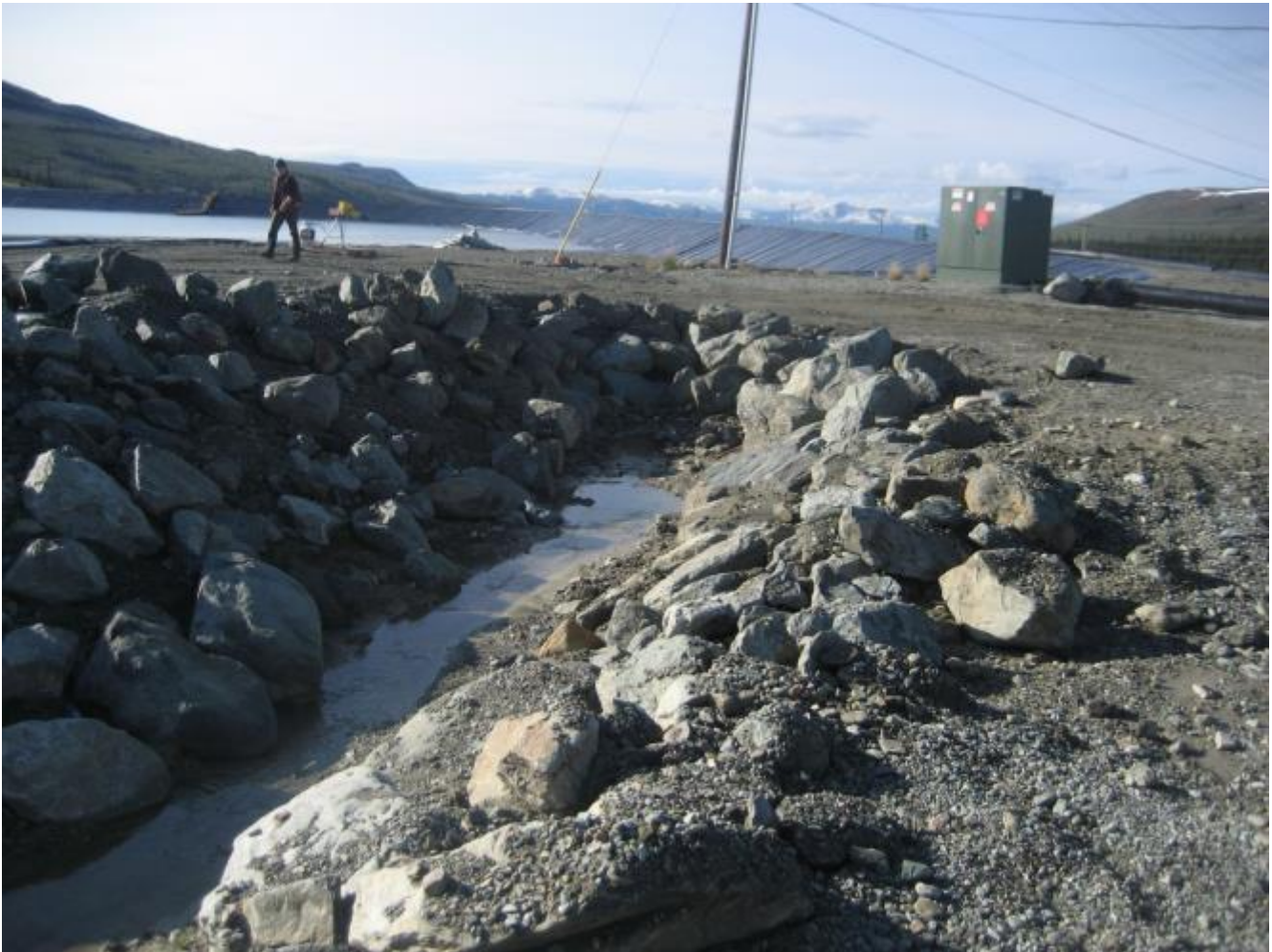
Photo 21 Diversion A culvert inlet
