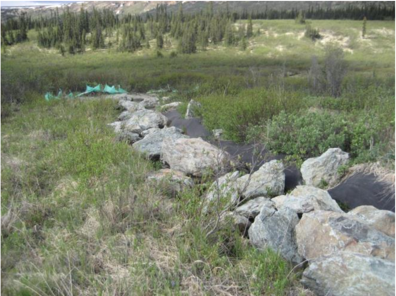
Photo 15 Downstream of underdrain outlet
