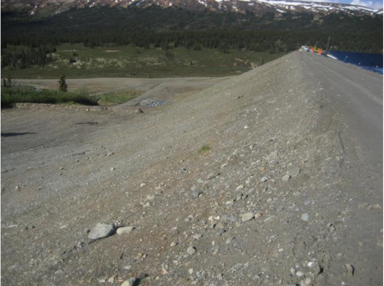
Photo 1 Dam crest and downstream face
