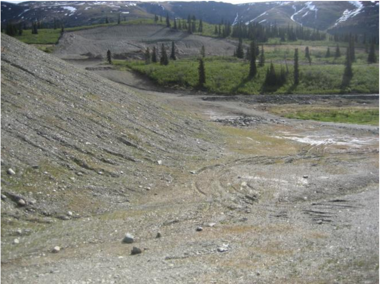
Photo 12 Toe of Southeast arm of dam
