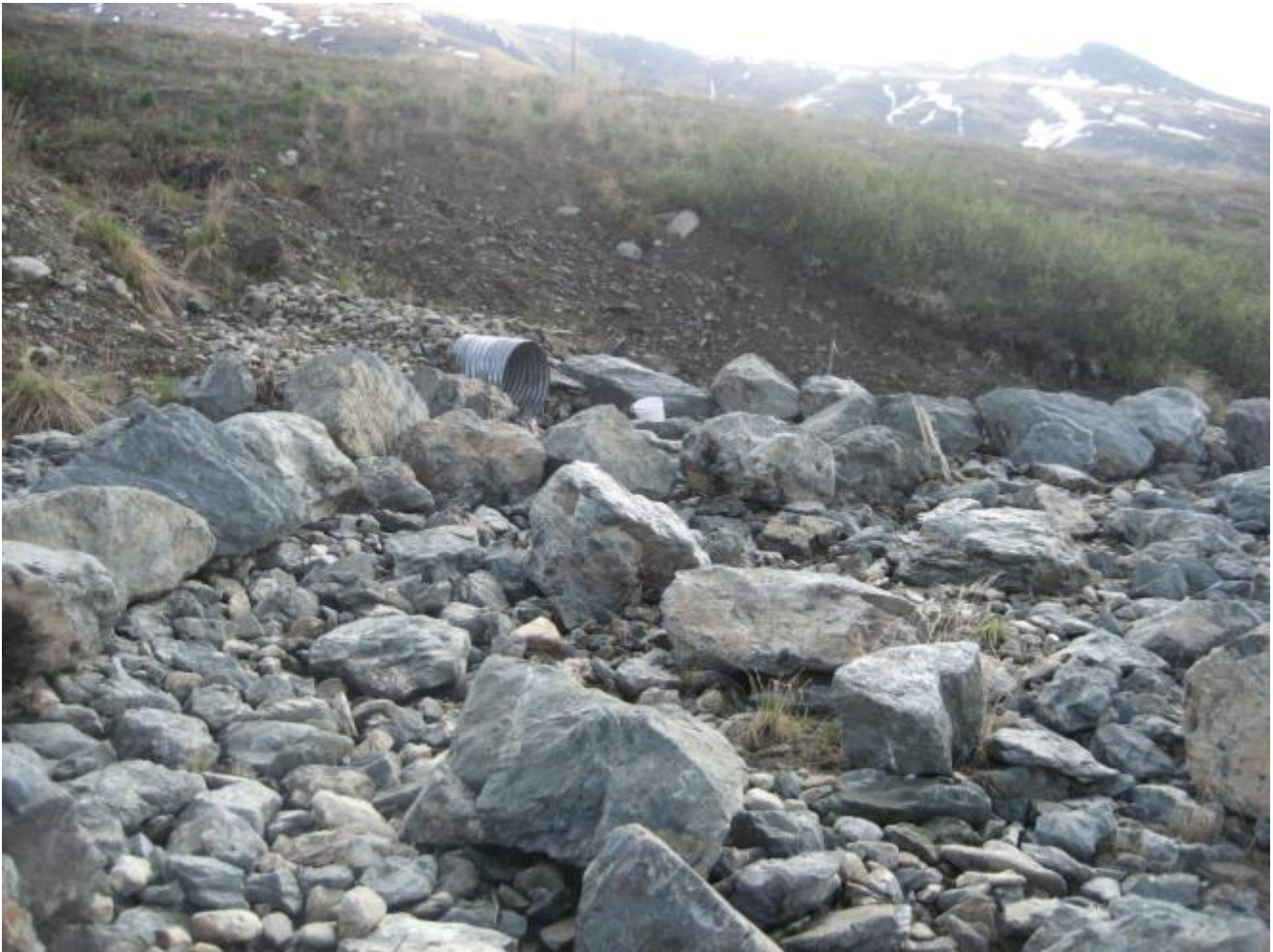
Photo 22 Diversion A culvert outlet
