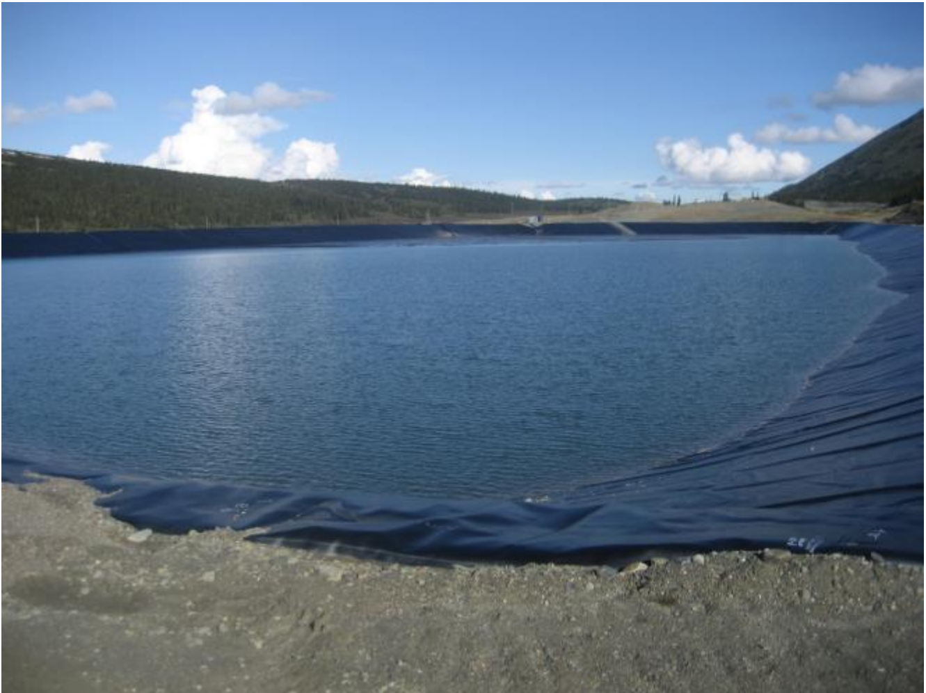
Photo 9 Impoundment from east abutment looking north
