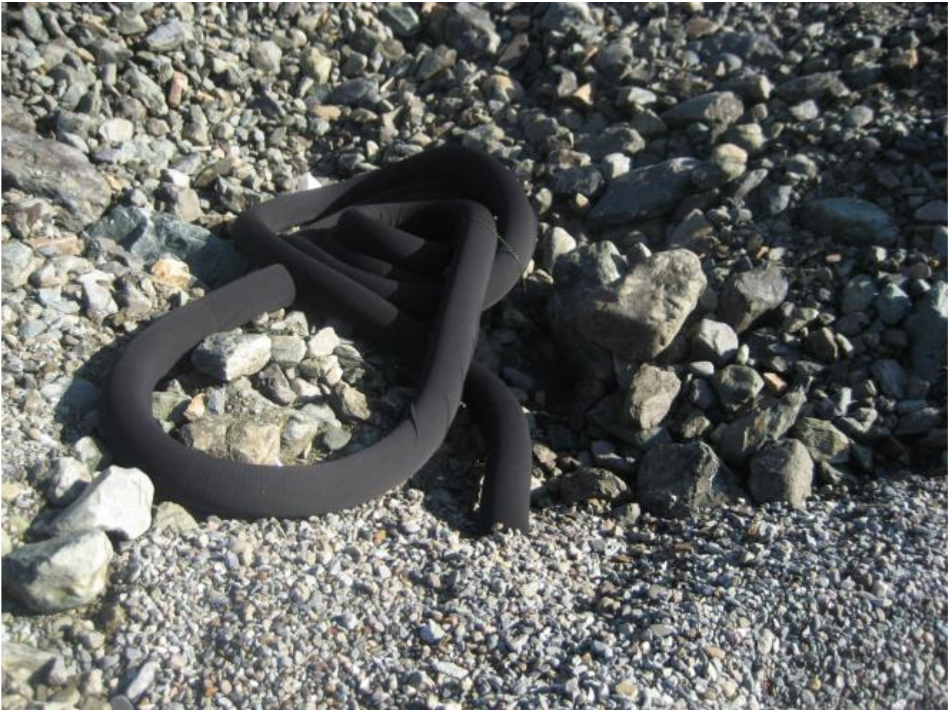
Photo 13 Underdrain inlet north of impoundment
