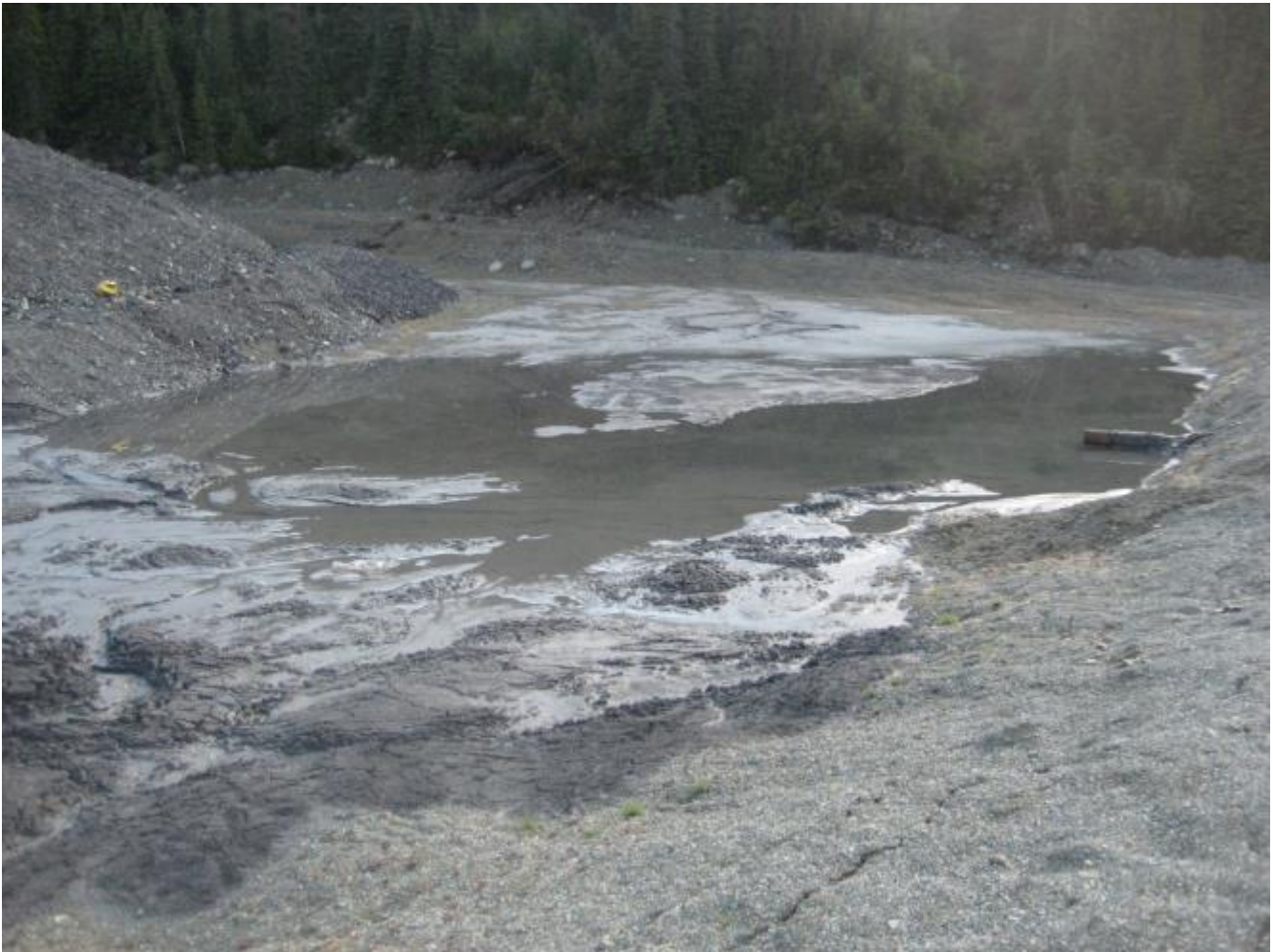
Photo 31 Waste Rock Seepage Collection
