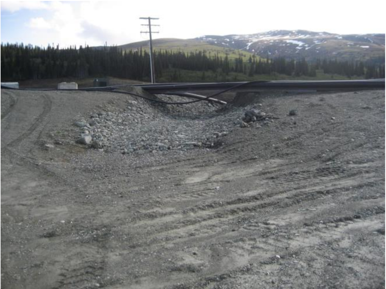
Photo 16 Spillway taken from Mine Access Road
