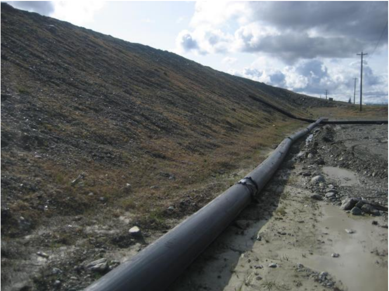
Photo 11 Toe of West arm of dam
