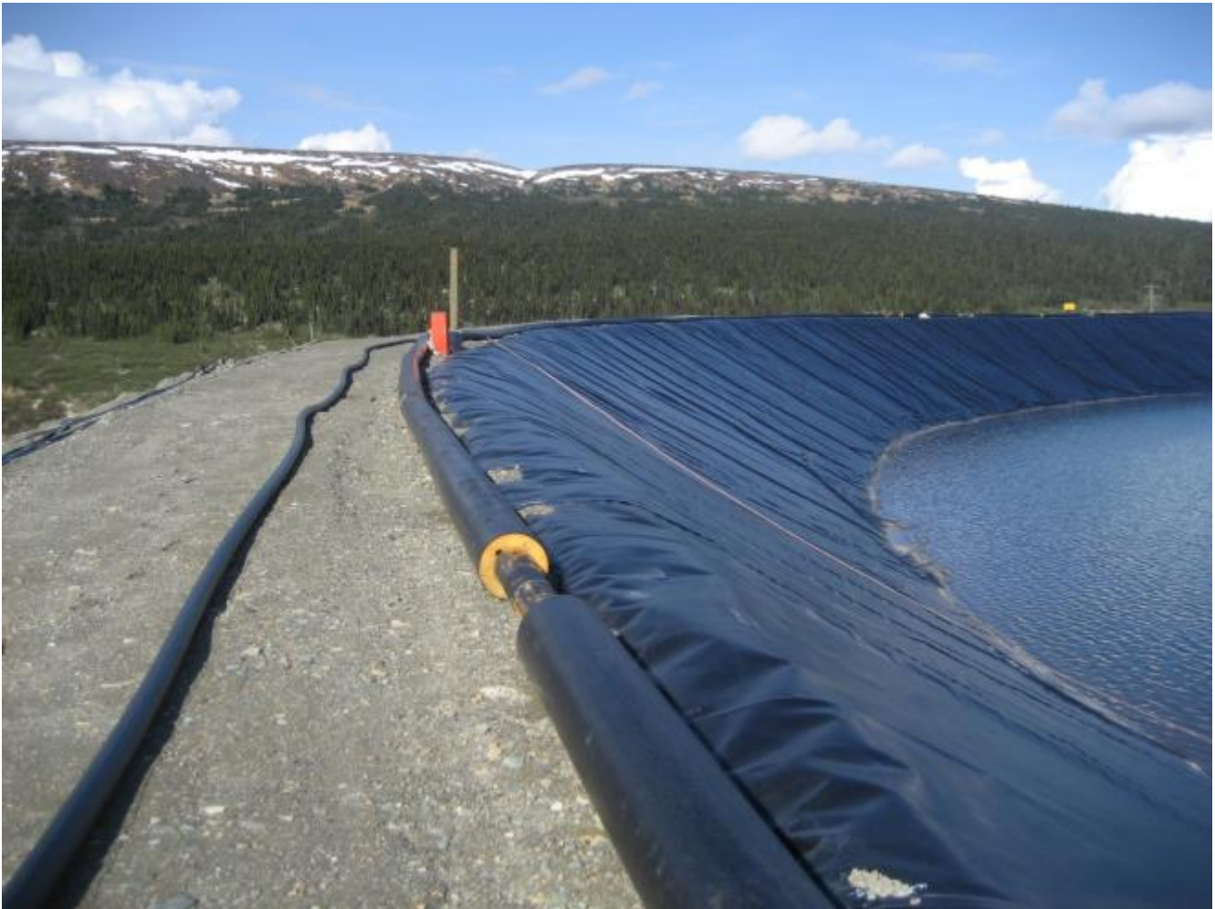
Photo 5 Reclaim Line and upstream dam face
