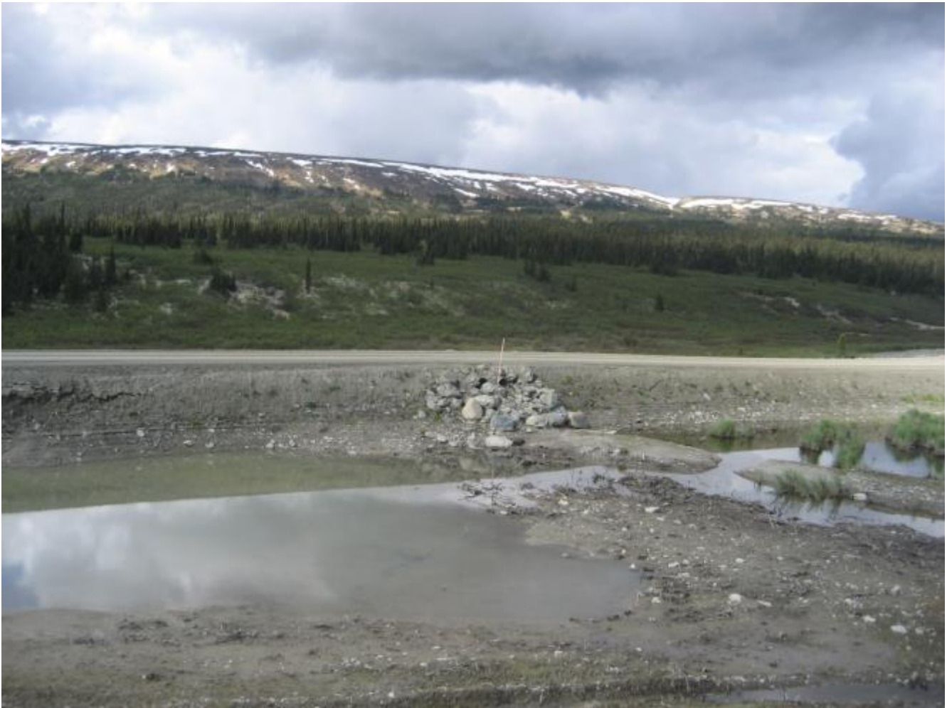
Photo 29 Seepage Collection Basin Spillway
