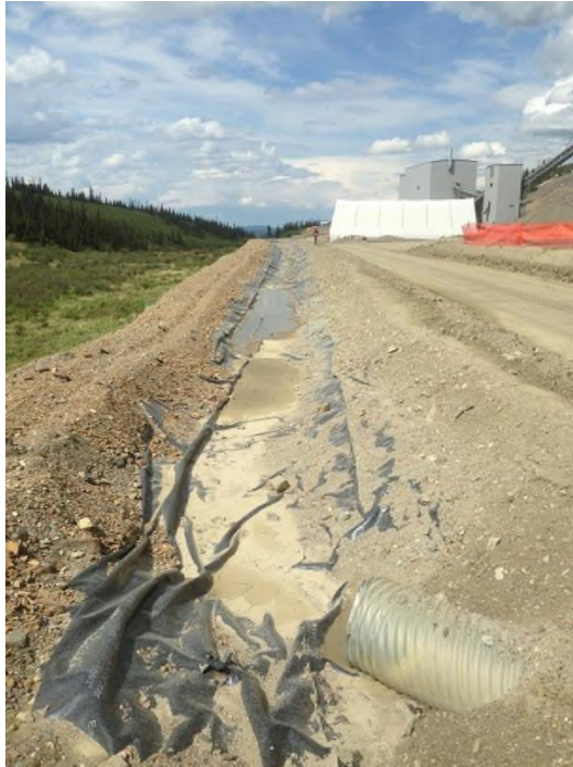
Photo 14 The reconstructed Ditch 3. (June 24, 2014)
