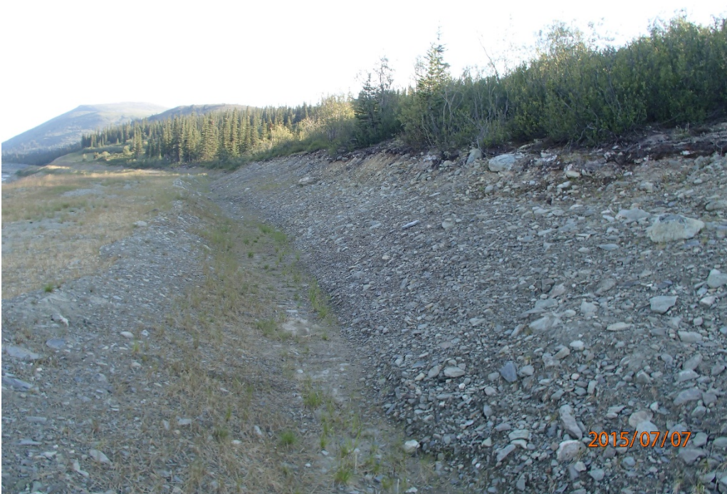
Photo 31 Ditch B – parallel to the TSF looking north
