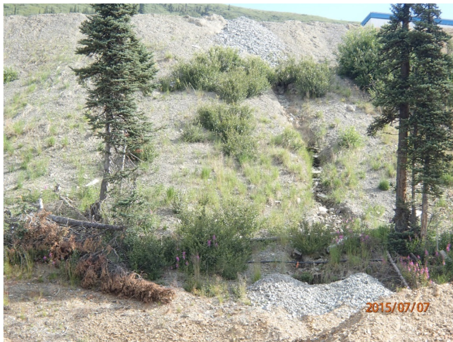
Photo 33 Camp pad – erosion channel in cut slope in south wall, partially backfilled with rock (west end)
