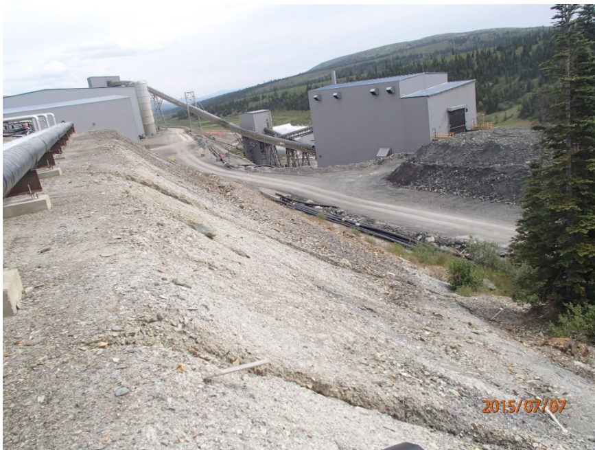
Photo 7 Fuel Tank farm and Genset Pad – downslope at south side looking towards crusher building, minor erosion gully
