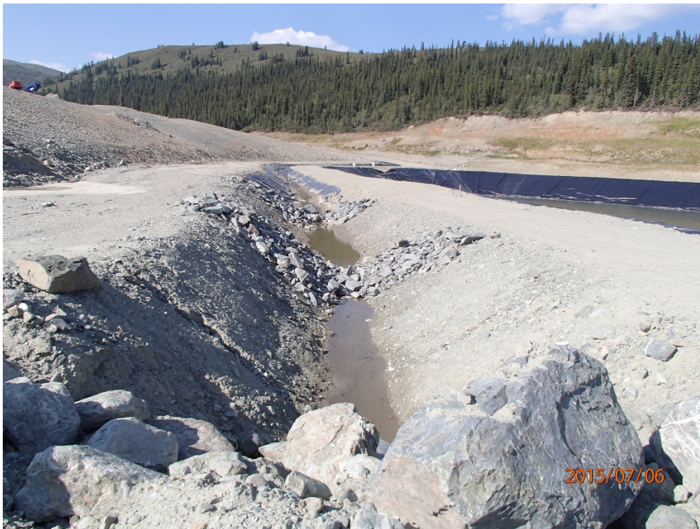
Photo 25 Ditch A – unlined part beyond the west end of TSF
