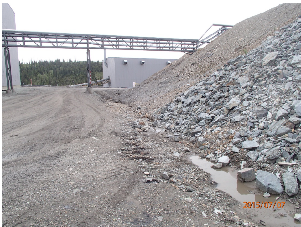
Photo 30 Ditch 5 –looking south
