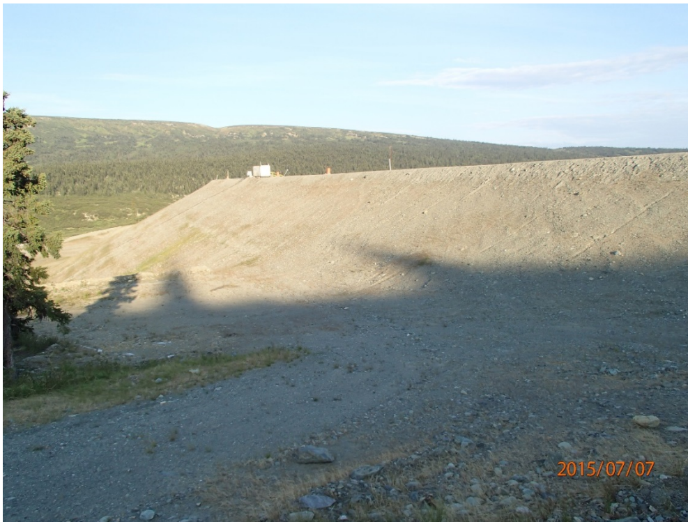
Photo 4 South dam – downstream slope, looking west
