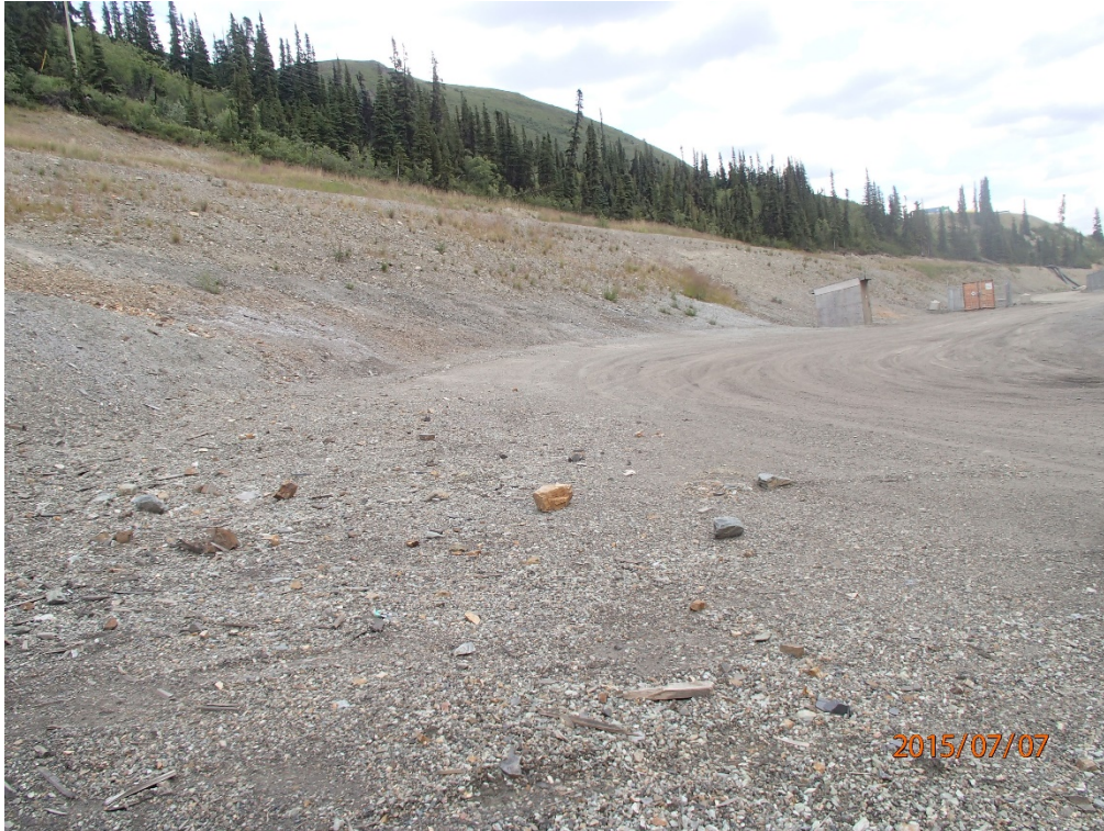
Photo 1 Mill building pad – upslope behind the Mill building
