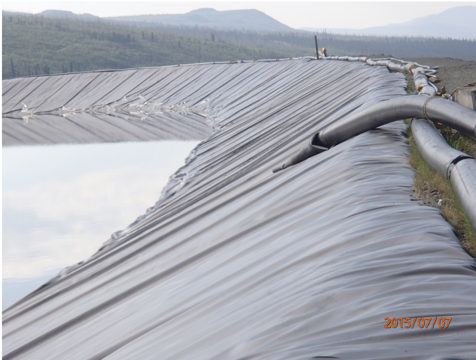
Photo 12 West dam – upstream slope, looking south
