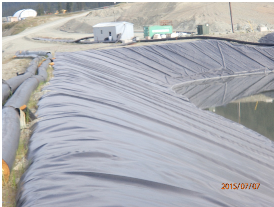
Photo 11 West dam – upstream slope, looking north
