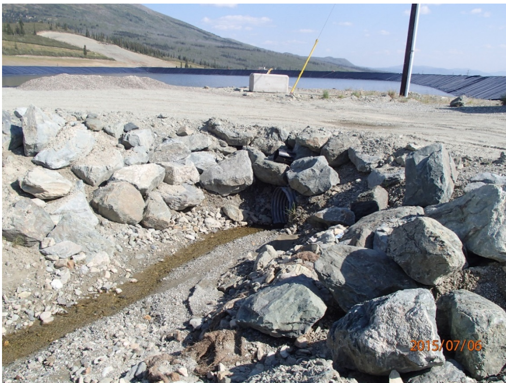
Photo 23 Ditch A – inlet to Ditch A culvert
