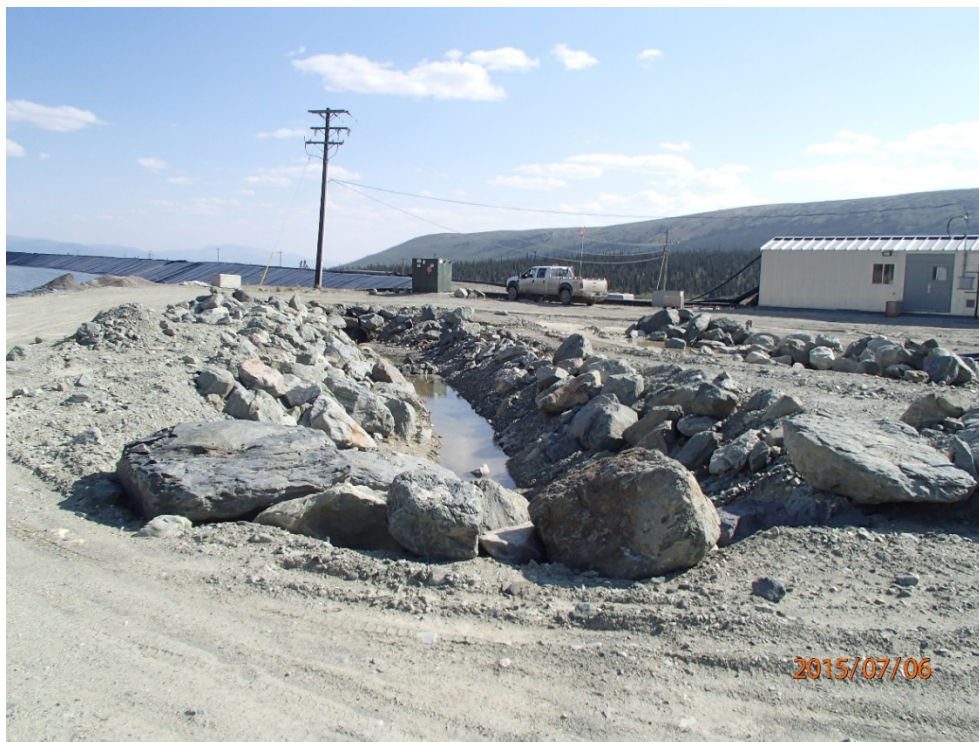
Photo 26 Ditch A – Rip-rapped section south of upper culvert
