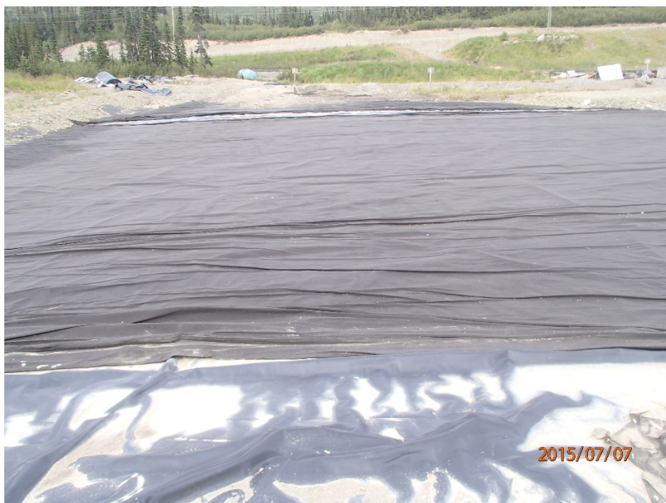
Photo 45 Land Treatment Facility – cover
