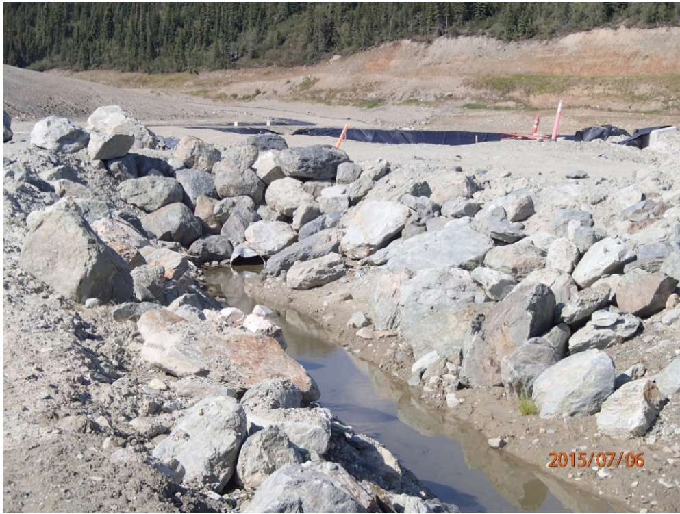
Photo 24 Ditch A – outlet end of the upper culvert for Ditch A
