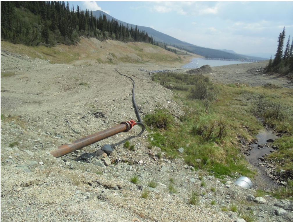
Photo 37 Waste Rock Storage Area - seepage and underdrain outlet
