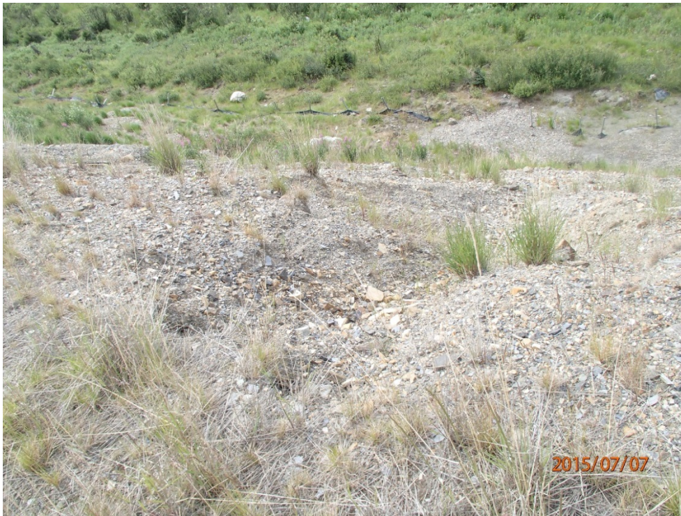
Photo 27 Ditch 4 – erosion channel in the downslope
