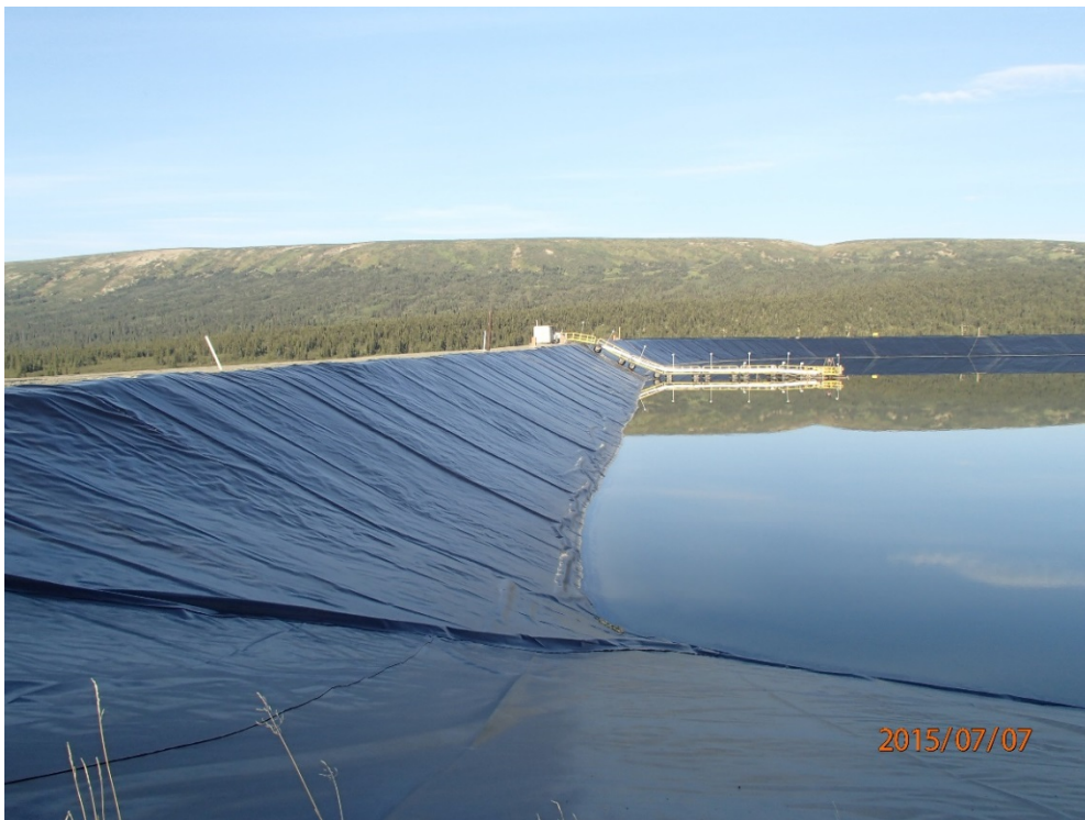
Photo 5 South dam and east abutment – upstream slope
