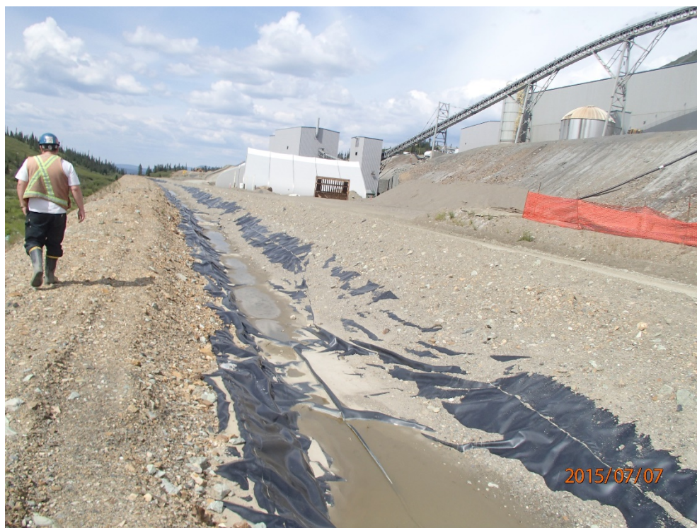
Photo 23 Ditch 3 – looking west, channel bed filled with silt and gravel
