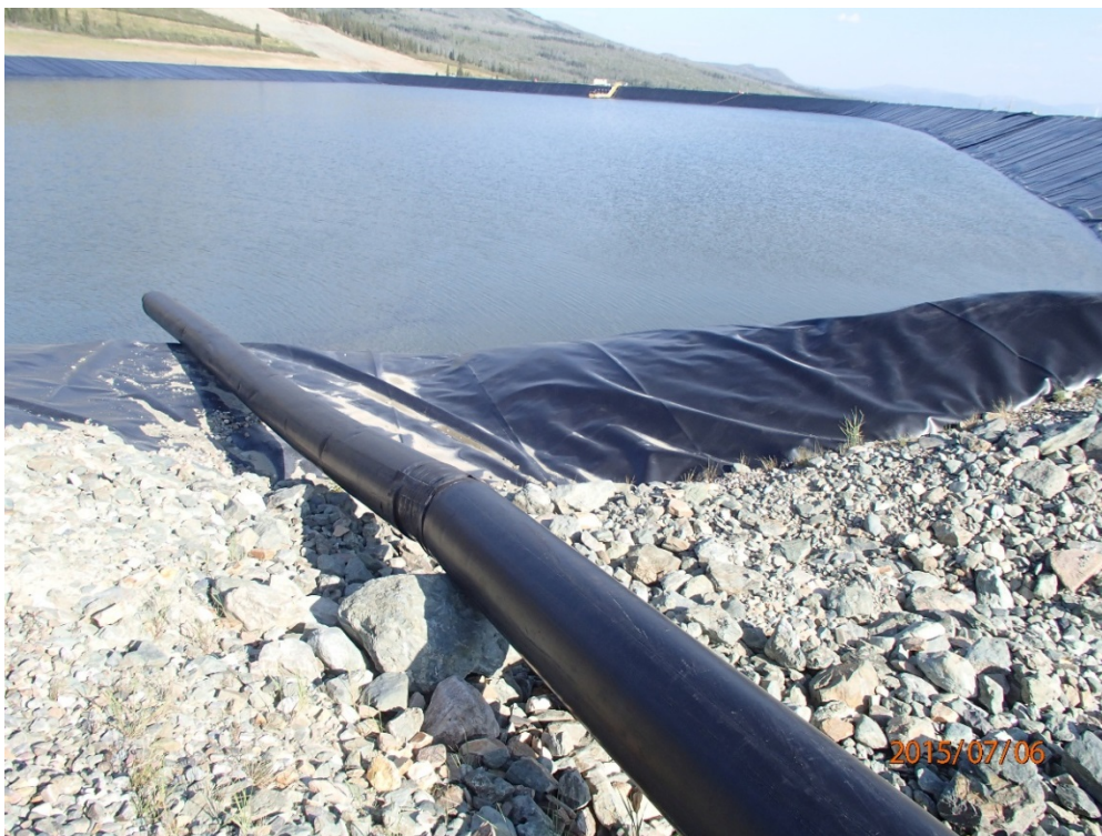
Photo 35 8 inch tailings line over the spillway
