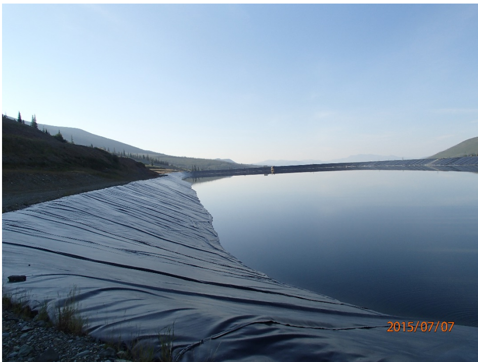
Photo 13 TSF east side liner –looking south
