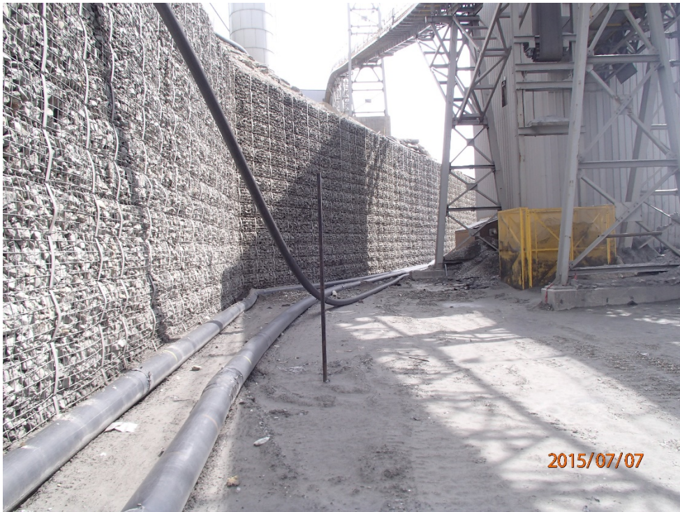
Photo 5 MSE wall – below the conveyor belt
