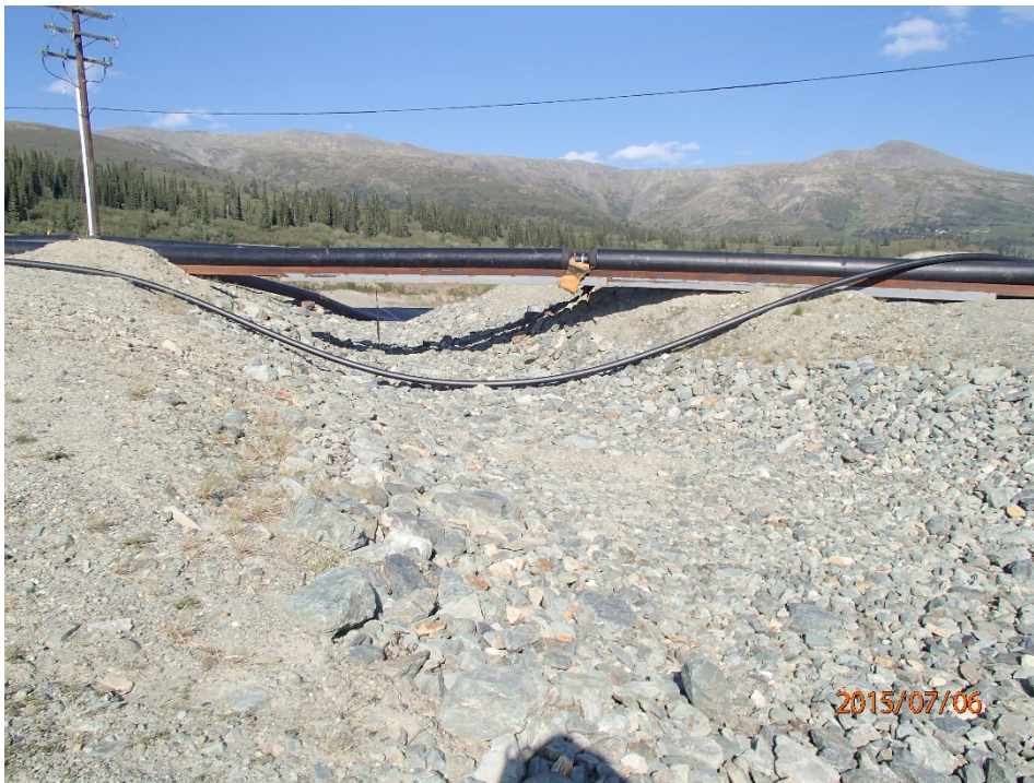
Photo 16 Spillway – looking upstream
