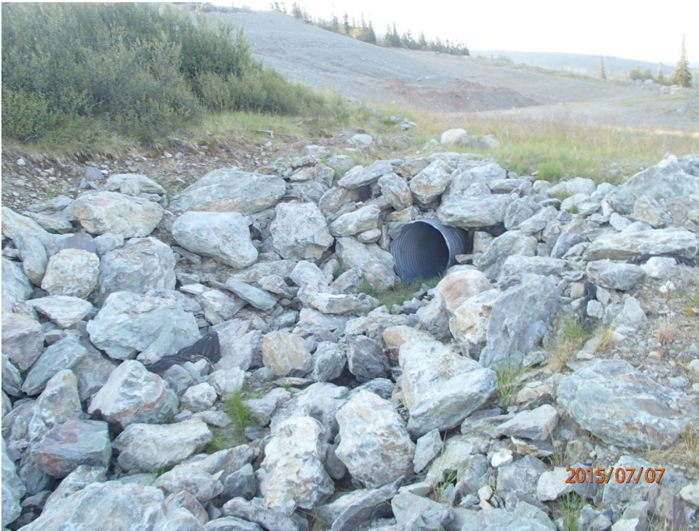
Photo 30 Ditch B – inlet of Ditch B culvert; no flow
