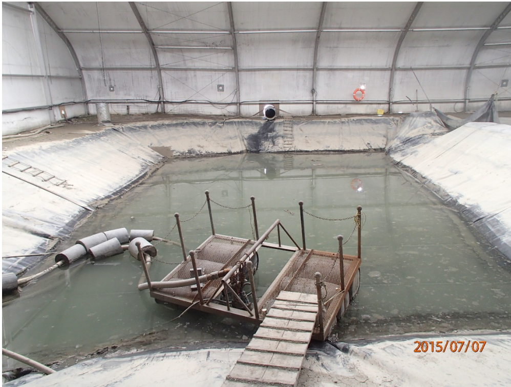
Photo 10 Sump 2 – culvert outlet from Ditch 4 in west sump, dry
