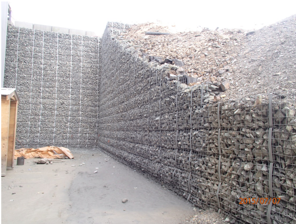
Photo 4 MSE wall – by the crusher building
