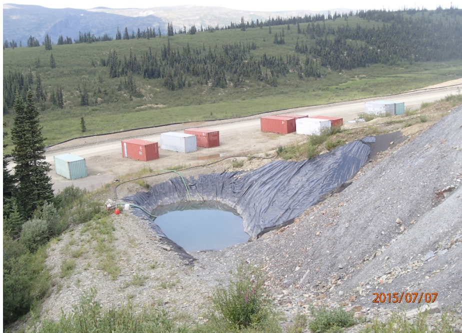
Photo 44 Ore stockpile area runoff collection sump – looking from the waste rock area
