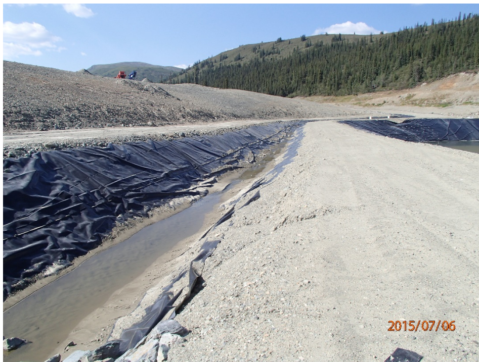
Photo 27 Ditch A – lined part
