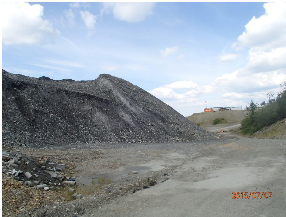
Photo 43 Waste Rock and Ore Storage Facility – inside slope
