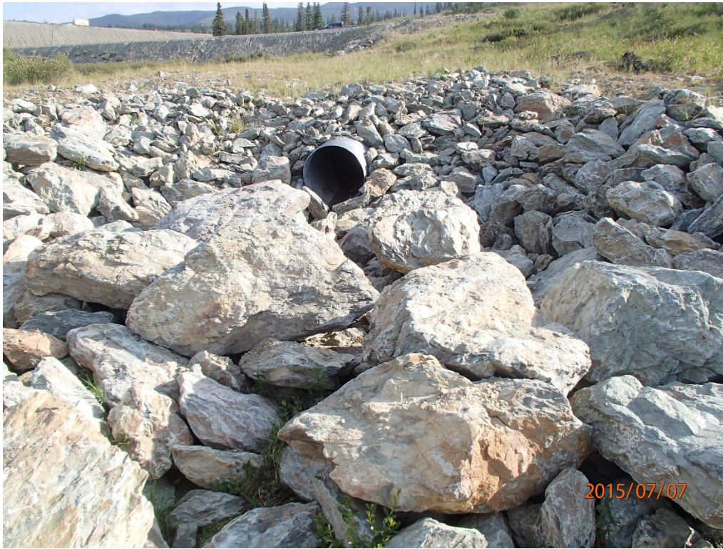
Photo 32 Ditch B – culvert outlet at stilling basin
