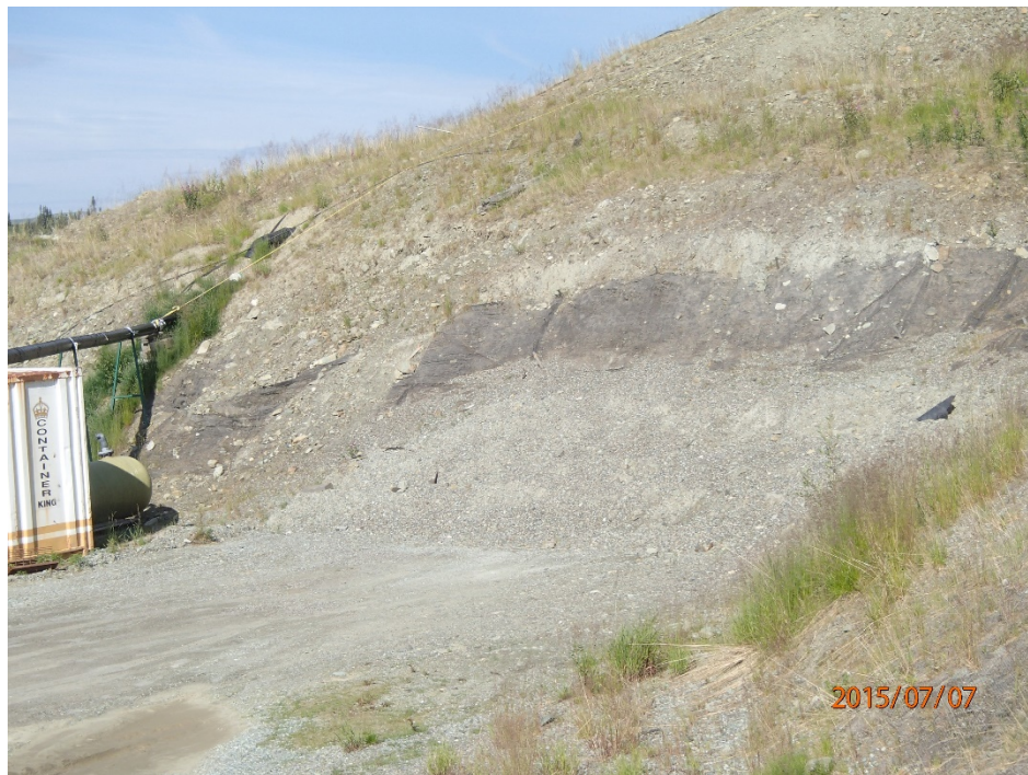
Photo 39 Sewage Treatment Plan Pad – Back slope
