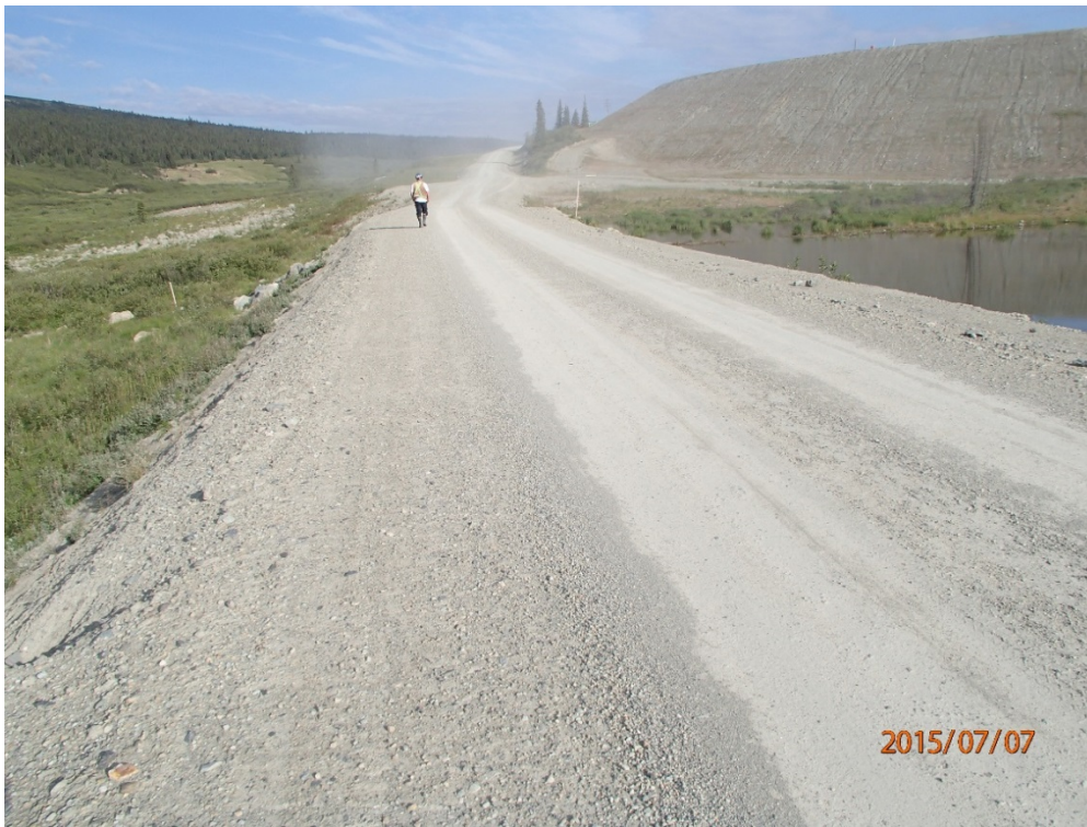
Photo 22 Seepage berm- looking north
