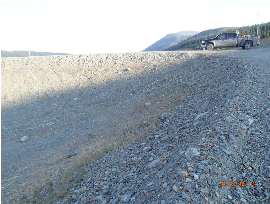
Photo 15 East (right) abutment – downstream side, looking north east
