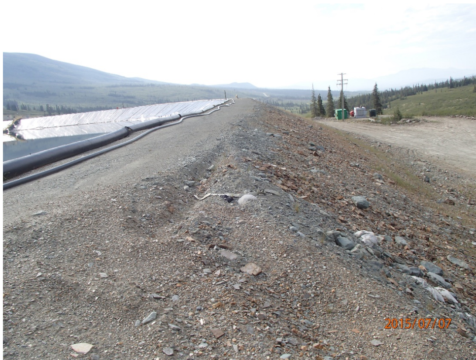
Photo 10 West dam –downstream slope, looking south, south of access ramp
