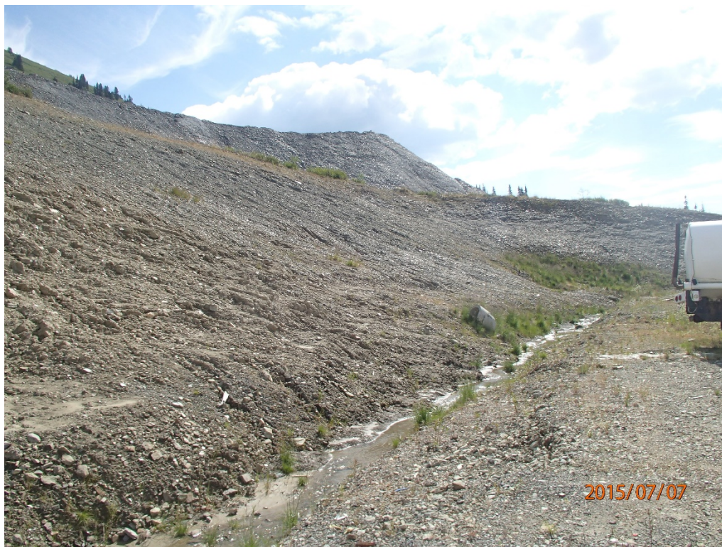
Photo 42 Waste Rock and Ore Storage Facility – outside slope
