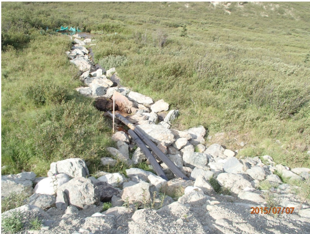
Photo 19 Underdrain outlet – downstream of seepage berm
