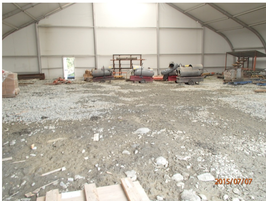
Photo 9 Sump 1 – decommissioned and backfilled, now used as covered laydown area
