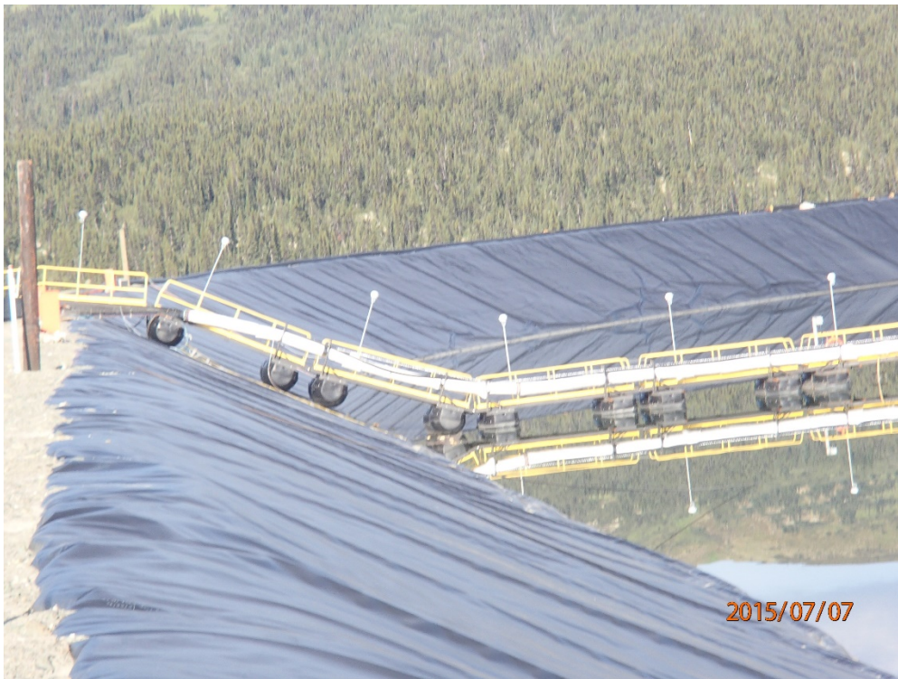
Photo 33 South Dam – Access ramp to reclaim barge on upstream slope
