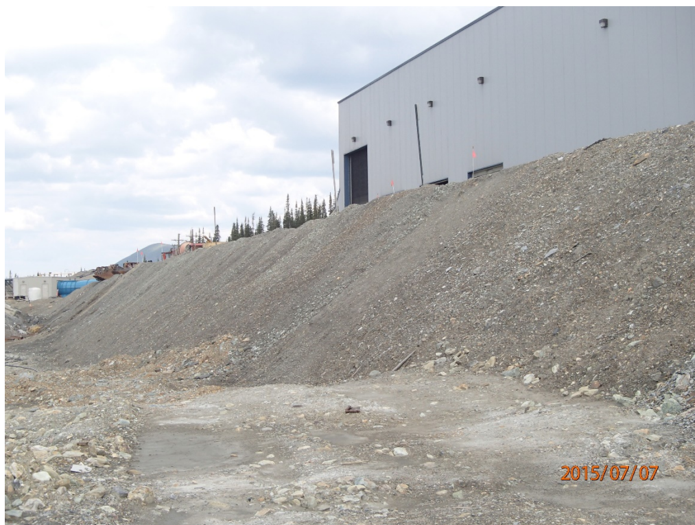
Photo 50 Truck shop pad – downslope, looking west
