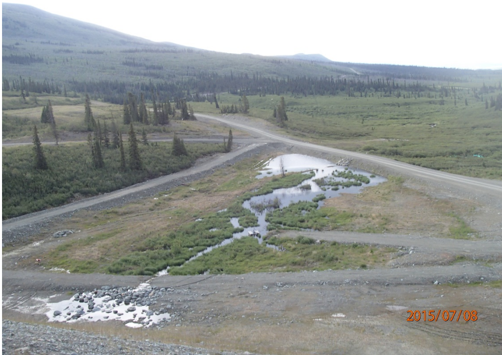
Photo 20 Seepage Collection Basin
