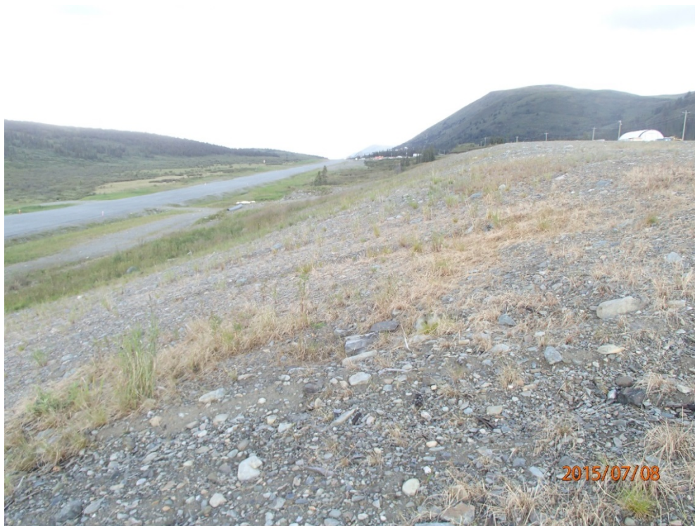
Photo 40 Northwest waste pile
