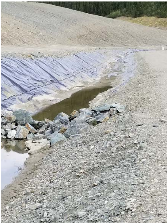
Photo 44 Lined section of Ditch A
