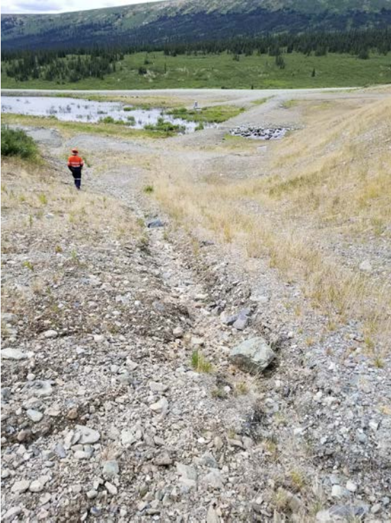
Photo 18 Minor erosion gullies on downstream slope
