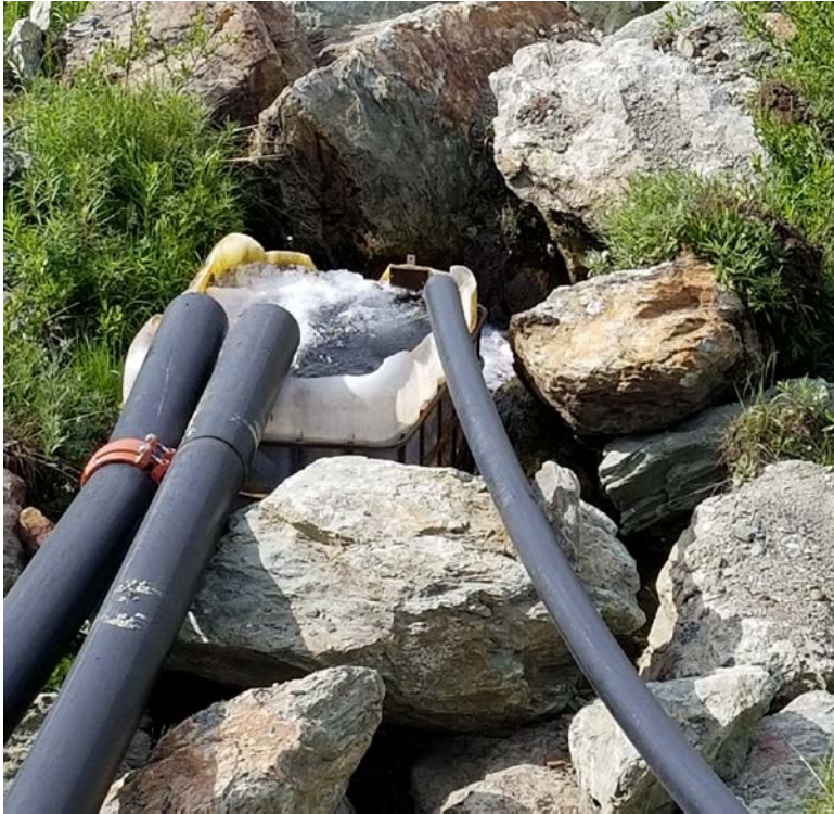
Photo 12 Upstream end of under drains
