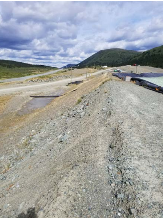
Photo 22 Minor ponded water from recent rainfall
