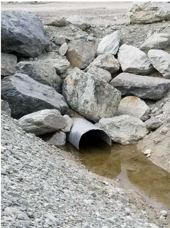
Photo 42 Ditch A Culvert leading to discharge point
