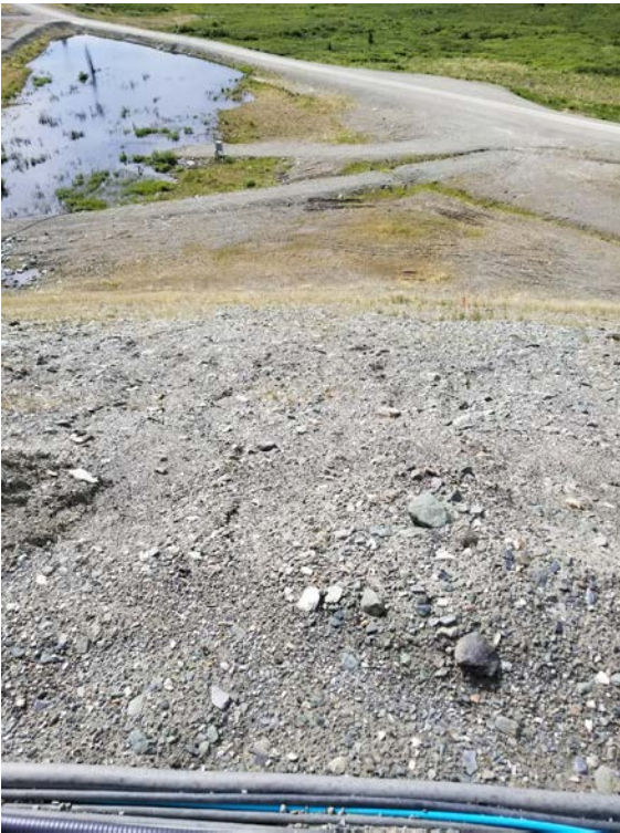
Photo 18 Minor erosion gullies on downstream slope
