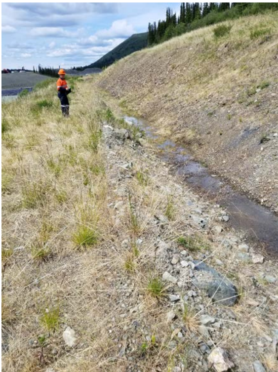
Photo 30 Ditch B Some Ponding Water
