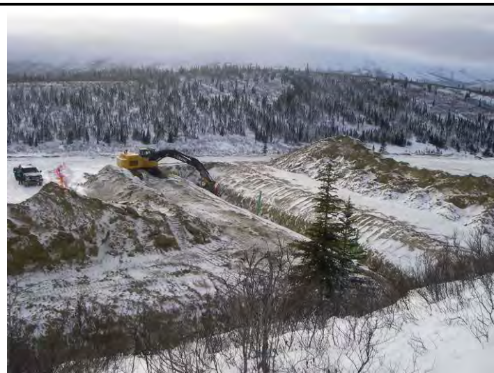
11-02-08 Excavation of the north side underground utility corridor – facing SW
