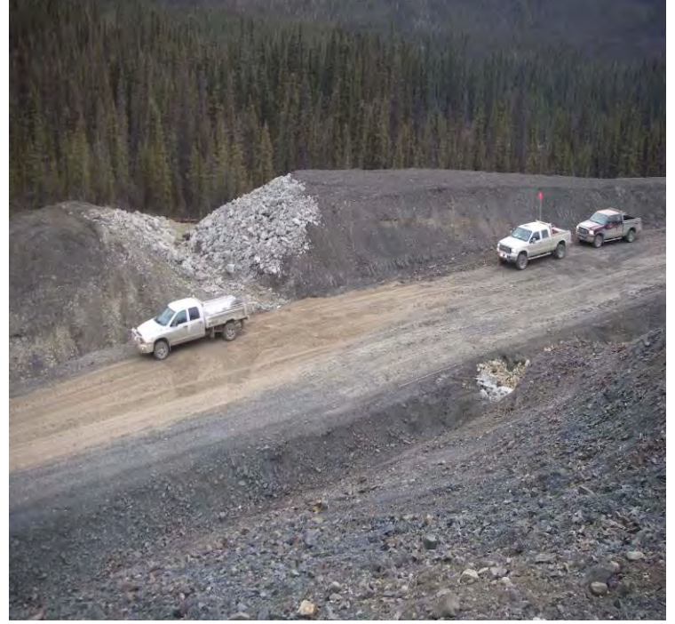
10_15_08 Facing d/s, cross-drain for culvert and ditchblock on UC side of bridge
