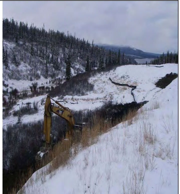
10_18_08 Facing North, bench built at toe of portal pad to accept the new pipeline
