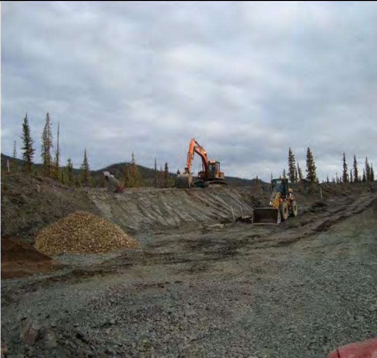
Bunker Creek: up chain landscaping and drain rock hauling for UC bin wall. 09_25_08 (facing UC)
