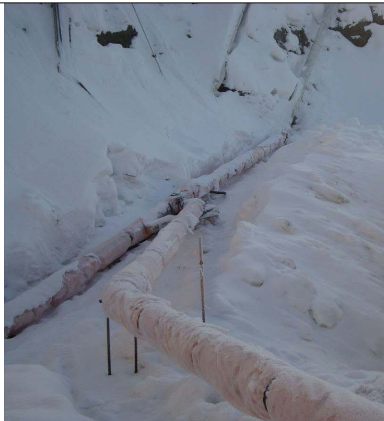
12-13-08 Steel to HDPE connections at Portal adit adjacent to the multiplate (facing SW)
