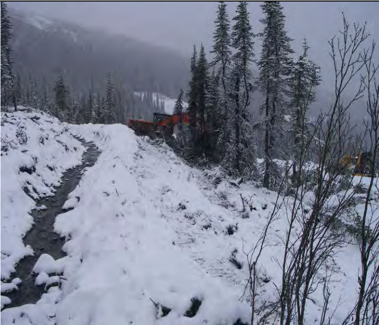
10_17_08 Facing UC km 15+100 looking at the diversion for excavating the high ditch further downslope, but still offset from the road.
