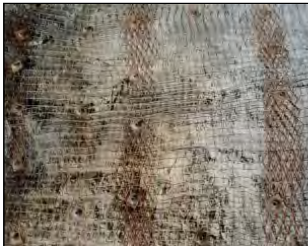
Picture 4-4: Rock bolt and screening completed on the left side of portal, 9/22/08.
