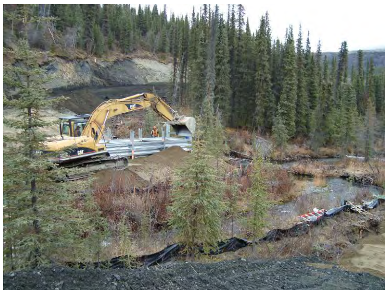
09_29_08 Down chain bin wall backfill (facing DC)
