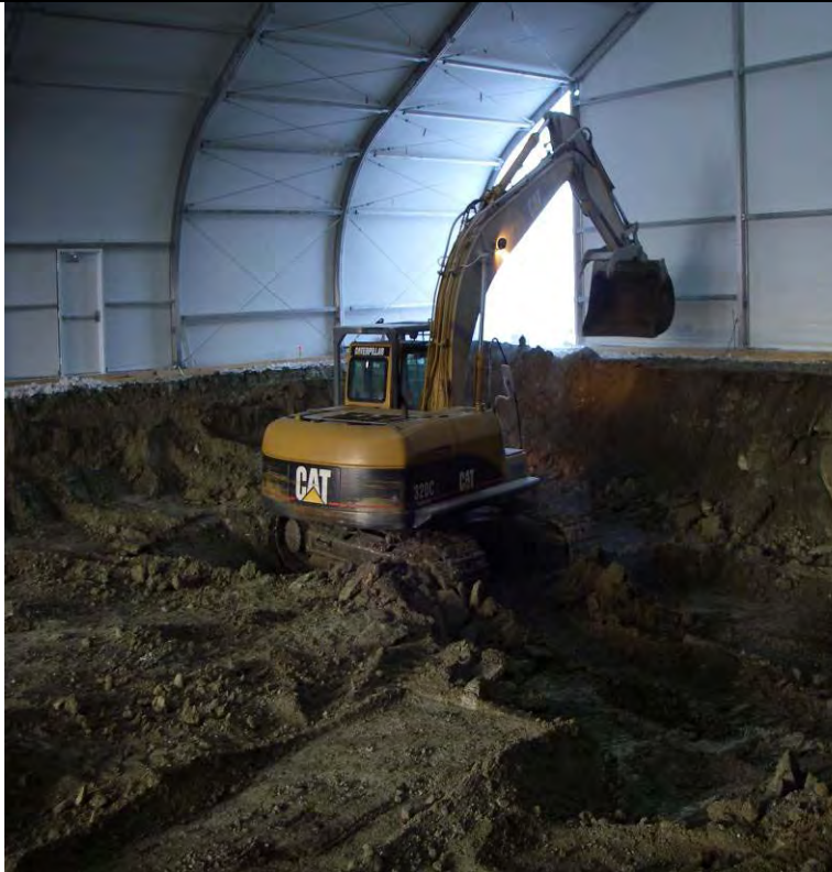
11-07-08 Excavation of the 2000 m 3 sump – facing NW
