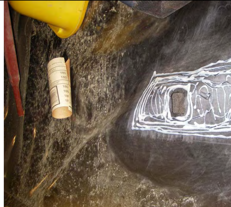
12-07-08 Liner puncture repair at Southwest corner of pond using 20:1 3M repair kit
