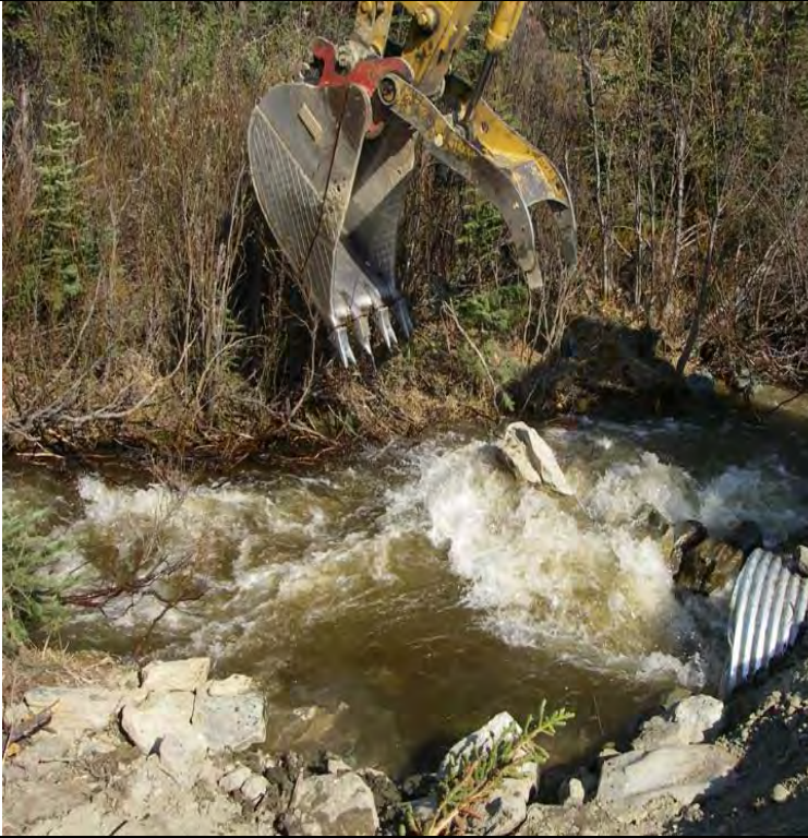
Photo 5 - 05/27/08 - Placing Cobble to align stream to 48" culvert. Looking u/s
