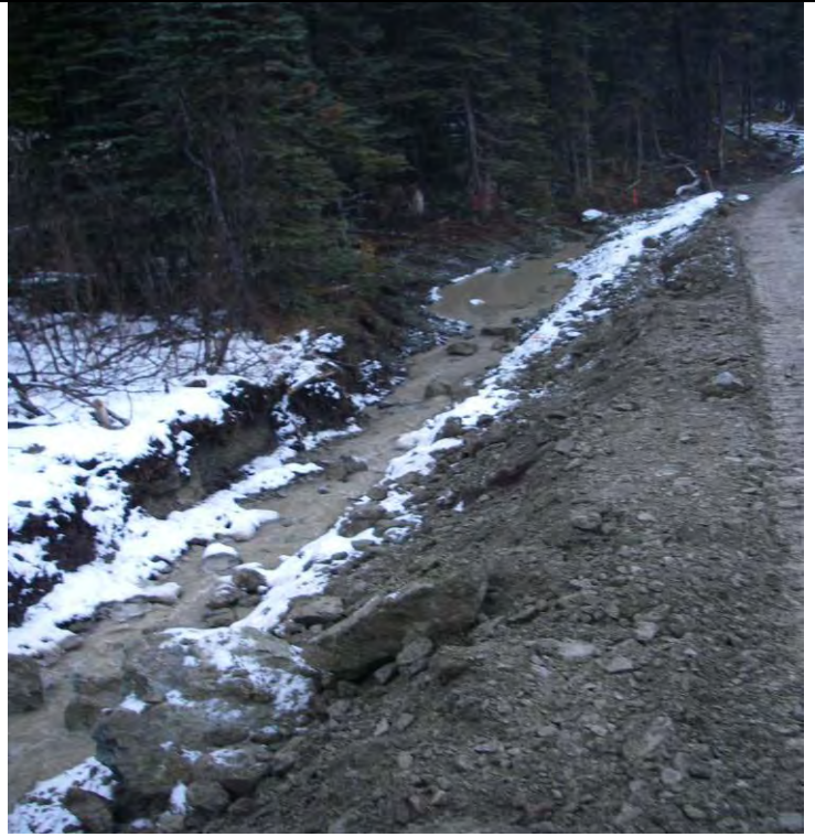
10_11_08 Looking DC at km 15cutslope ditch heavy siltation from earthworks no immediate d/s effects after culvert crossing after pool in background
