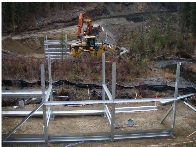
09_27_08 Up chain bin wall layout, and down chain install (facing DC)
