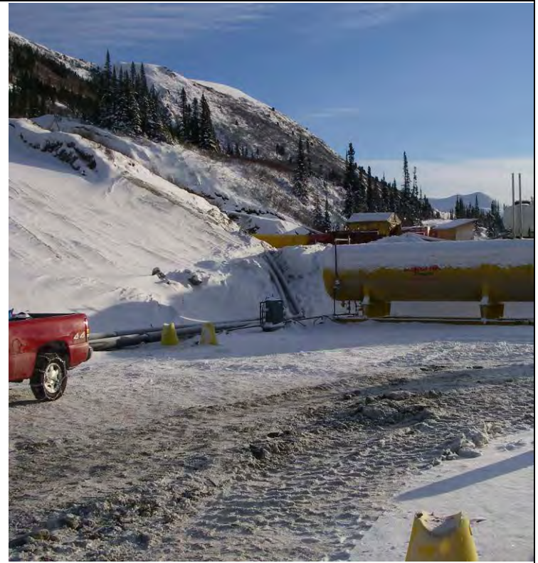
11-08-08 Propane tank and vaporizer and pipeline to left – facing S
