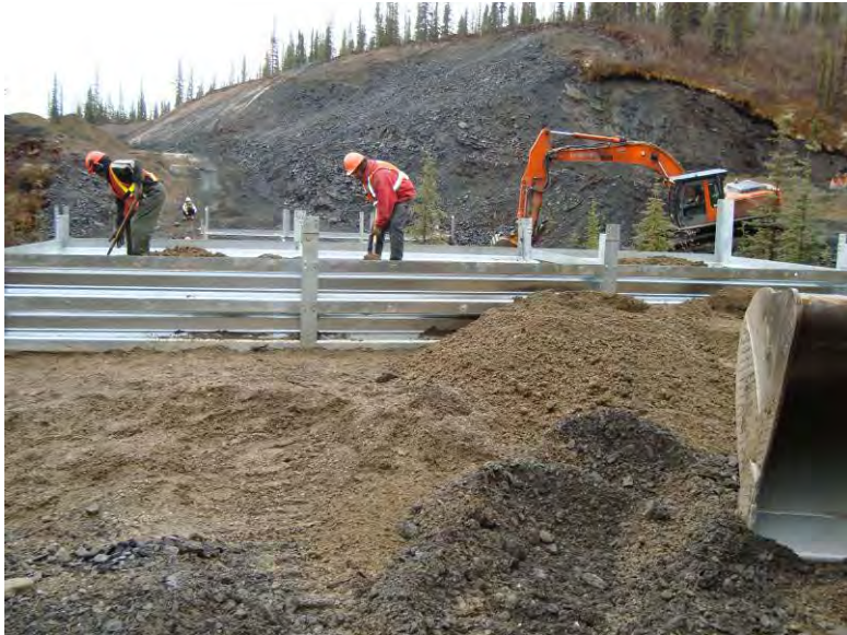
09_30_08 Loading and backfilling of down chain bin wall (facing UC)
