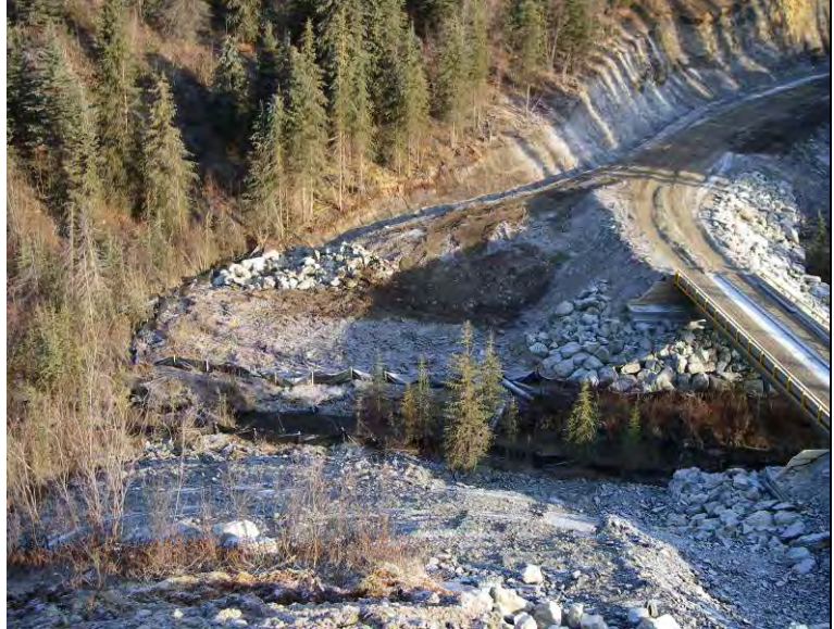
10_08_08 Facing DC, location of removed temporary bridge contoured and organics replaced. Pile of rip rap at location of energy dissipater
