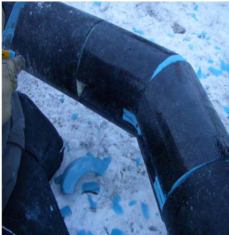
11-05-08 View of Elbow insulation kits and heat shrink, adjustments for kits required
