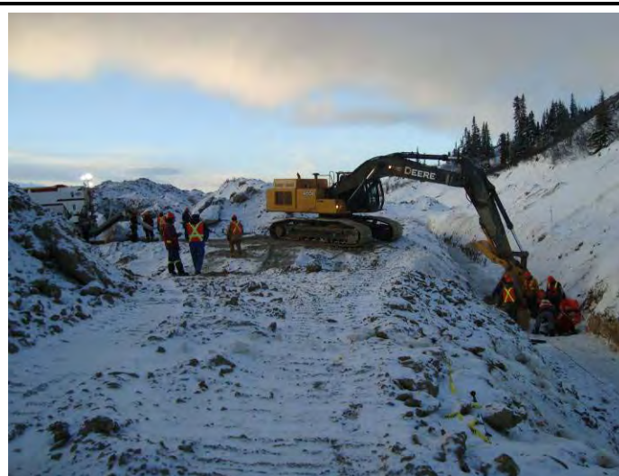
11-22-08 Filling thrust blocks with cement
