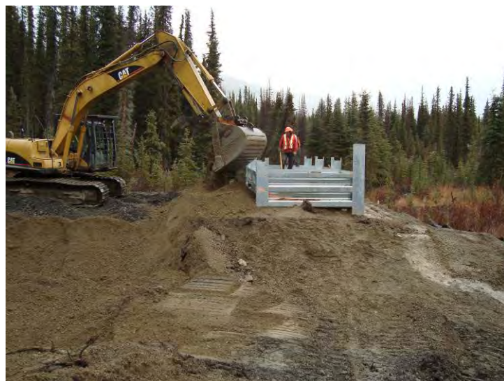
09_30_08 Loading and backfilling of down chain bin wall (facing downstream)
