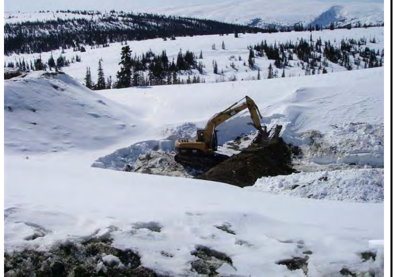
04/24/08 WRP berm being compacted and shaped
