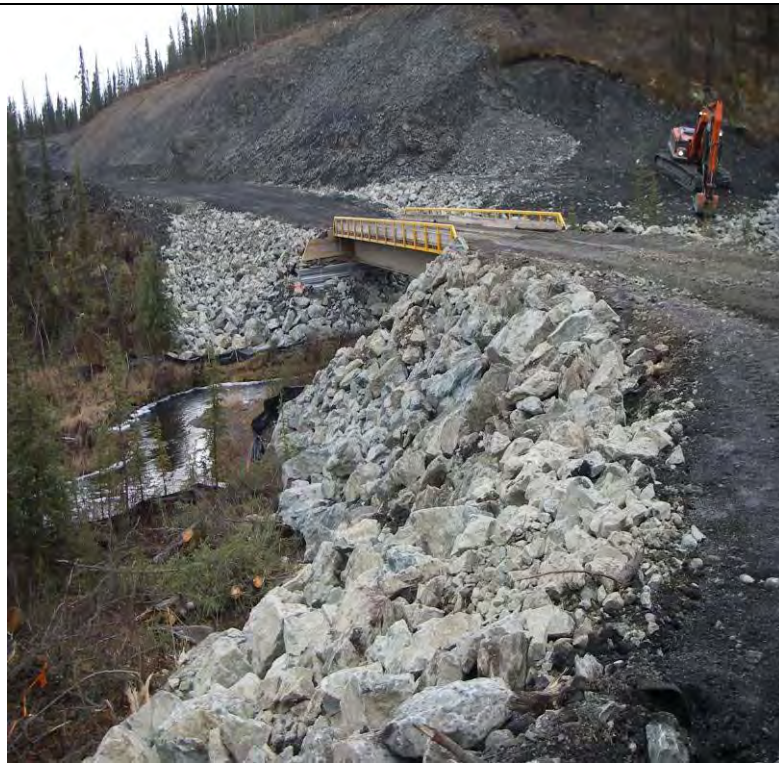
10_13_08 Facing UC, finishing the armouring and rock lined outflow on UC d/s side
