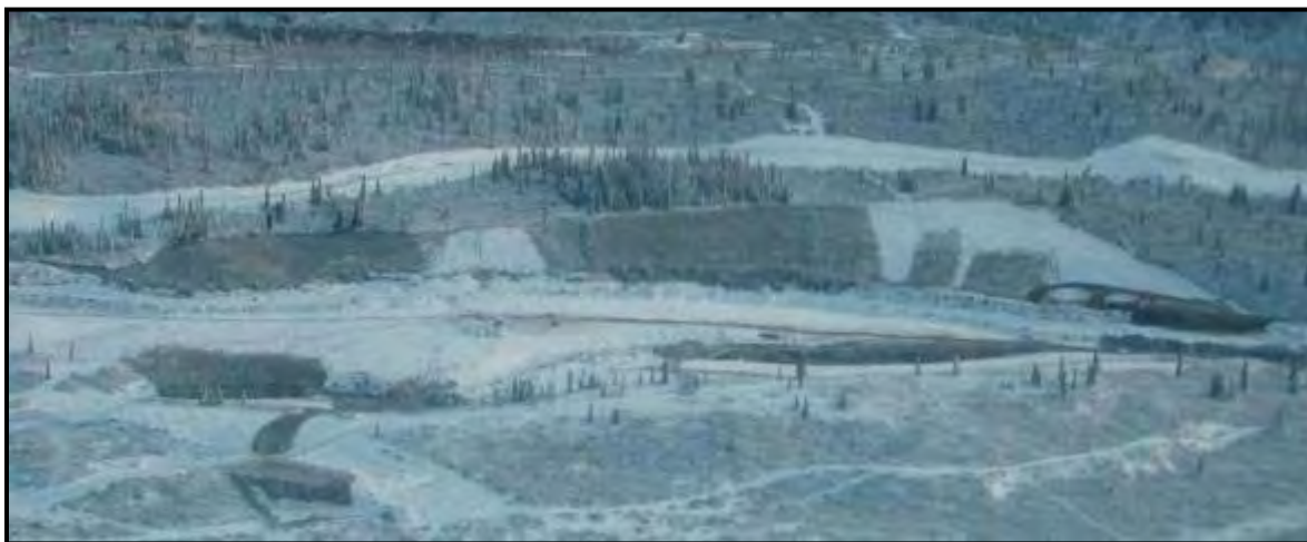
Picture 2-9: Looking east at stripping of organic material from within the tailings facility basin (Nov. 2008).
