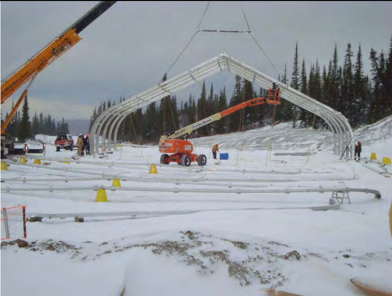
10_24_08 Sprung set up (facing North)
