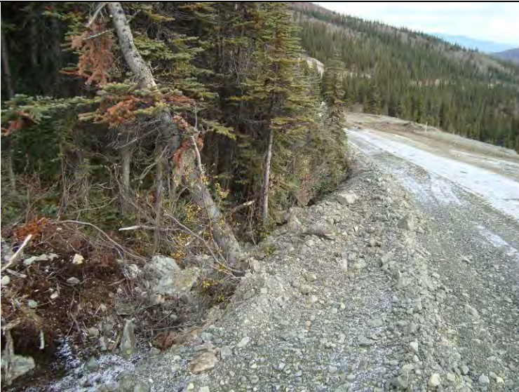
09_27_08 Upslope ditching not done, water draining underground (facing DC)
