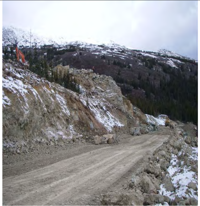
10_15_08 Looking DC at km 15+300 final scaling and loose rock clean-up
