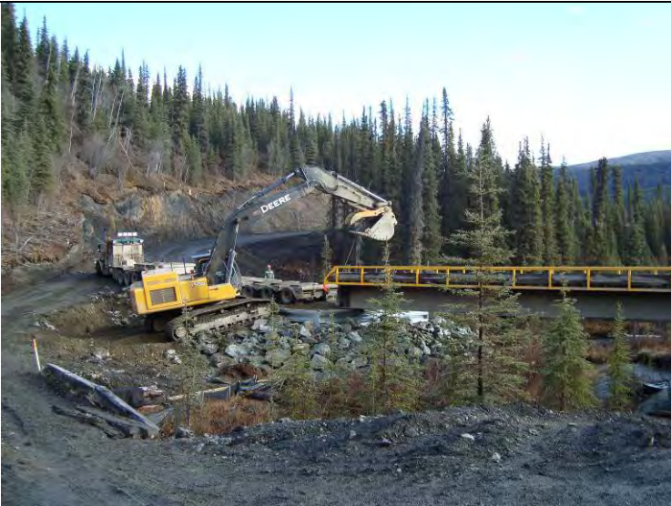
10_03_08 Facing (DS), lifting bridge off of low bed and onto bin wall below.
