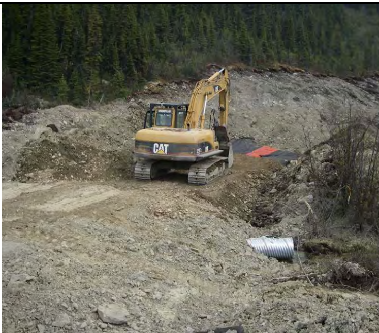
06/07/08 – Facing SE – Filling over snow fence and geotextile
