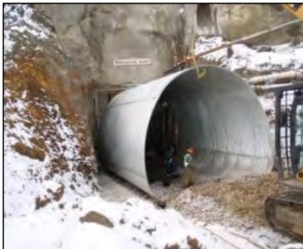
Picture 4-5: Multi-plate installed, 10/16/08.
