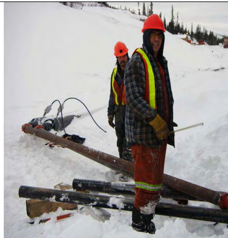
12-05-08 HDPE to Steel line connection outside Sprung for UG discharge and Mine Water Return
