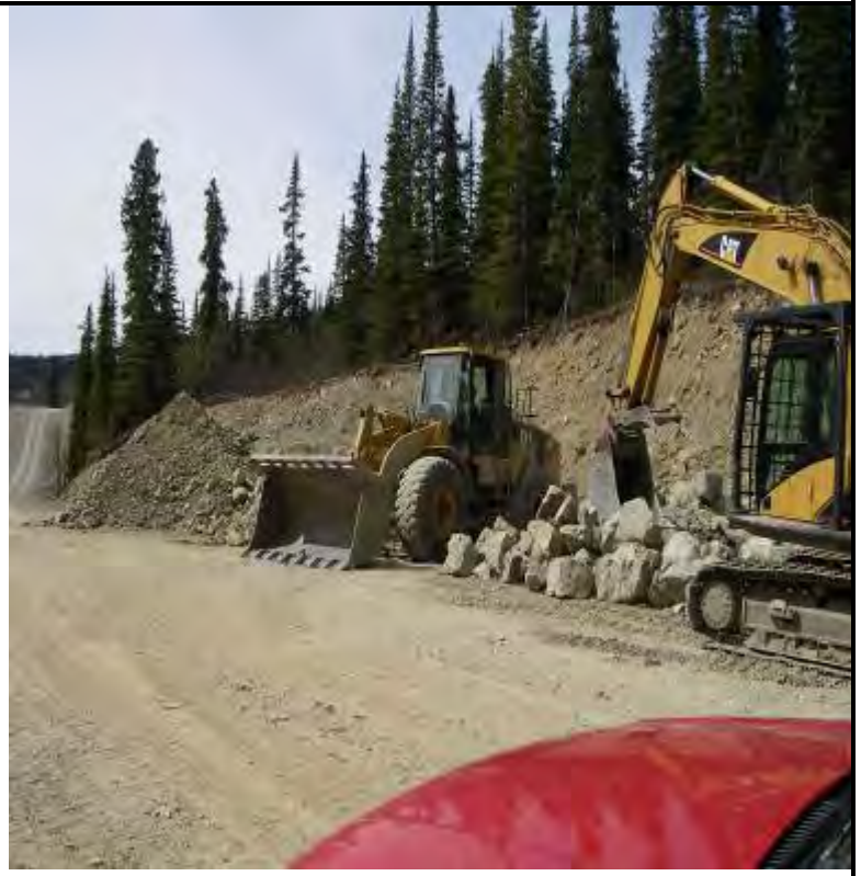
Km 14 – Gathering/sorting material for km 9 repair
