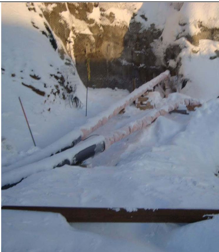
12-13-08 Steel to HDPE connections at Portal adit above the multiplate (facing E)
