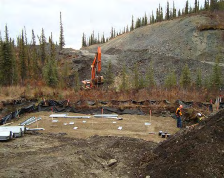
Bunker Creek: down chain bin wall layout. 09_25_08 (facing upchain (UC))
