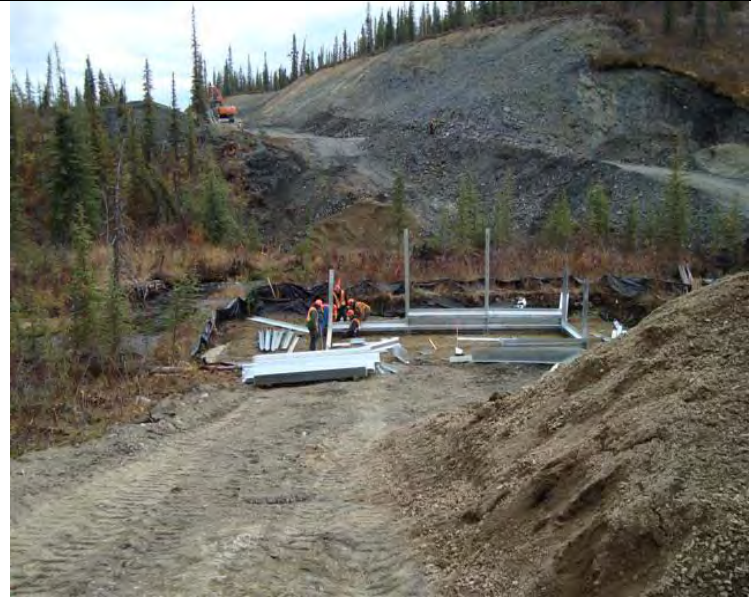
Bunker Creek: down chain bin wall establishment. 09_25_08 (facing UC)
