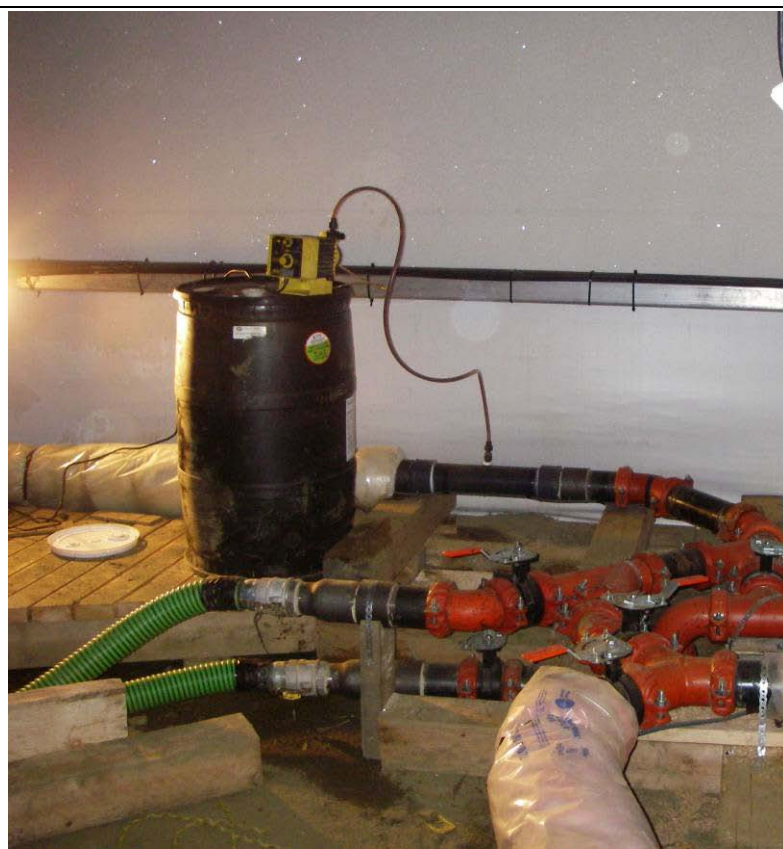
12-20-08 Header install with hoses attached and ferric injector installed
