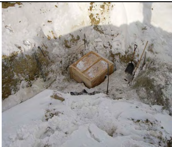
11-07-08 Forming of the thrust blocks for the buried services
