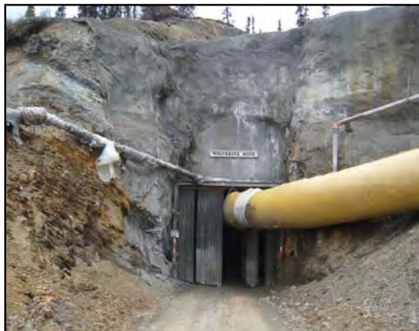
Picture 4-2: View of the rockfall area (left side of portal) after scaling, 6/06/08.
