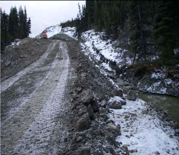
10_13_08 Facing UC @ km 15+200 looking at cutslope ditchpool was dredged out to improve settlement before culvert inlet
