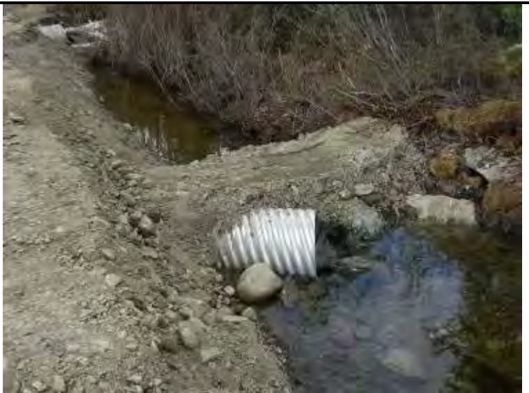
Hawkowl Creek – 24” culvert with ditch plug
