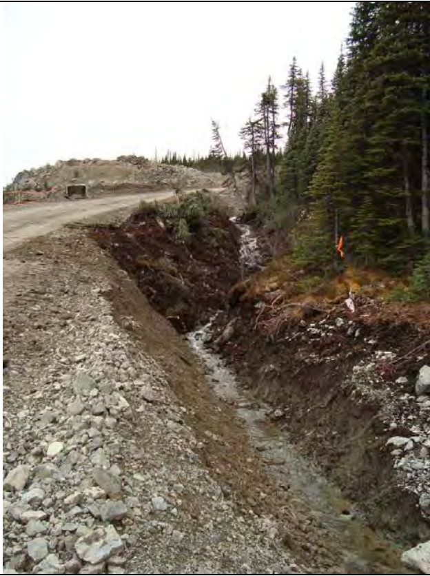
09_28_08 Deeper ditching upslope to intercept surface flow (facing UC)
