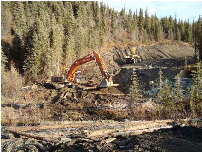
10_06_08 Facing DC, pulling abutments apart. Area needs to be filled, sloped. Rip rap to be continued from bin wall around base of slope. Ditching to continue on left hand side of road down along tree line (approx.). Silt fence to be continued where abutments have been removed.
