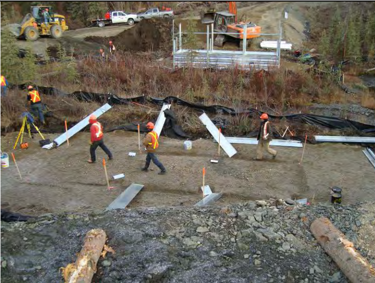
09_27_08 Up chain bin wall layout (facing DC)
