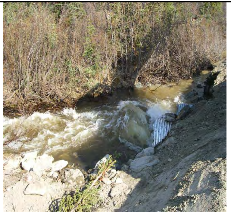
Photo 2 - 05/27/08 - Placing Culvert 24” to handle ditch flow
