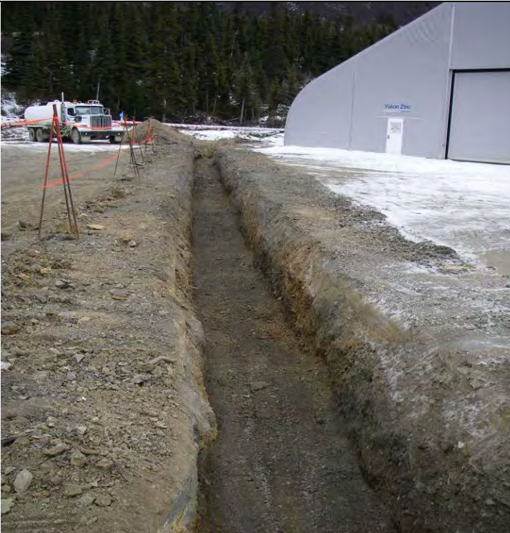
10_15_08 Trench at lower portal to accept the new pipeline
