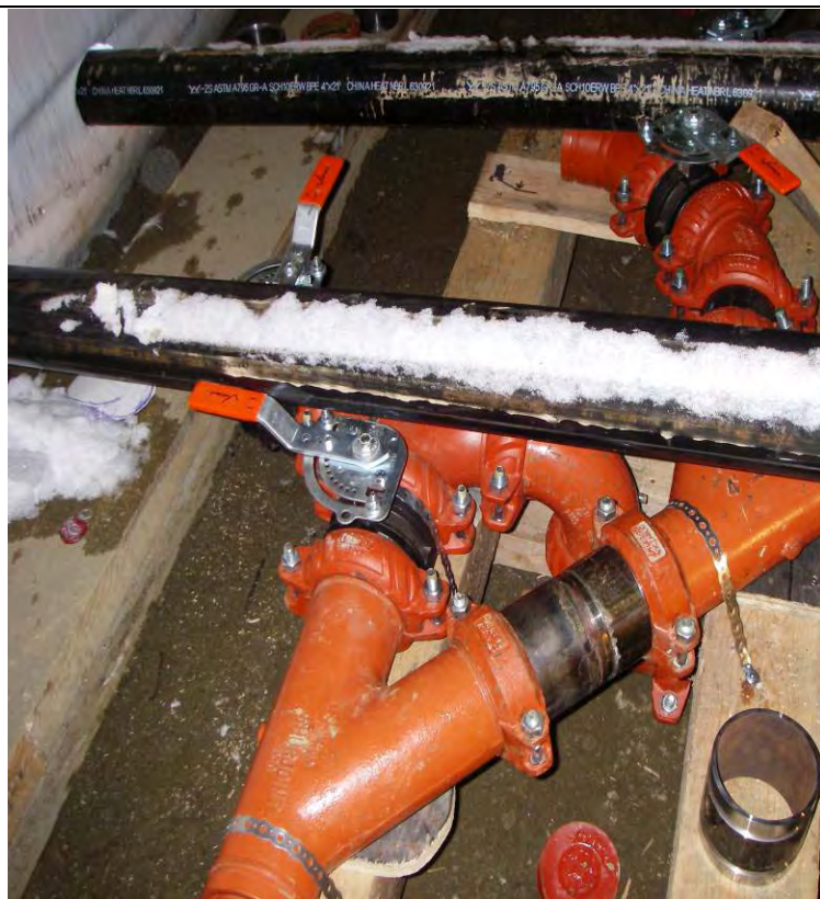
12-05-08 Header Install and pipe penetration on East side of building
