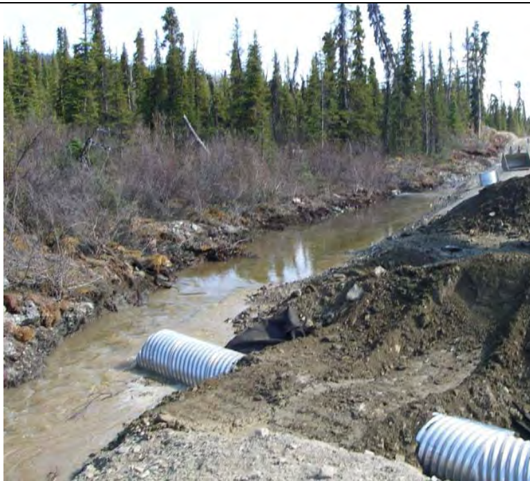
Photo 2 - 05/27/08 - Placing Culvert 24” to handle ditch flow
