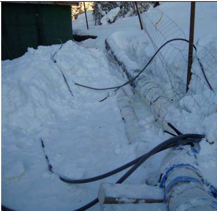
12-13-08 HDPE to Steel connection at Lower Portal (facing NE)
