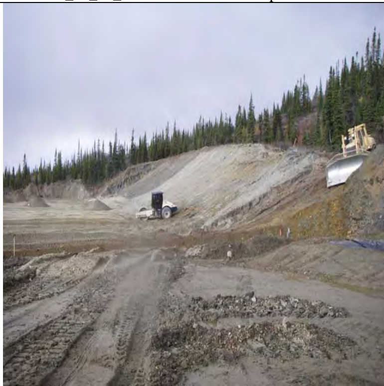
PortalPad_09_17_08 Compacting the Portal Pad
