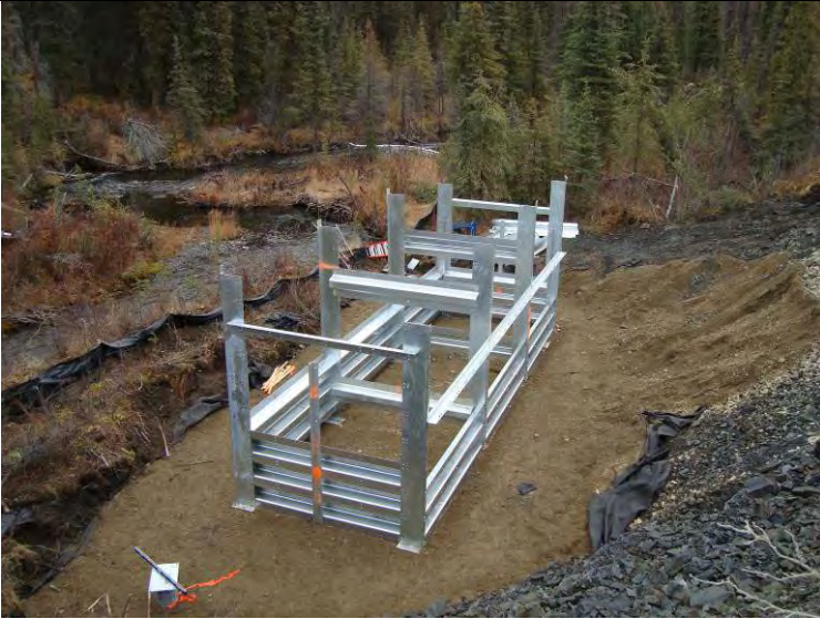
09_29_08 Up chain bin wall layout and construction (facing downstream)
