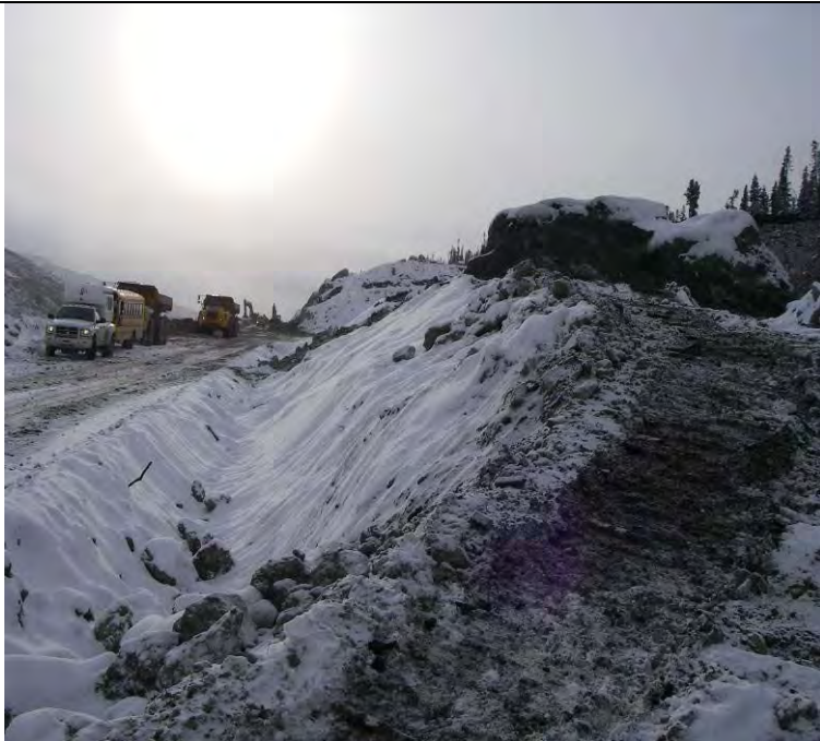
10_19_08 Looking DC at km15+100 cutting down the permanent ditch to capture groundwater seepage
