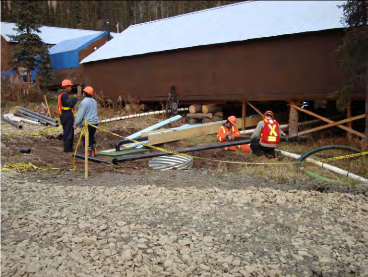
09_27_08 Insulating and heat tracing discharge lines
