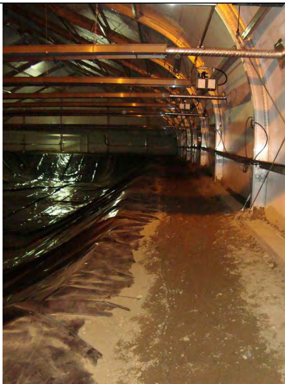
12-01-08 Filled in lock trench
