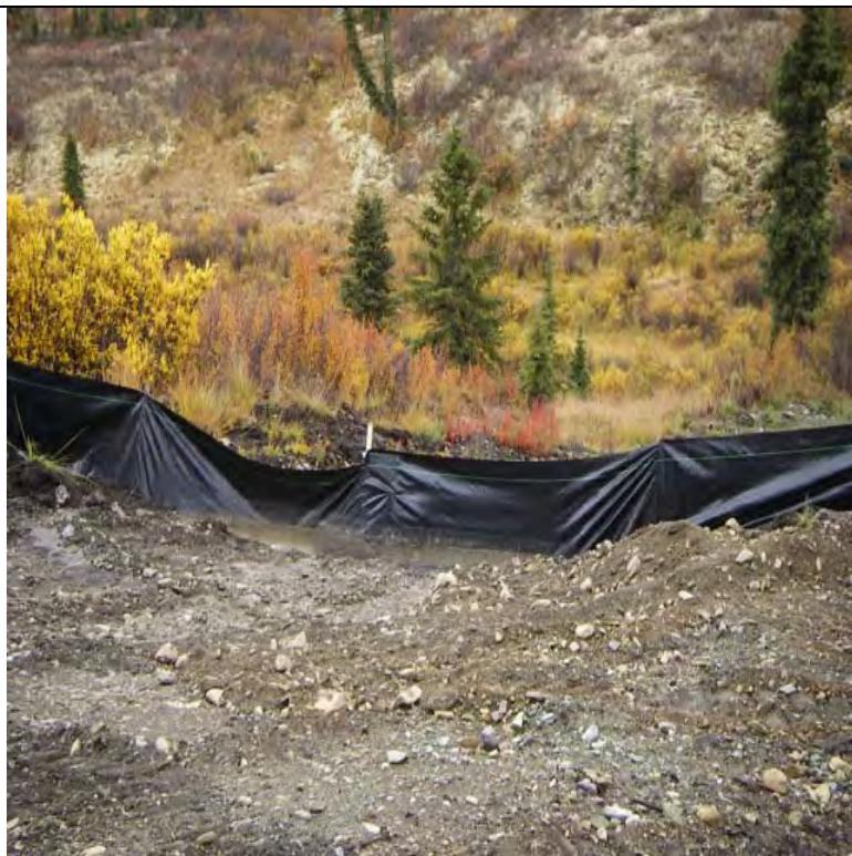
PortalPad_09_10_08 Silt Fence at toe of pad
