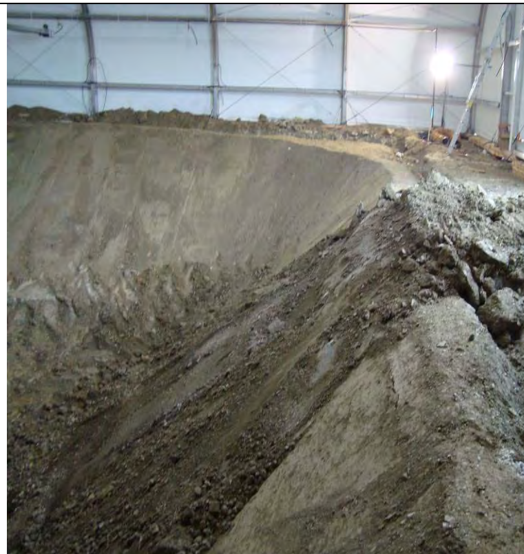
11-14-08 Excavation of the 2000 m 3 sump pulling the ramp - facing E
