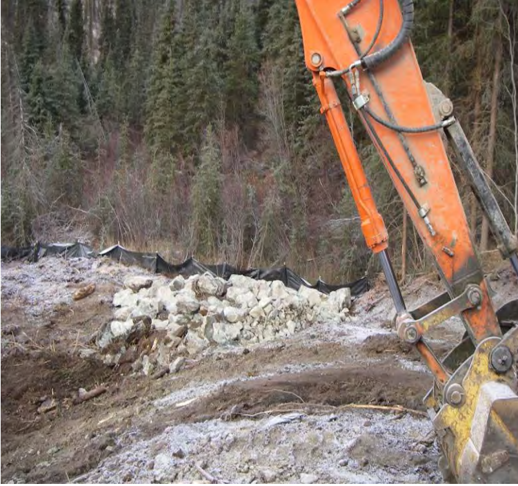
10_08_08 Facing UC, preparing ditch grade and energy dissipater on u/s DC side of bridge
