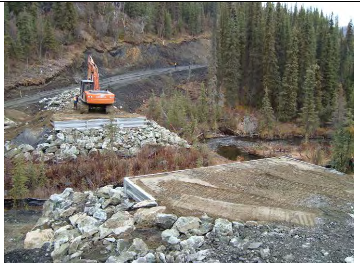
10_02_08 Facing DC, bin walls complete, geotech wrapped around backfilling followed by rip rap placement.
