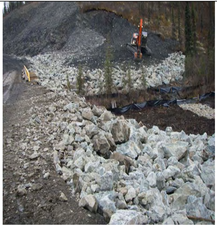
10_13_08 Facing UC, armouring on UC u/s bank completed rock lined ditch
