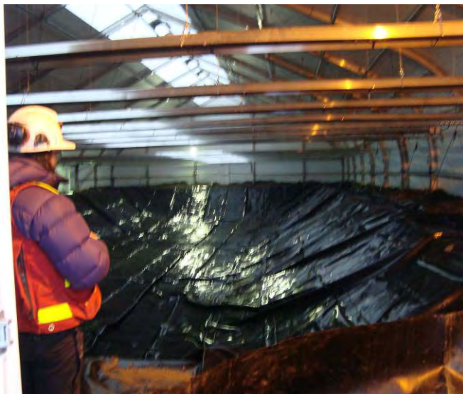
11-23-08 Finished liner install, still requires backfilling of lock trench
