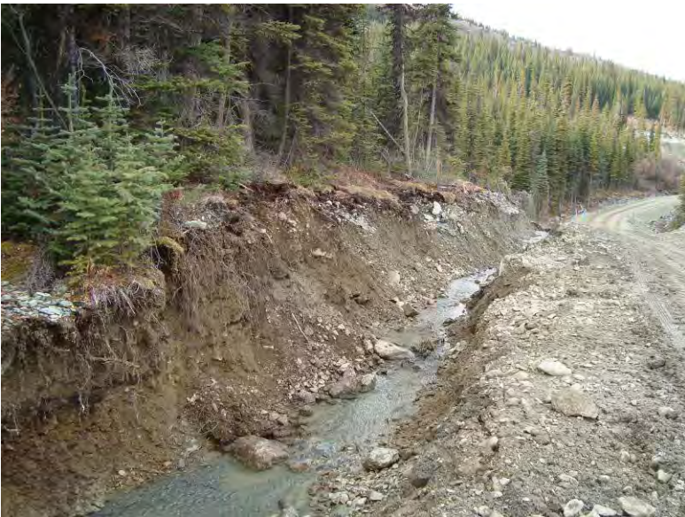
10_02_08 Water running clearer after ditching the previous day (Facing DC)
