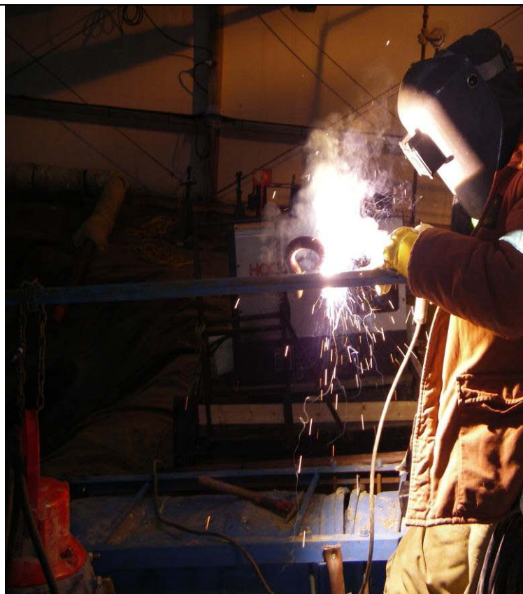
12-15-08 08 Raft Modifications using tubular steel and rubber drill hose
