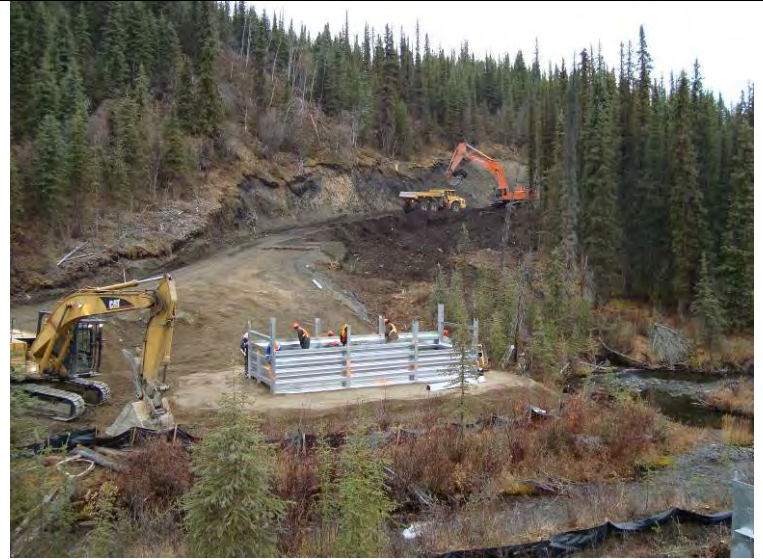
09_29_08 Down chain bin wall installation, backfilling and loading (facing downchain (DC))
