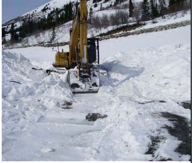
04/24/08 WRP snow clearing for berm placement
