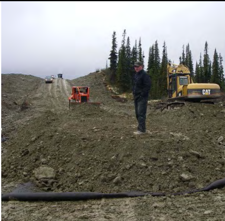
06/08/08 –Facing NW 2 nd layer of geotextile and fill
