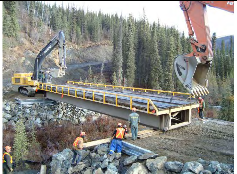
10_03_08 Facing DS, sliding boards under bridge for extra support.
