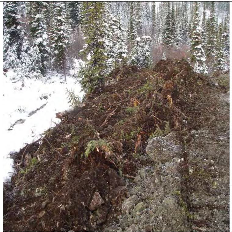
10_19_08 Looking DC at km 15+200 Organics windrowed above the diversion
