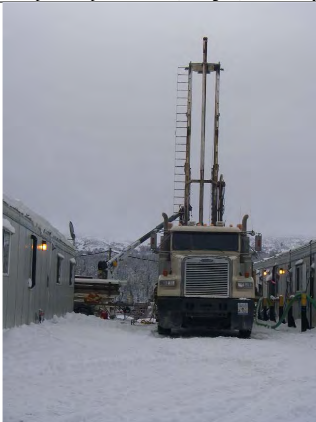
11-03-08 Drilling of the potable water well – facing W
