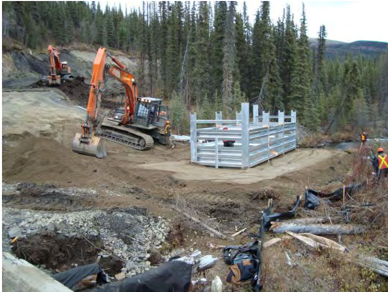
09_28_08 Down chain bin wall backfill and compaction in foreground, down chain approach work in background (facing DC)
