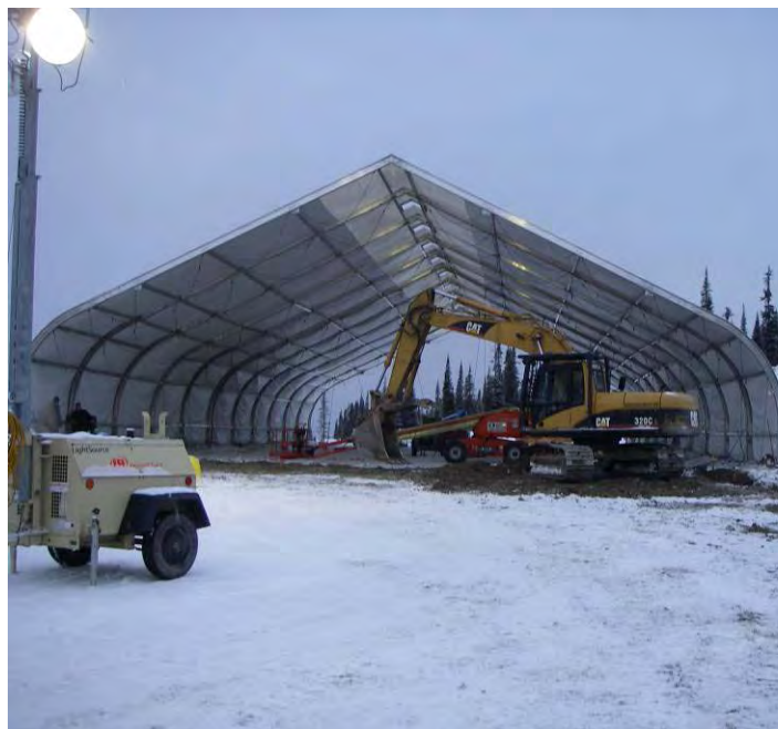
10-29-08 Installation of the side panels in background, digging of the propane pipeline trench in foreground (with hoe) – facing NNW
