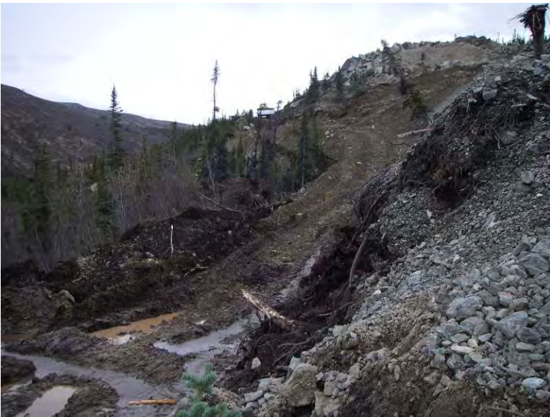
09_27_08 Down slope cut, Trough cut to minimize sediment loading (Facing UC)
