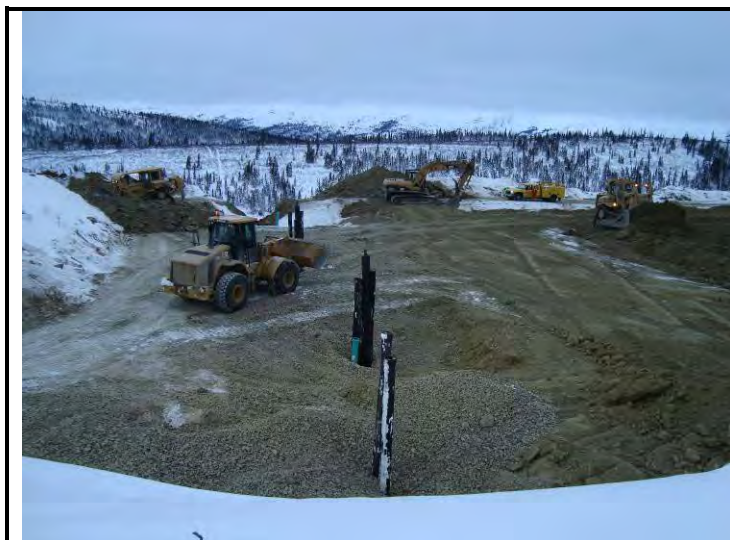
12-06-08 Backfilling around raises (facing W)
