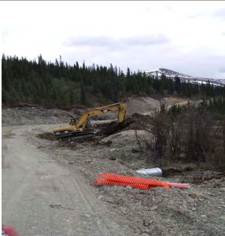
06/06/08 - Facing SE – clearing area to straighten road
