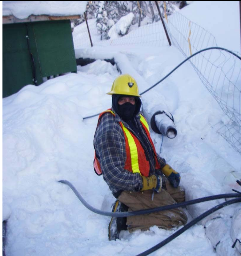
12-13-08 HDPE to Steel tie in at Lower Portal u/s of pump shack ( facing NE)
