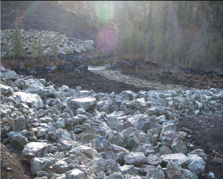
10_09_08 Facing DC, finishing the armouring and energy dissipater and prepping for the outflow path of the ditch to creek
