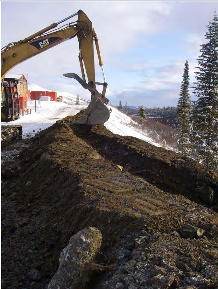
10_18_08 Looking South,Saddle for pipeline on berm outside Procon's shop
