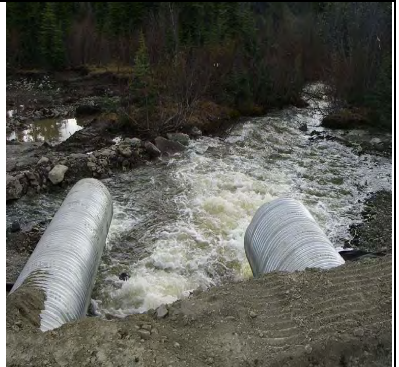
Photo 8 - 05/28/08 – 36" overflow installed, and flows peaking, some armouring added looking d/s
