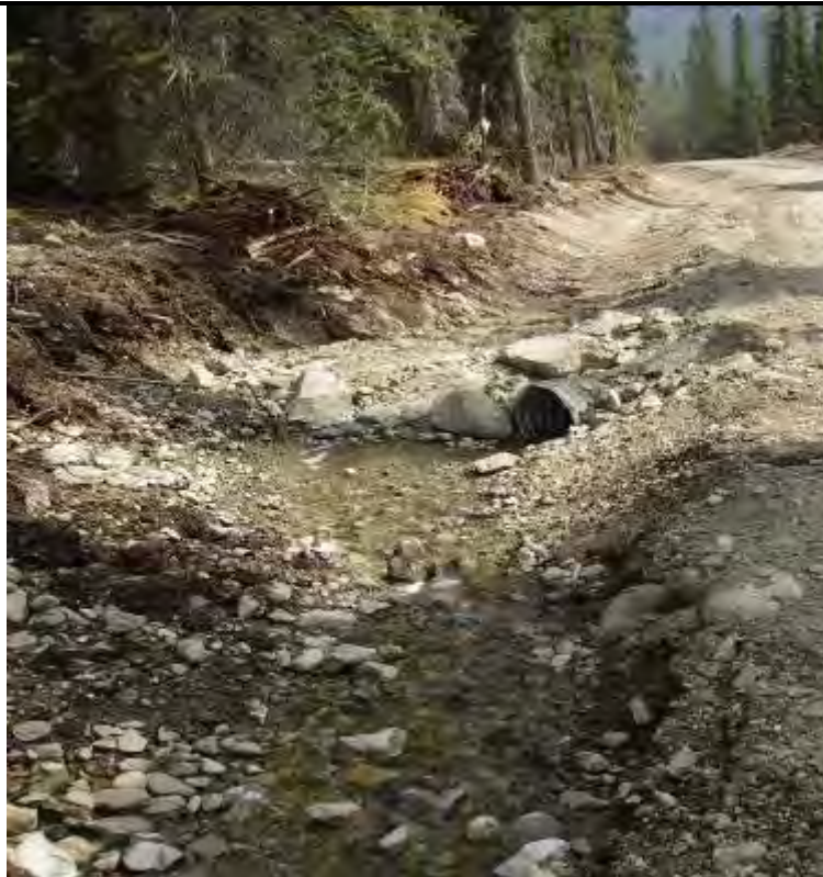
Km 12.5 – Culvert with ditch block ( to mitigate km 12)
