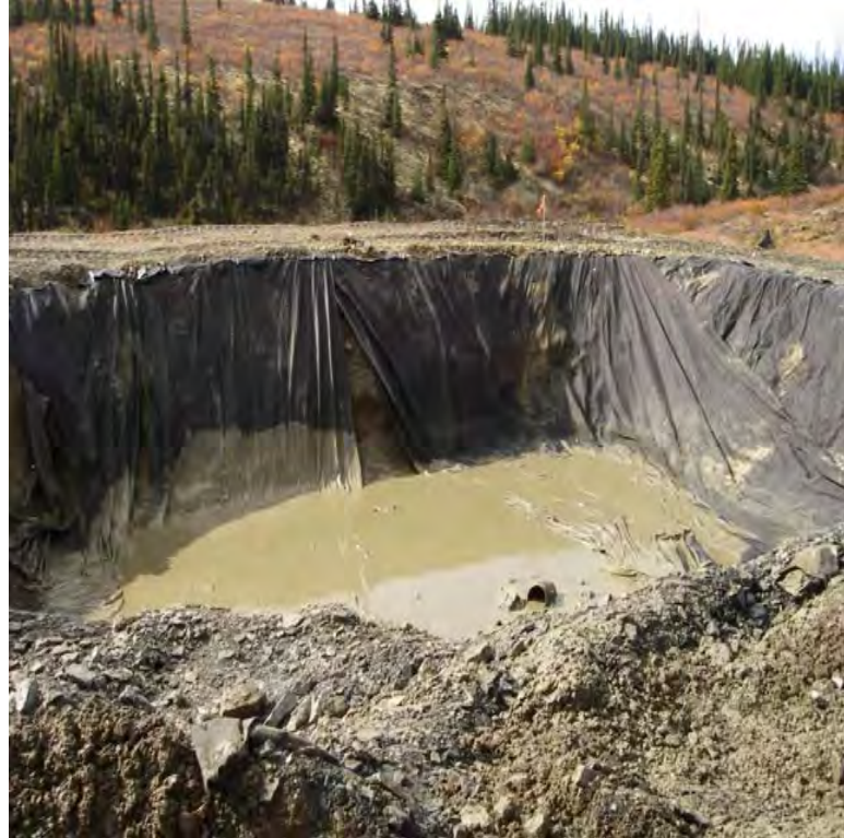
PortalPad_09_09_08 Decommissioning PCS preparing to pump water to WRP before liner removal
