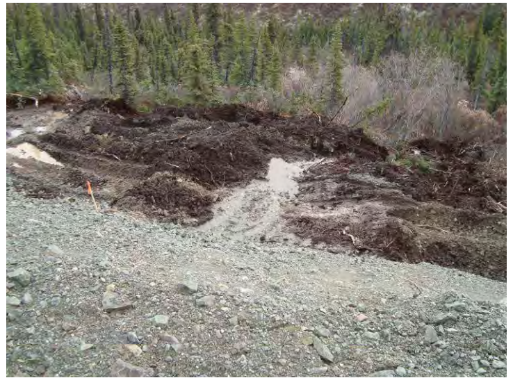
09_28_08 Water running under road before upslope ditch improvements
