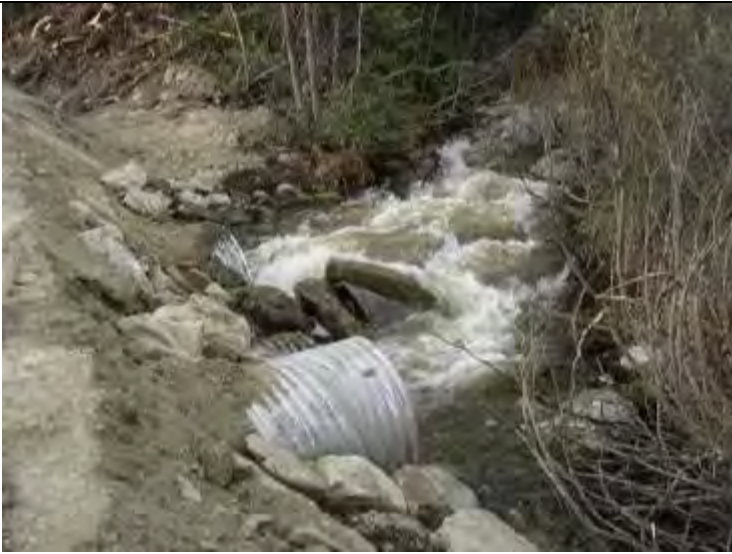
Hawkowl Creek – main stream following 36” overflow culvert installation and cobbling of stream
