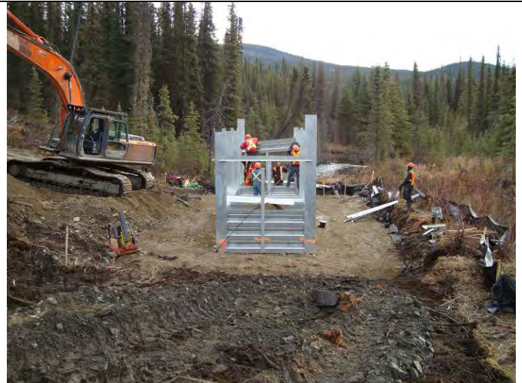
09_27_08 Down chain bin wall installation (facing downstream )
