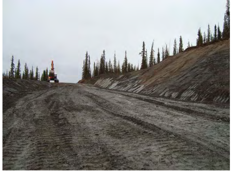
10_05_08 Facing UC, road re-contoured and re-sloped. Cross drain needs to be installed from slope through bank.
