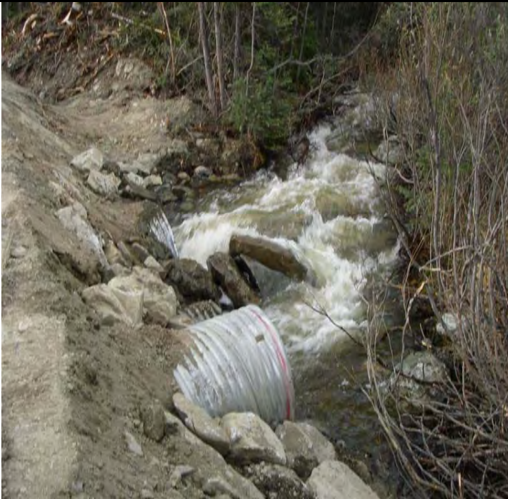
Photo 7 - 05/28/08 – 36" overflow installed, and flows peaking, some armouring added looking u/s
