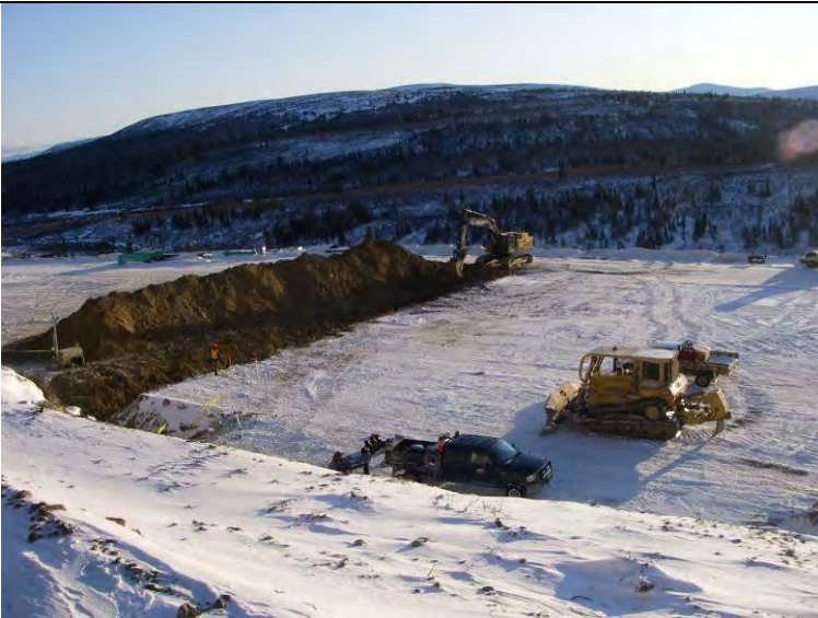
10_23_08 Stockpiling fill material for excavations (facing southwest)
