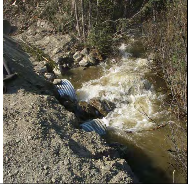
Photo 6 - 05/27/08 - Placing Cobble to align stream to 48" culvert complete, headwall protected. Looking u/s
