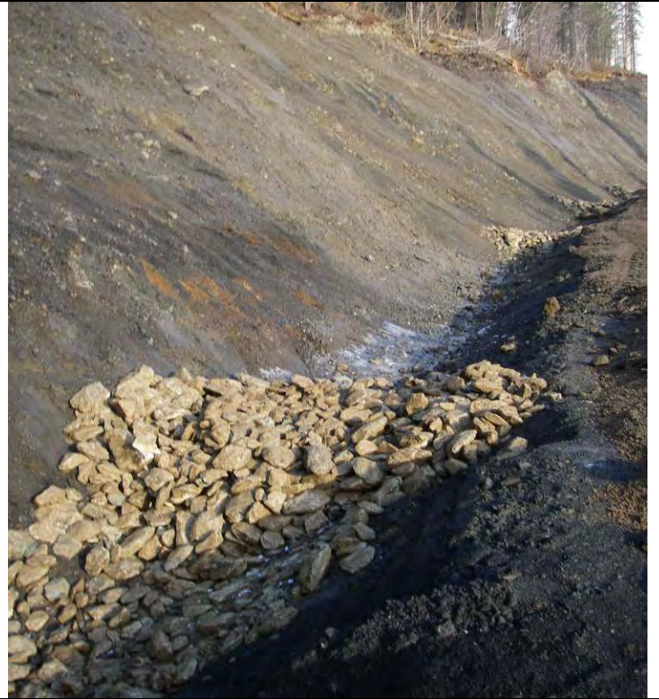
10_11_08 Facing DC, Ditch blocks and start of rock lined ditch on u/s DC side
