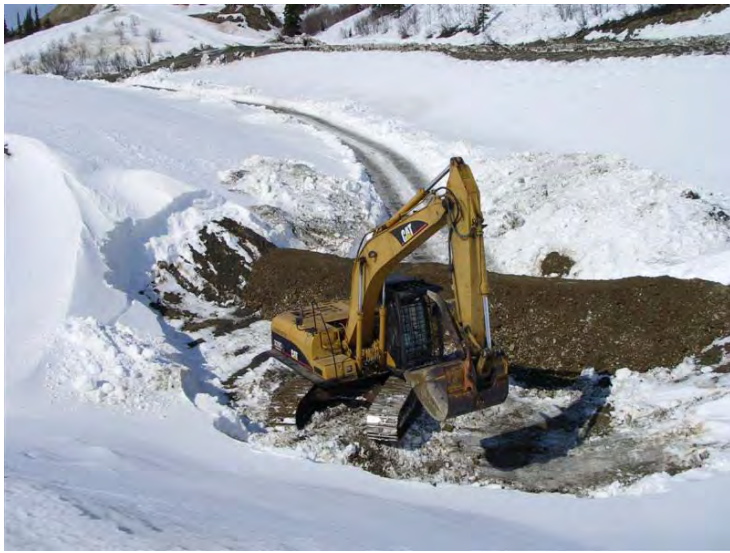
04/24/08 WRP berm being compacted and shaped
