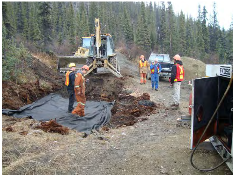
10/03/08 Geotextile over permafrost that was found (facing SE)
