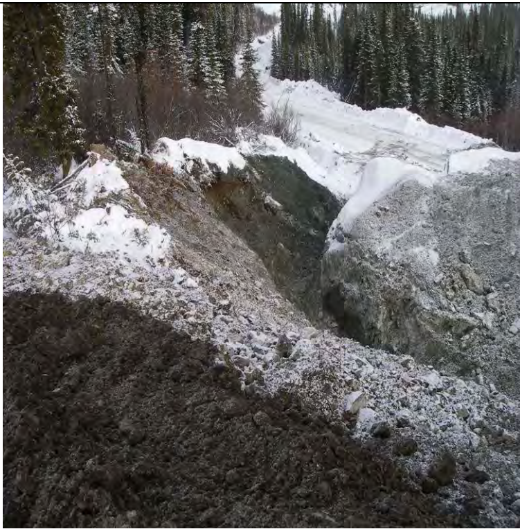
10_19_08 Looking DC at km15+100 cutting down the permanent ditch to capture groundwater seepage
