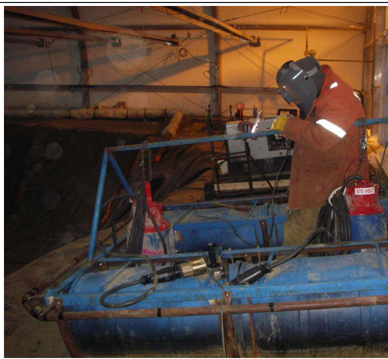
12-14-08 Raft Modifications using tubular steel and rubber drill hose
