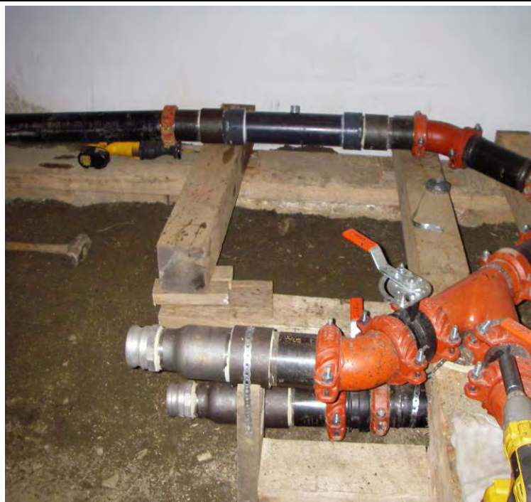
12-07-08 Header Install with Ferric Injection Splice
