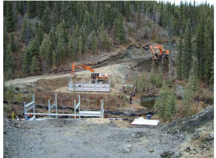
09_28_08 Down chain bin wall backfill and compaction in foreground, down chain approach work in background (facing DC)
