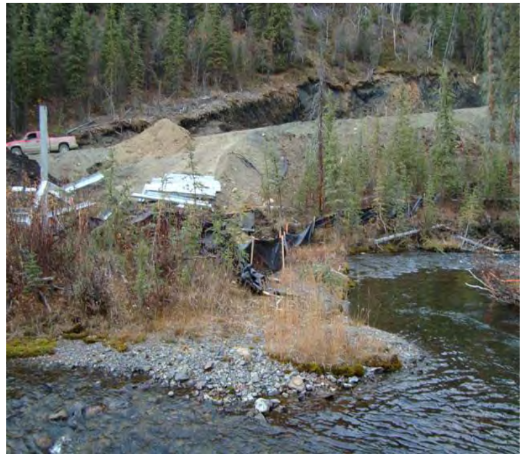
Bunker Creek: Silt fencing re-installed. 09_26_08 (facing DC)
