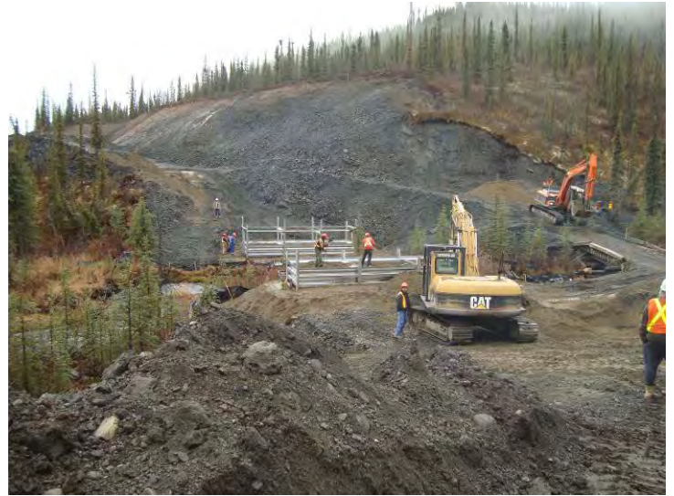
09_30_08 Loading and backfilling of bin walls (facing UC)
