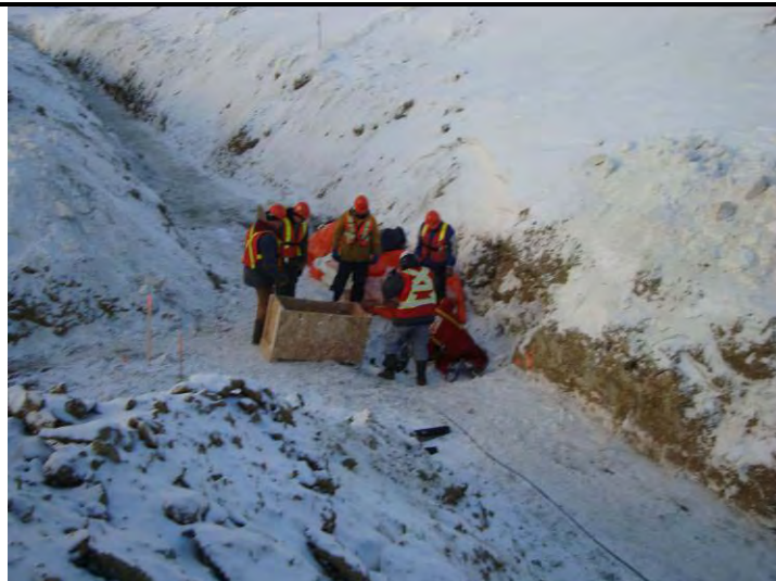
11-22-08 Filling thrust blocks with cement
