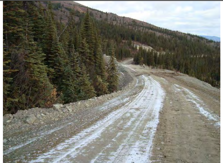
09_27_08 Upslope ditching not done, water draining underground (facing DC)
