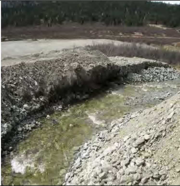
Go Creek Airstrip – culverts pulled looking d/s ( more rip/rap and cobble needed on outside turn of bank)
