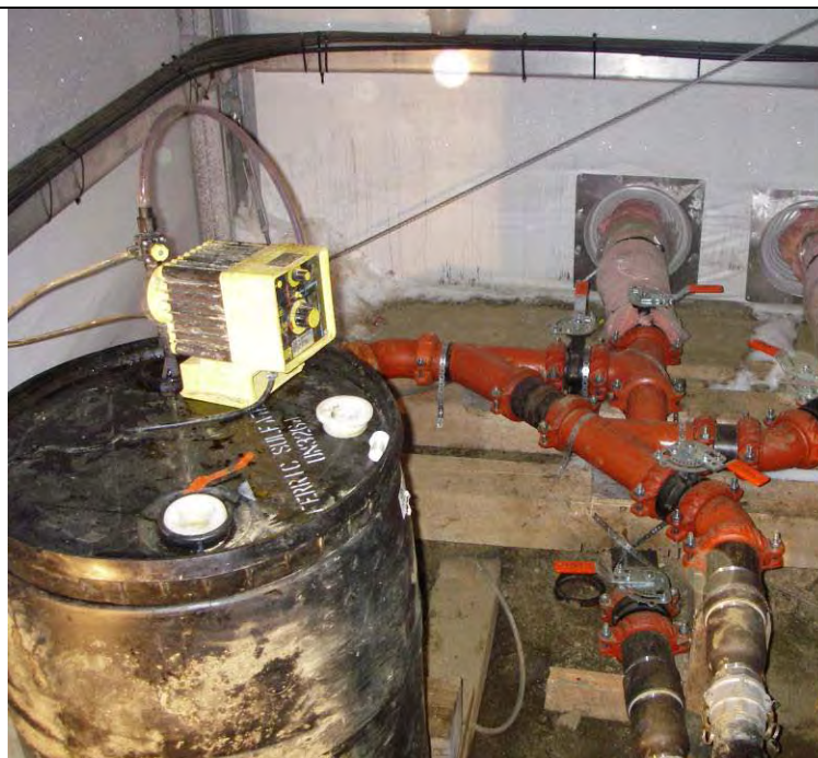
12-20-08 Header install with hoses attached and ferric injector installed
