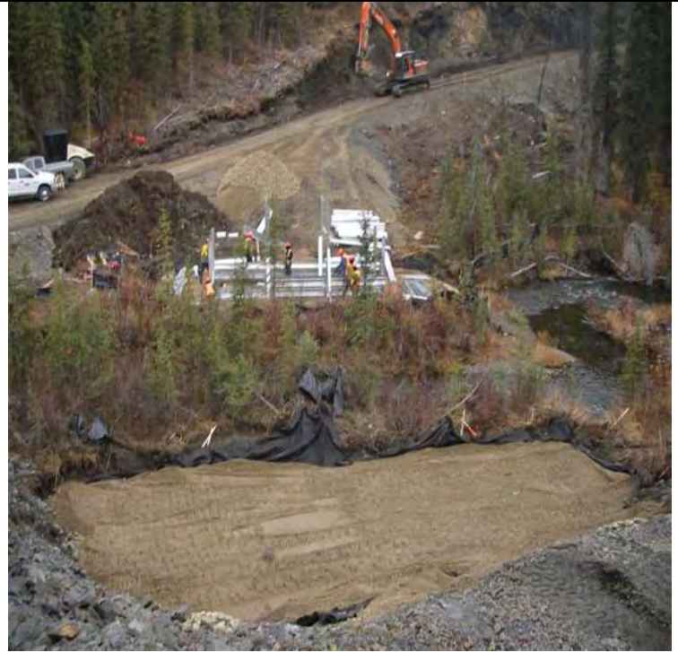
Bunker Creek: 09_26_08 Site over view. Ground prep work for UC bin wall. (Note: silt fence installed later.)
