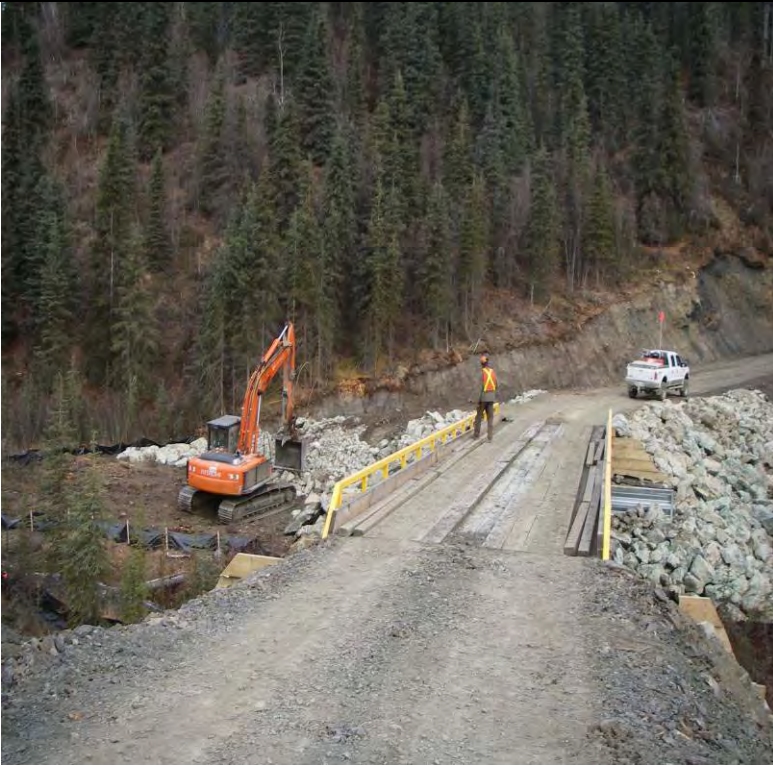
10_09_08 Facing DC, finishing the armouring and energy dissipater and prepping for the outflow path of the ditch to creek
