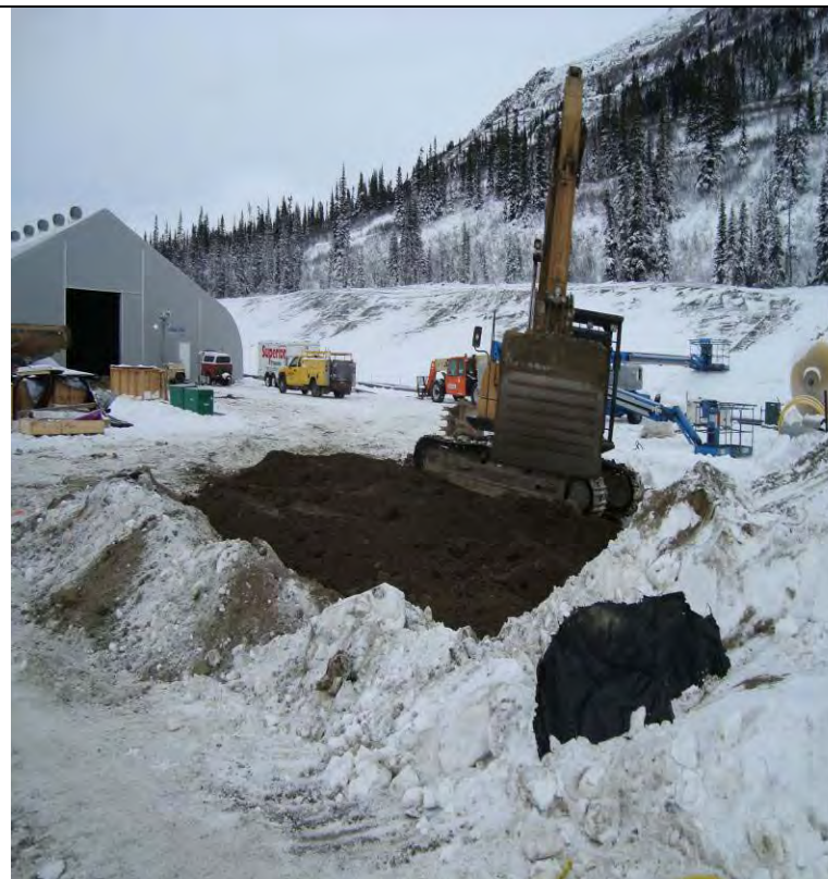
11-14-08 Backfilling the temporary sump – facing N
