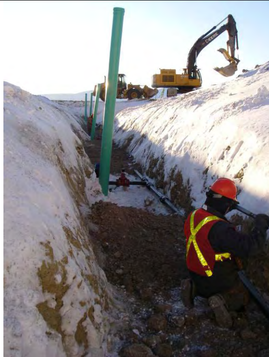
12-02-08 Pipe laying in trenches
