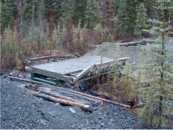
10_05_08 Facing DC, temporary bridge cleaned of debris, both backs with sediment pulled back from abutments and area prepped for bridge removal.
