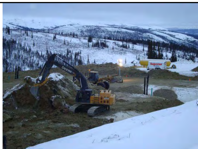
12-06- Backfilling around raises (facing NW)
