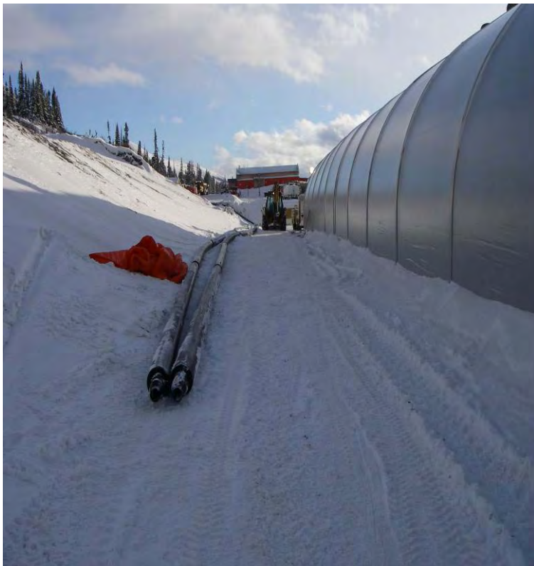
11-07-08 6" HDPE being run behind the new Sprung-facing S
