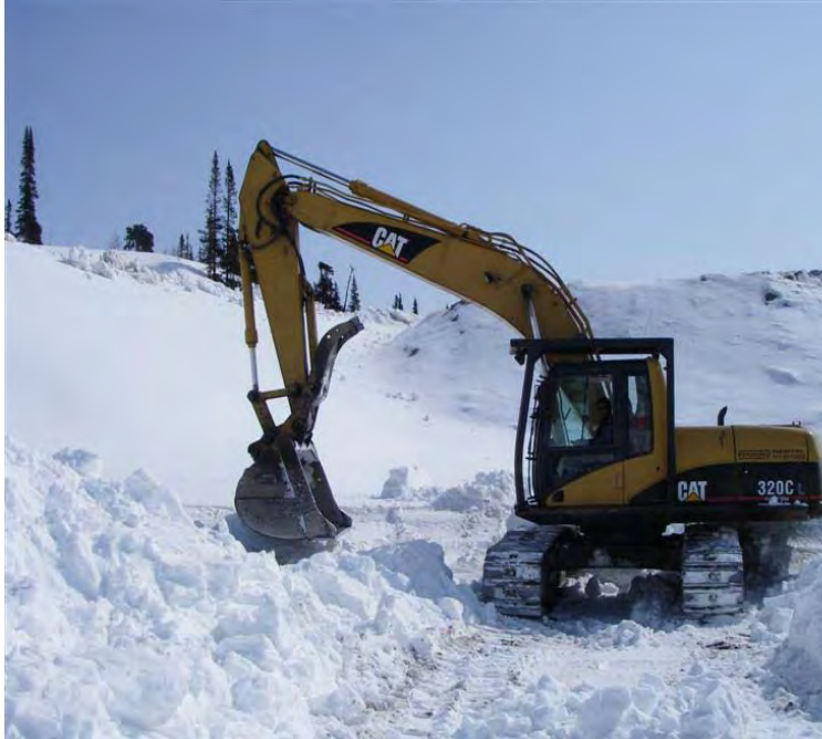
04/24/08 WRP snow clearing for berm placement
