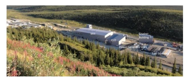
Picture 2-1: Overview of industrial complex area including camp, mill, concentrate load-out (CLO), crusher buildings, as well as power generator area and fuel storage areas.
