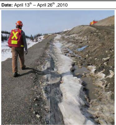
10/04/15 Ice built up along the ditch blocking flow
