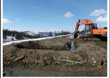
10/04/22 A sump has been built to collect water pooling above ditch 4. This water is then pumped into ditch 4 or taken via truck to tailings facility
