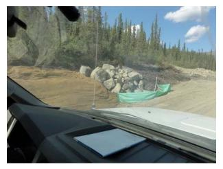
Picture 8-6: Coconut matting, rip rap, and silt fence (temporary) at culvert inlet.
