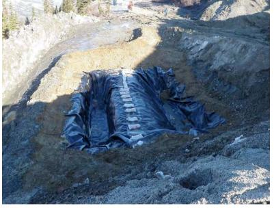
10/04/24 Sump built below north end of ditch 4 to catch runoff from dynamic waste rock pile. This water will then be pumped into ditch 4 or to tailings
