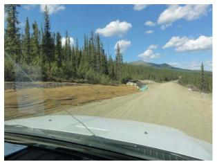
Picture 8-5: Coconut matting and seeding at erodible area draining to a newly installed culvert.
