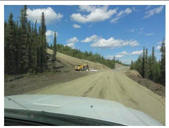
Picture 8-7: Grading of borrow pit and placement of organic material along road corridor.
