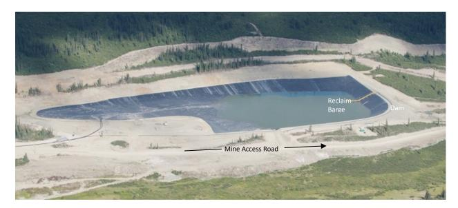
Picture 2-4: Tailings storage facility and mine access road.
