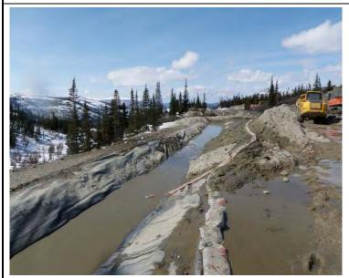
**10/04/18** Water is flowing at a steady pace. No more ice and debris damming it up. There is a lot of sediment building up that needs to be removed.
