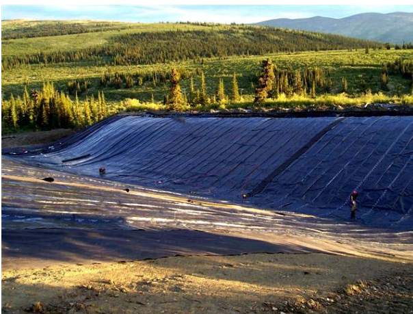
Picture 8-3 Completion of Enviro Liner® Installation
