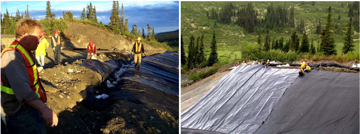
Picture 8-2 Installation of the Geotextile Layer and Enviro Liner®
