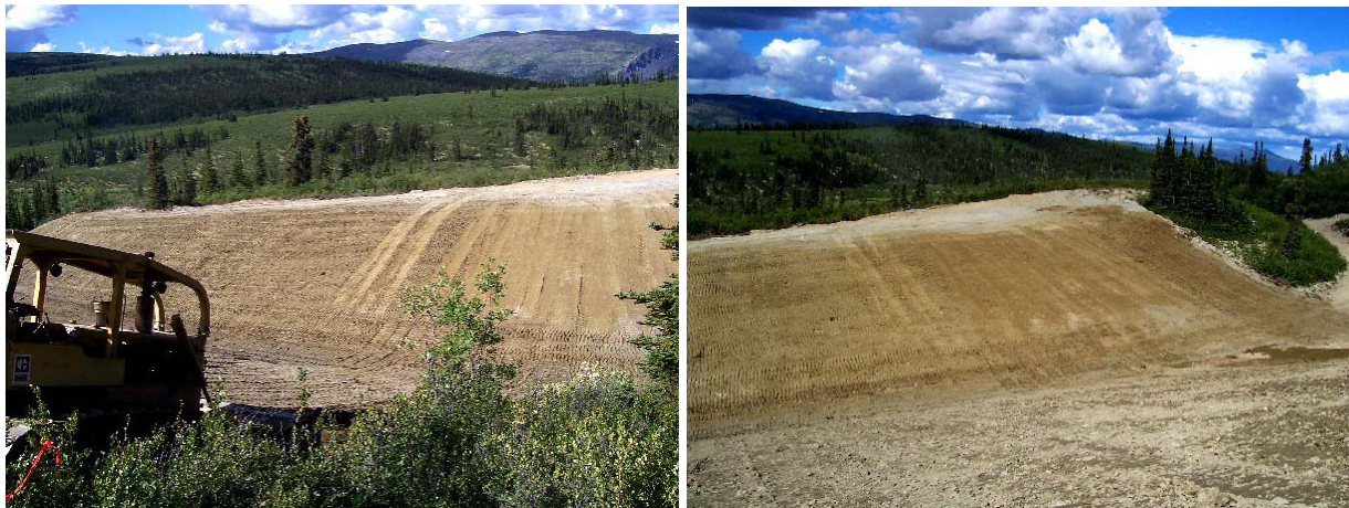
Picture 8-1 Grading, Contouring and Proof-Rolling the Till-Like Surface
