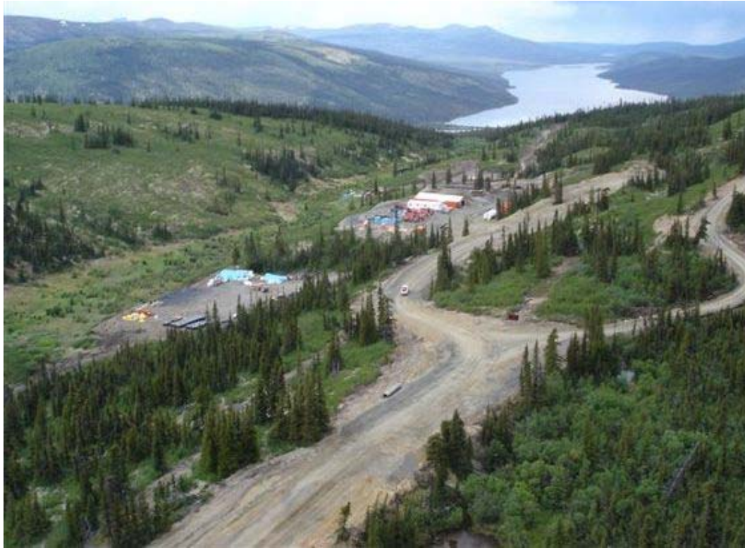
Figure 1 Looking Northwest from the Mine Site Across the Broad Wolverine Lake Valley
