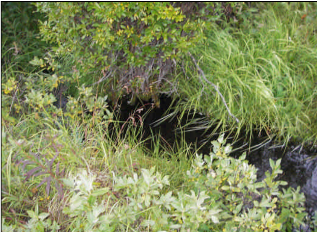
Photo 66: Site 14 looking downstream on August 7, 2005.
