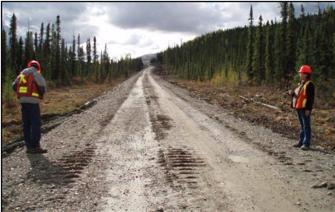
Picture 1: Access Road at km 3, Looking South Towards the Mine Site.
