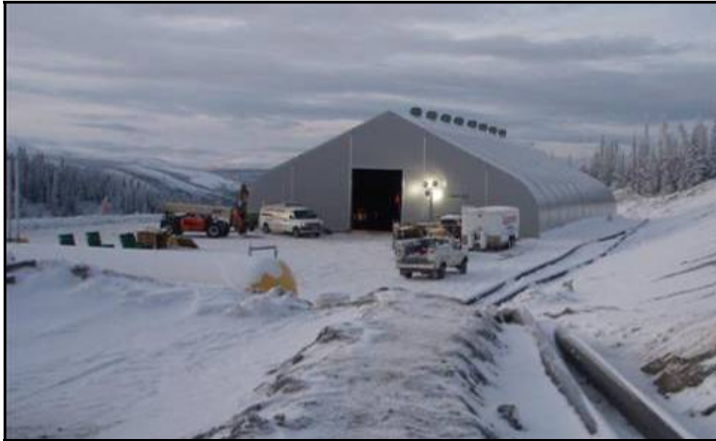
Picture 4: Underground Dewatering/Settling Sump #3 Located Near the Portal.
