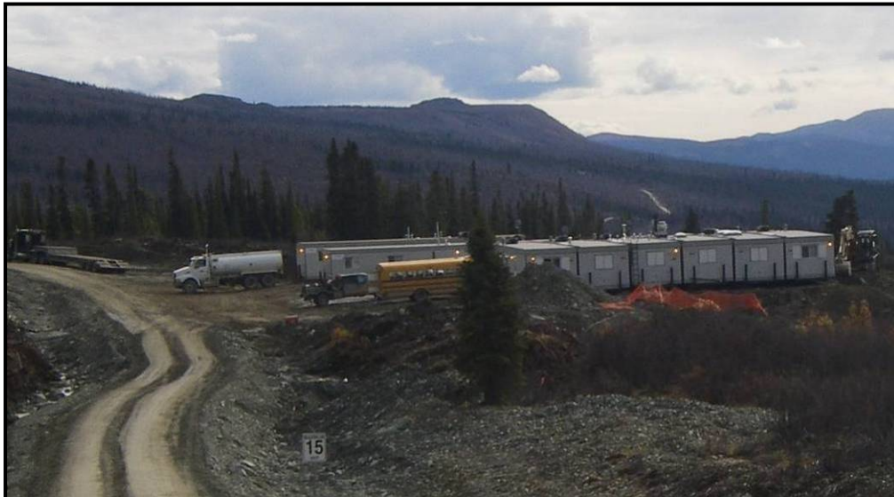
Picture 5: Temporary construction camp situated north of the tailings facility.
