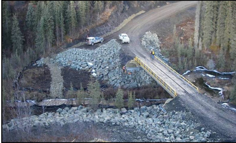
Picture 3: Bunker Creek Permanent Bridge.
