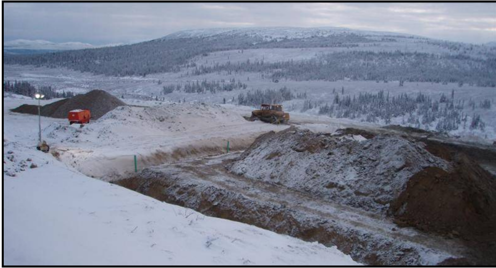
Picture 6: Installation of the underground utilities for the permanent camp.
