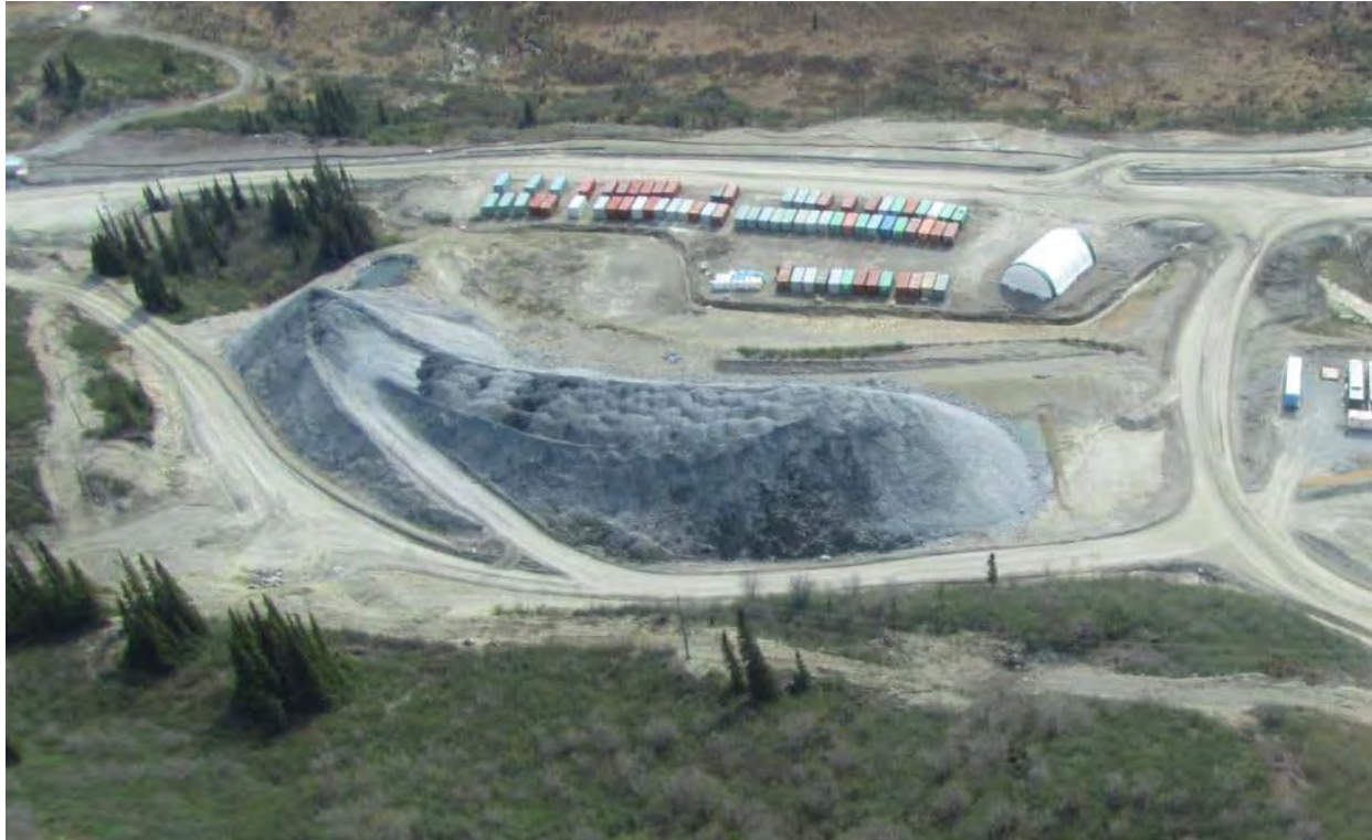
Picture 2-3: Temporary Waste Rock and Ore Storage Facility (taken June 1, 2011)
