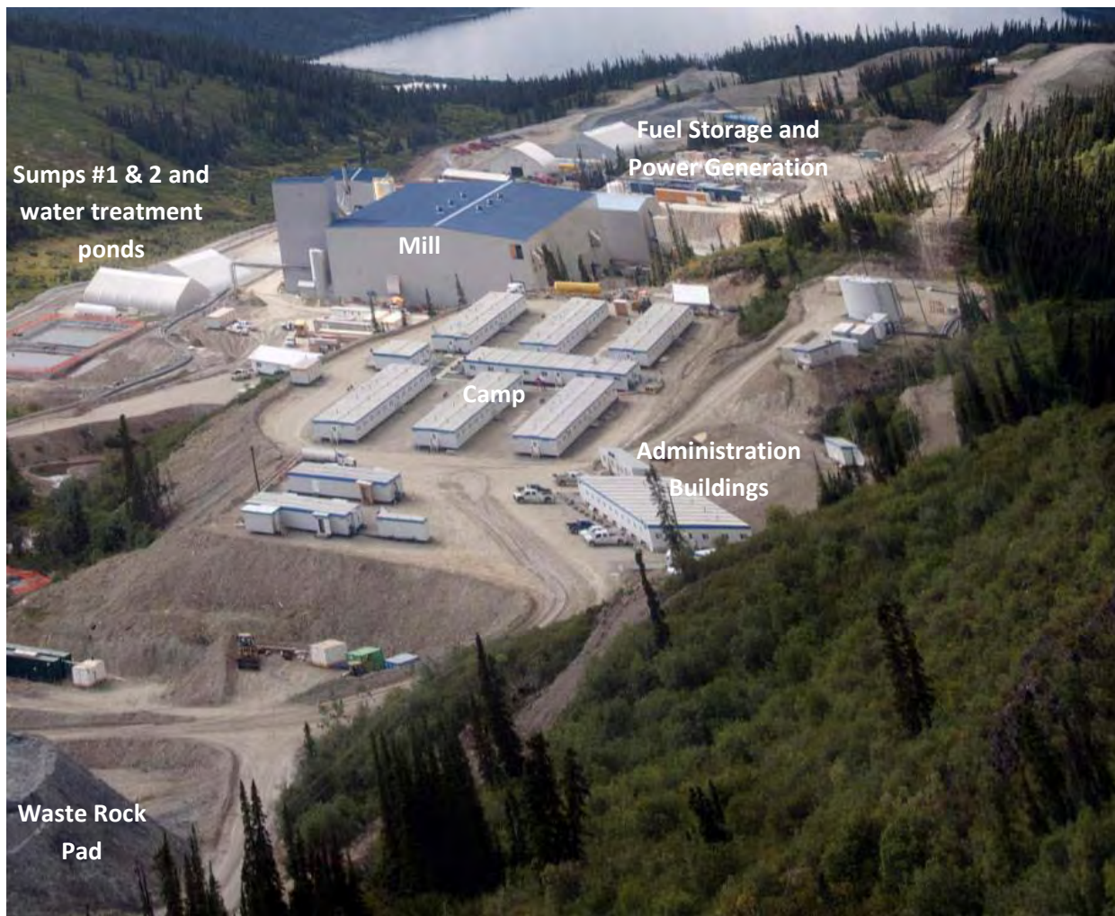
Picture 2-1: Surface Infrastructure within the Industrial Complex (August 10, 2010)
