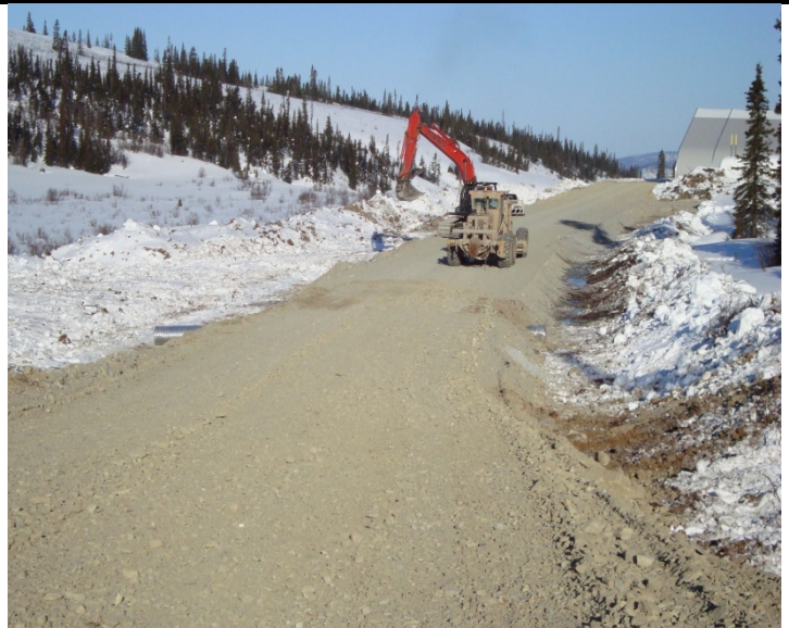
04_03_09 Excavator is ditching and grader making a pass over on the road. Photo taken looking U/C towards Sump#1. Culvert in place at the low point.
