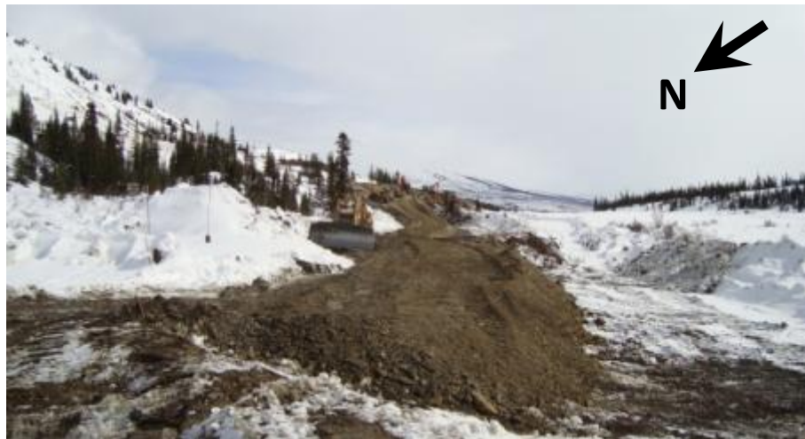
Picture 2. Road Bed Fill and Compaction of Mill Bypass Road (April 1, 2009)
