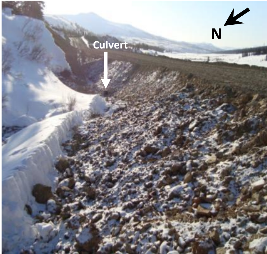
Picture 3. Completed Mill Bypass Road (April 3, 2009)
