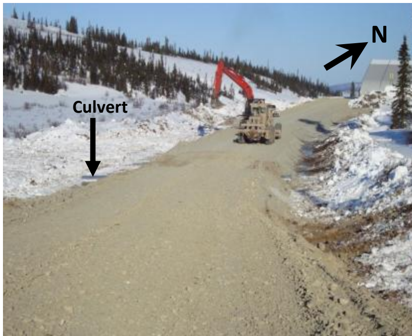
Picture 4. Completed Mill Bypass Road (April 3, 2009)
