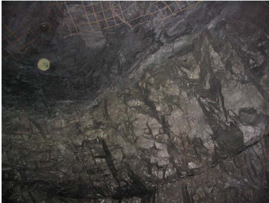
Photograph 23: Location 7 View of the exposed HW in Argillite.
