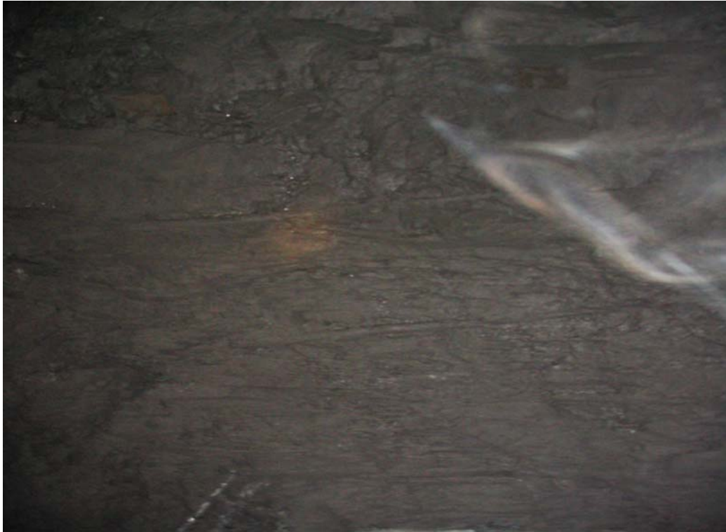
Photograph 15: Location 5 View of Shotcreted wall and back
