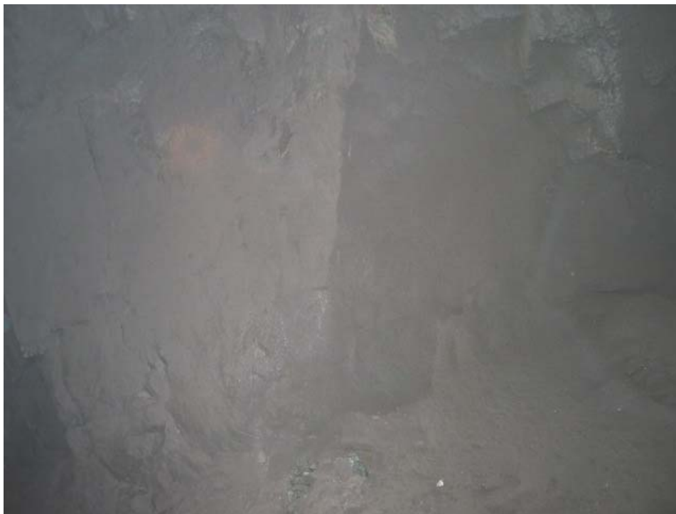
Photograph 30 View of the pillar between the herringbone panels
