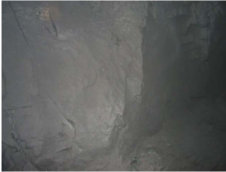
Photograph 31 View of the pillar between the herringbone panels
