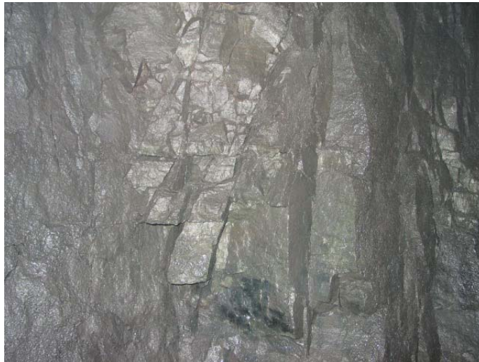
Photograph 26: Location 8 View of the wall in the ore zone
