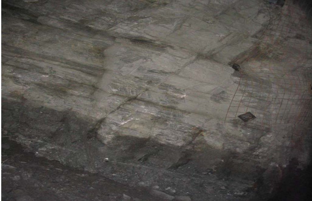
Photograph 9: Location 3 View of the wall in EXCP
