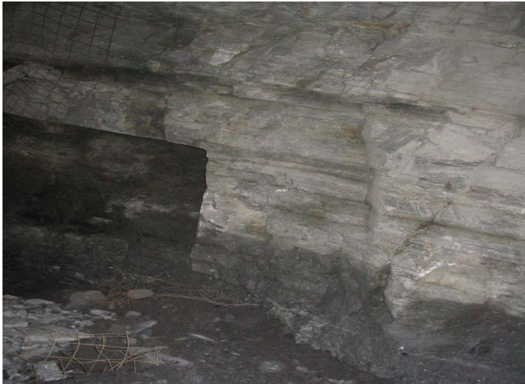
Photograph 10: Location 3 View of the wall in EXCP
