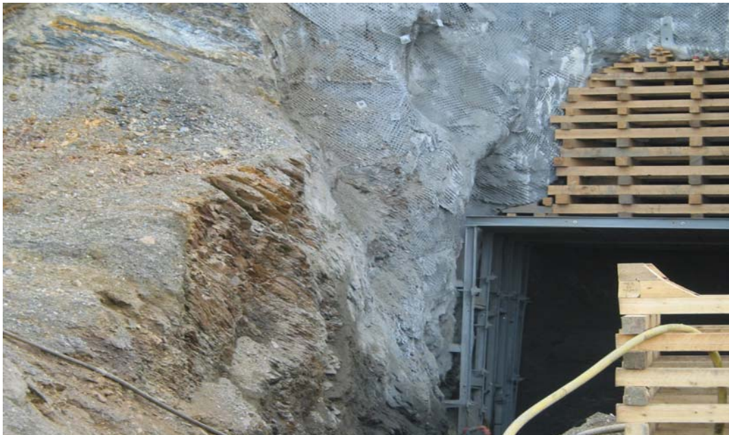
Photograph 2: Location 1 View of portal and square steel set at the portal
