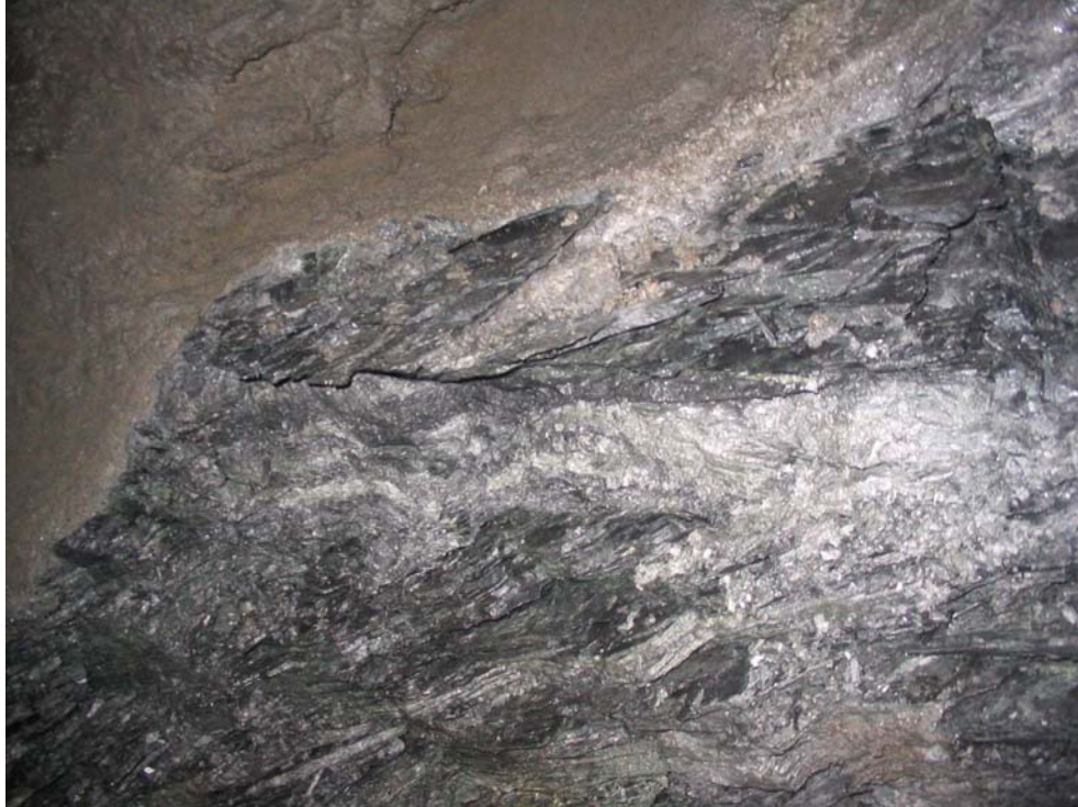
Photograph 11: Location 4 View of the Shotcreted back in Argillite
