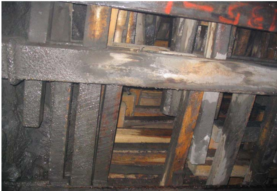
Photograph 12: Location 4 View of the timber set support in the argillitic back
