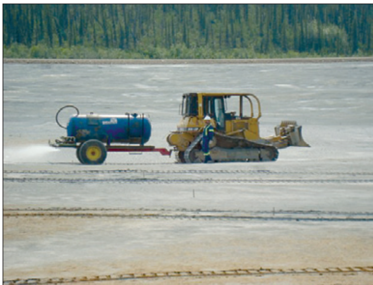
Faro Mine Complex — to reduce risk of contaminants being released into the environment, a product called Soil-Sement is sprayed on to the trailing at Faro to reduce dust in the air.
