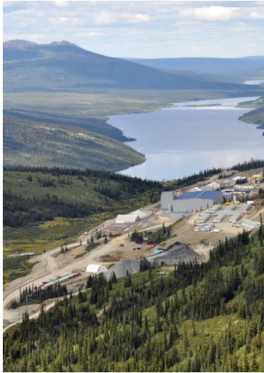
The Wolverine mine site. We're looking at ways to reduce mining's negative socio-economic impacts and increase its benefits.
