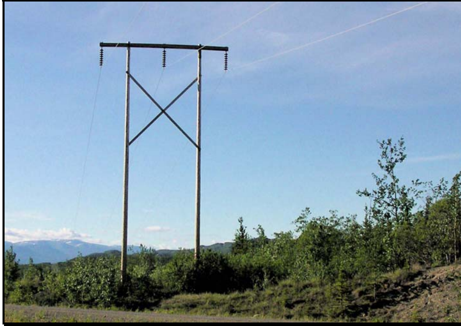
Figure 5.5-3 Typical 35 kV Pole Structure
