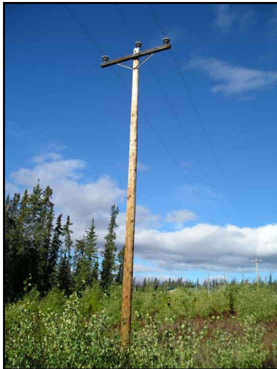
Figure 5.5-3 Typical 35 kV Pole Structure
