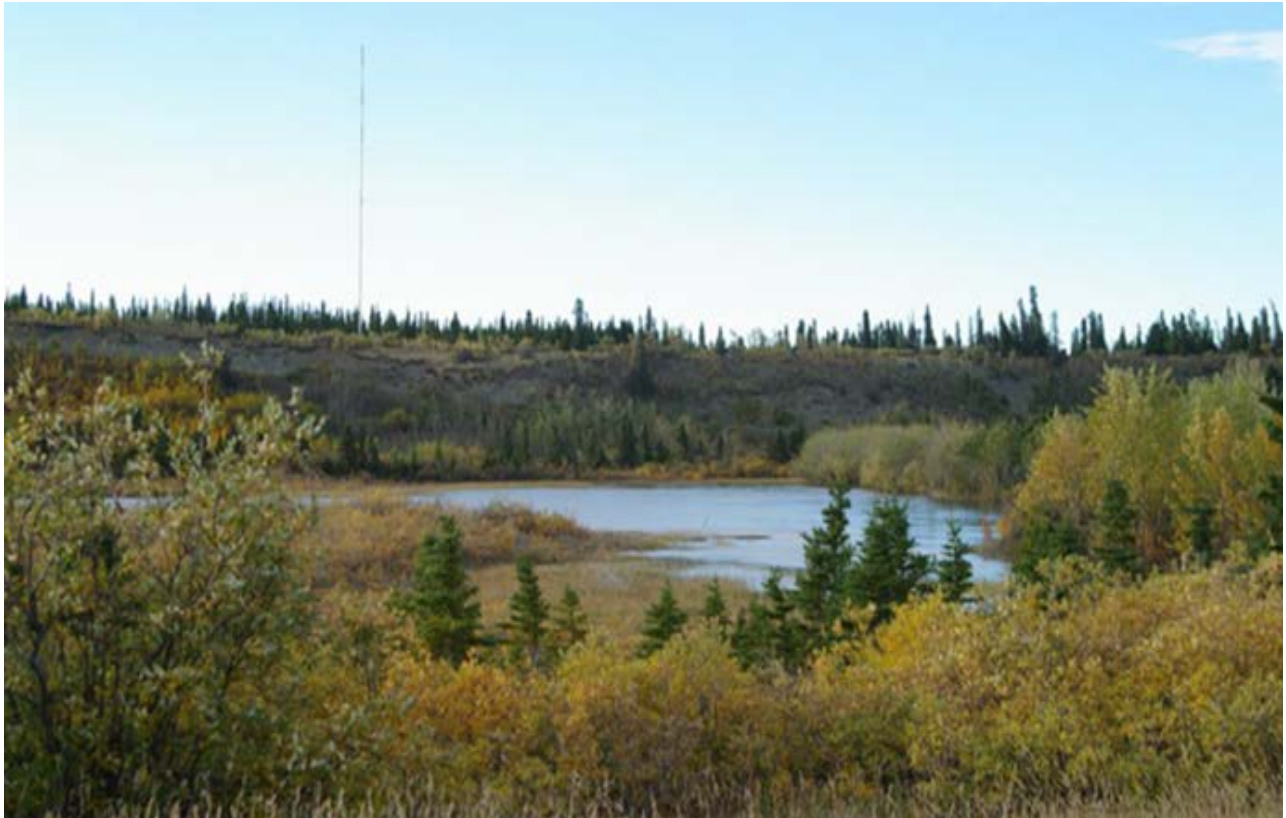
Figure 5 Met tower and wind project site looking south.
