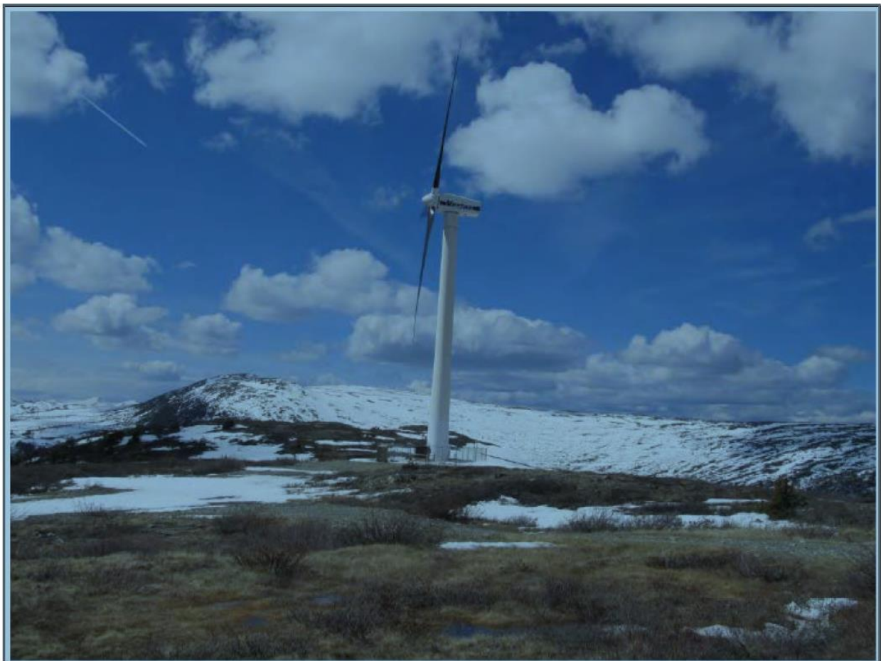
Figure 1: Photo of one of two existing towers and related infrastructure on Haeckel Hill.
