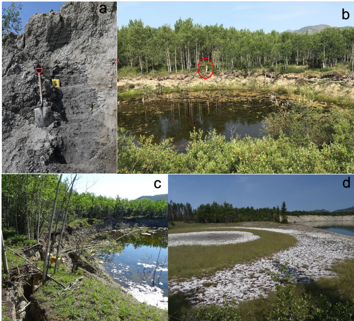
Figure 6.2 a) Interbedded glaciolacustrine silt and clay exposed in nearby Takhini River cutbank, b) typical thermokarst lake (note person circled for scale) with actively collapsing south-facing banks, c) fresh tension cracks and slumping along south-facing bank of thermokarst depression, and d) salt flats commonly develop in drained thermokarst lakes, such as this one along the banks of Takhini River.
