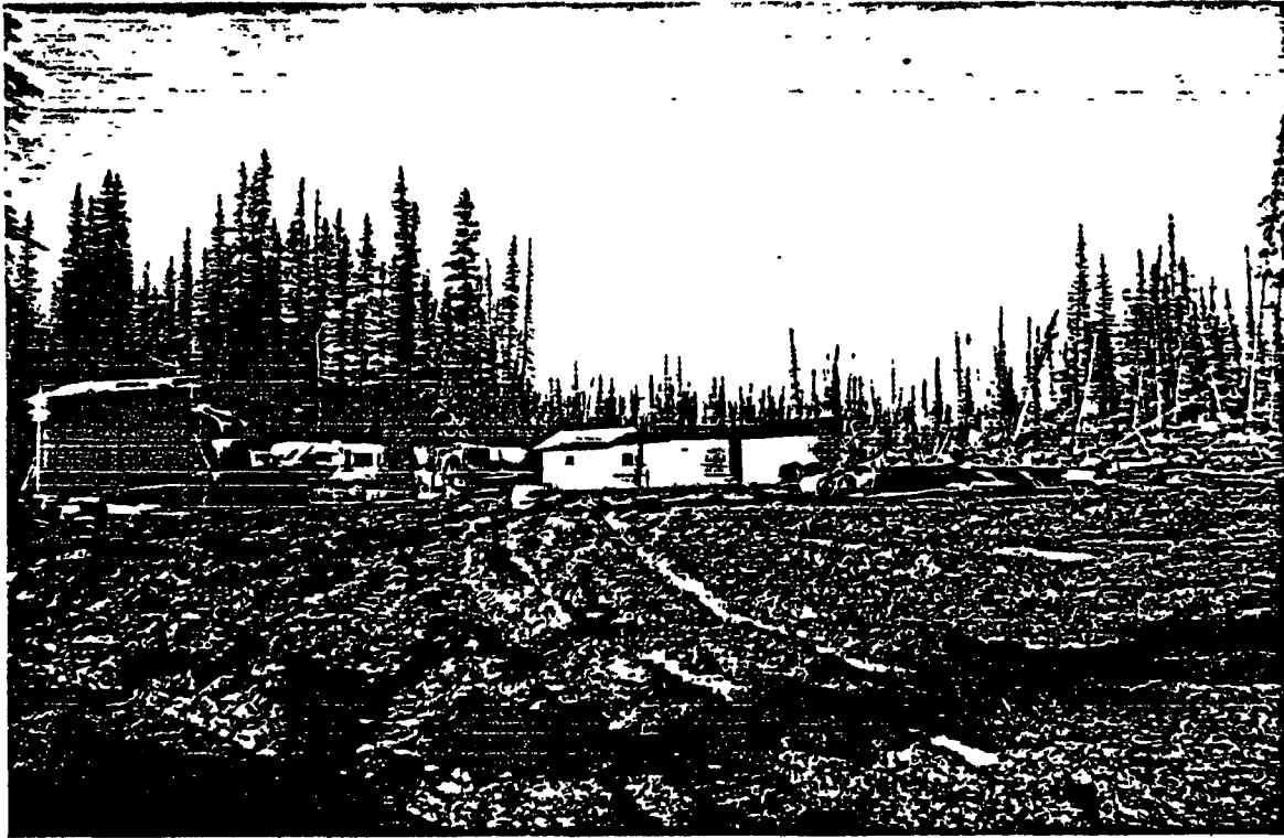
MINE CAMP INCLUDING 1 COOKHOUSE, 2 BUNKHOUSES, TRAILER, TOOL SHACK AND MISCELLANEOUS EQUIPMENT.
