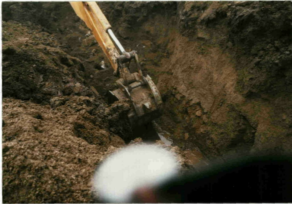
Backhoe trenching decomposed in-situ bedrock. Vein and wallrock alteration dipping at 30^\circ can be seen to the lower right of backhoe bucket.
