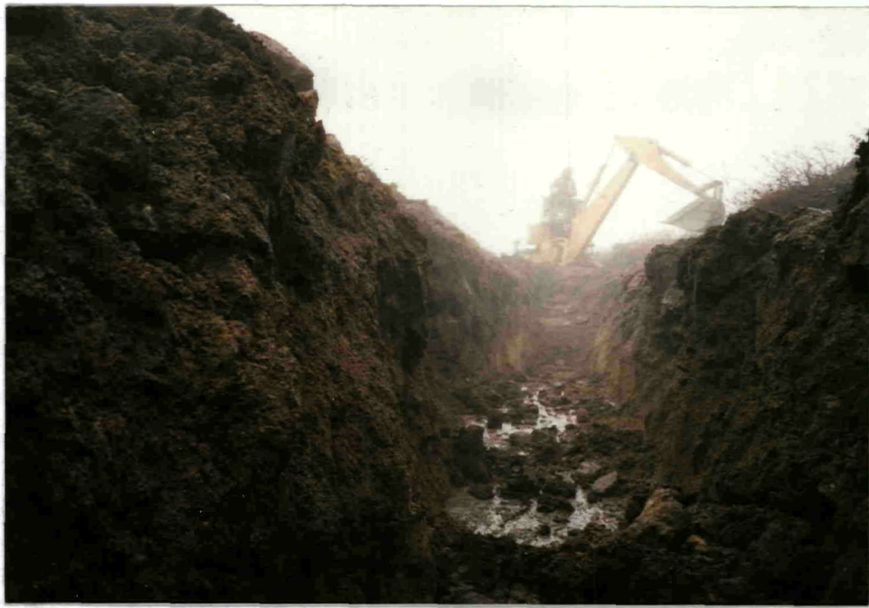
Trenching to bedrock through thawed ground.
