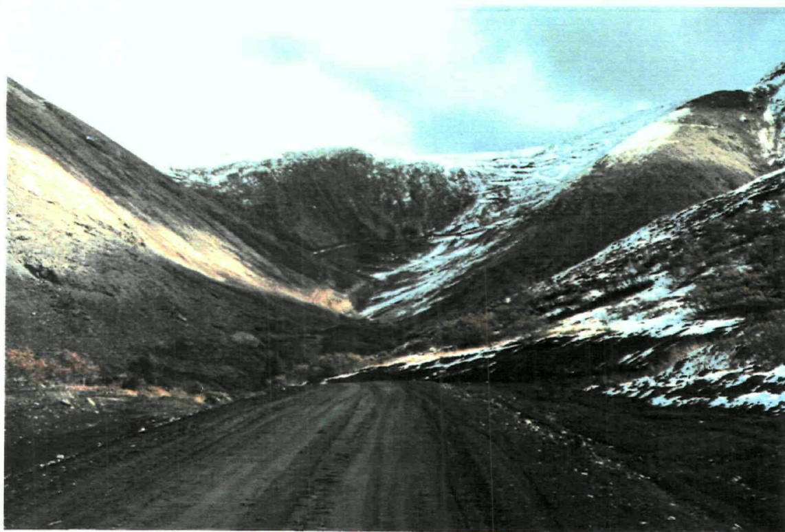
Portal access road (in distance) in early October, looking from Pass road north of camp
