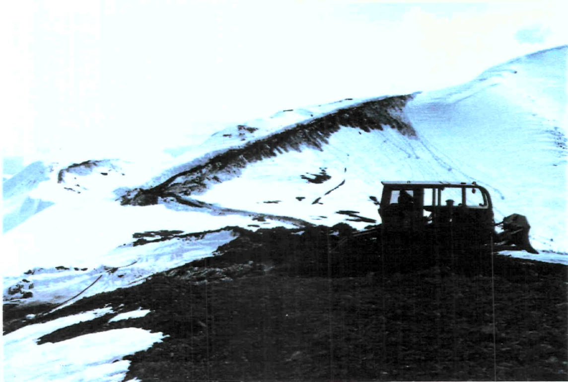
Diamond drill pad construction - Groundhog Zone
