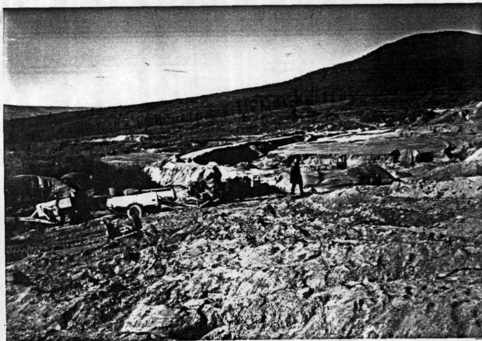
Crushing and grinding ore samples on Reef Claims (From left: John Deere bulldozer and trailer with sample barrels; test mill; Cat in background trenching decomposed bedrock.)
