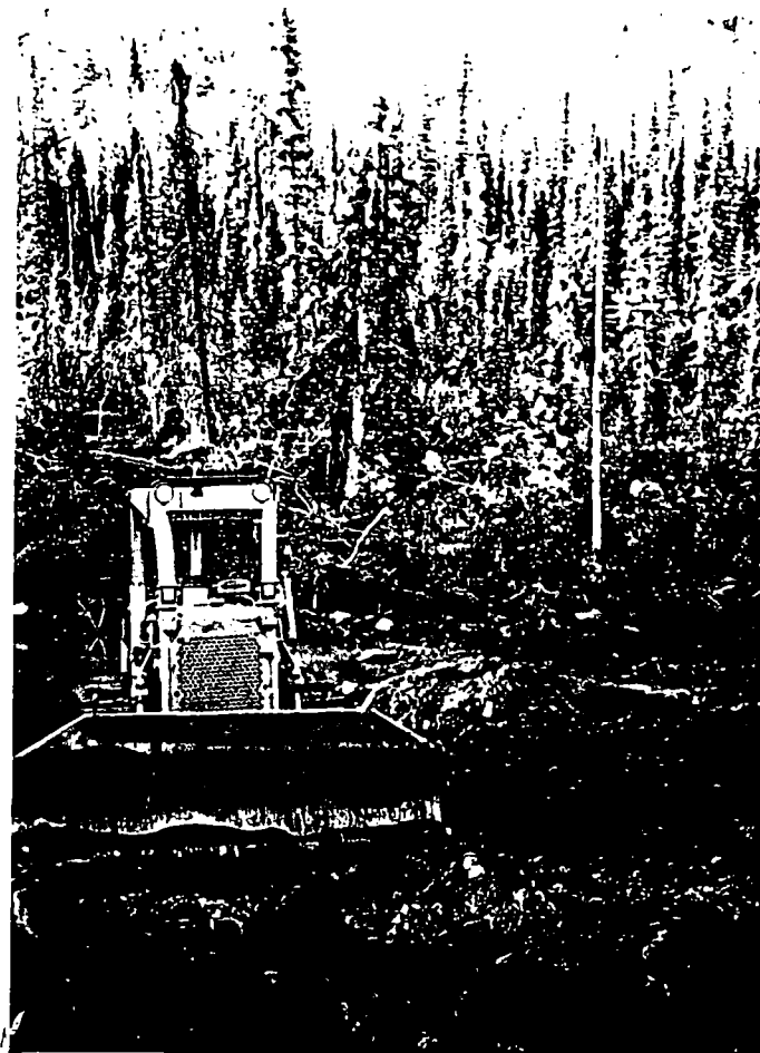
Stripping vegetation covering and insulating permafrost in placer creek.
