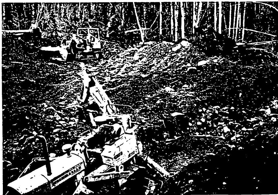
Backhoe and loader trenching.
