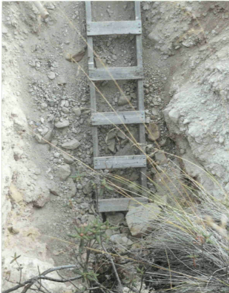
11. Test hole # 1. Approximately 7 feet deep.
