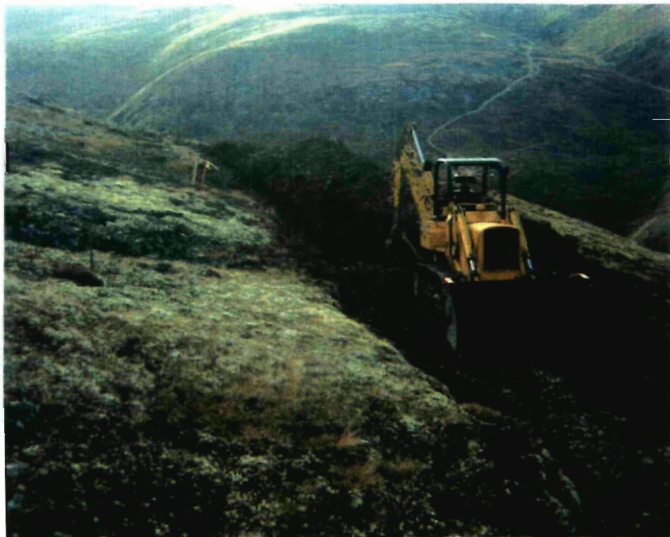
Figure 8. (a) Road construction to Sunrise adit (next to CAT) (b) Trenching T94-1.
