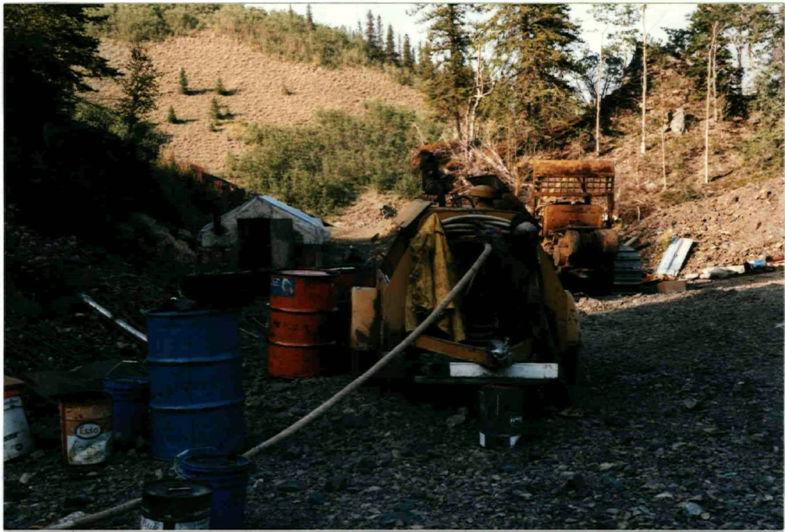
↑ COMPRESSOR SITE LOOKING NORTH
