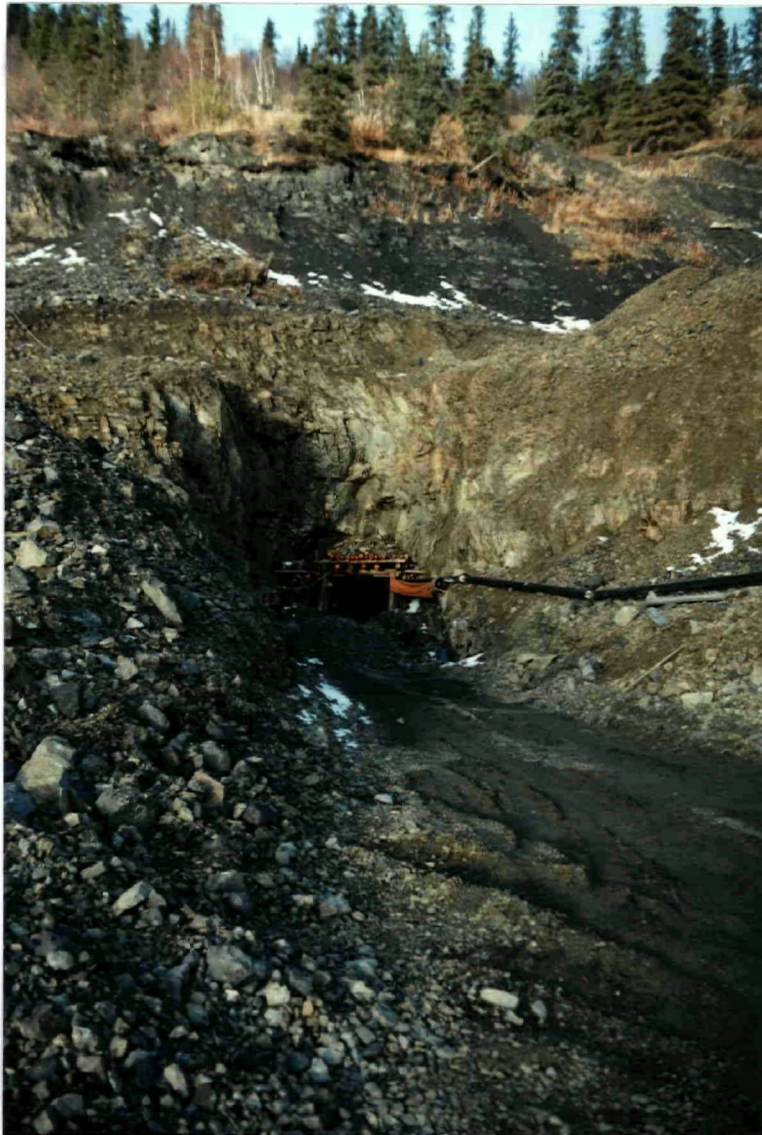
PORTAL / DRIFT LOOKING WEST
