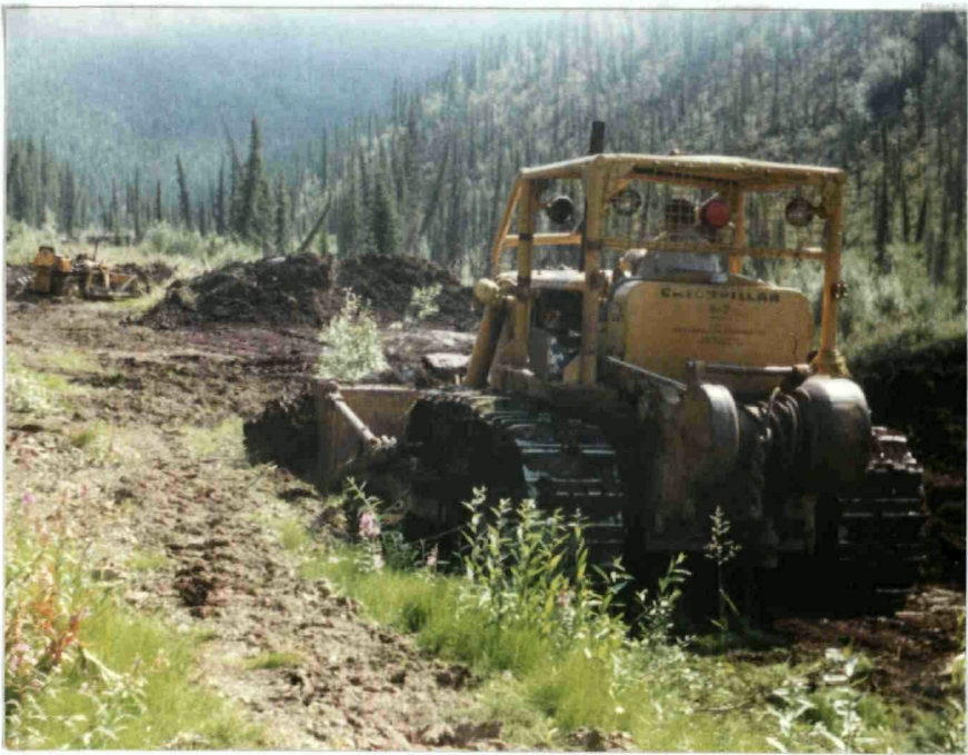
"Trail pushing" creek to right of cat work ▶
