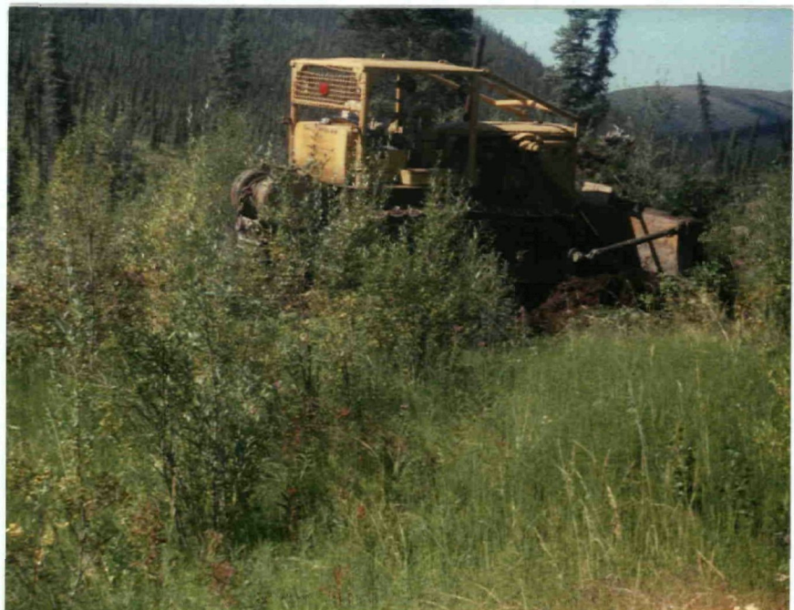
Pushing trail upstream bypassing swampy area ▶
