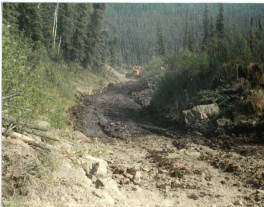
Pad sites along trail bottom end of gulch ▶
