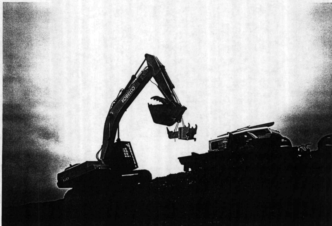
KOBELCO HOE -with ripper
