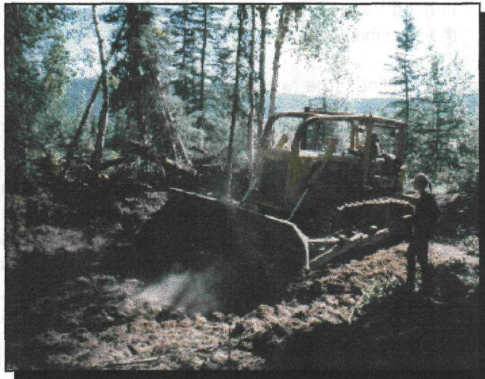
Spreading overburden to restore trench site
