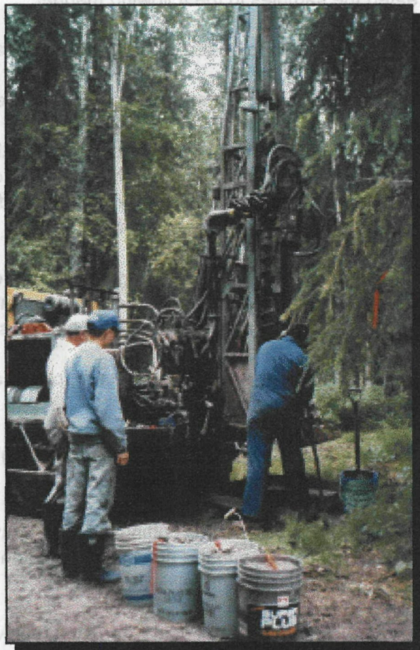
Drilling with 6" auger drill on the property
