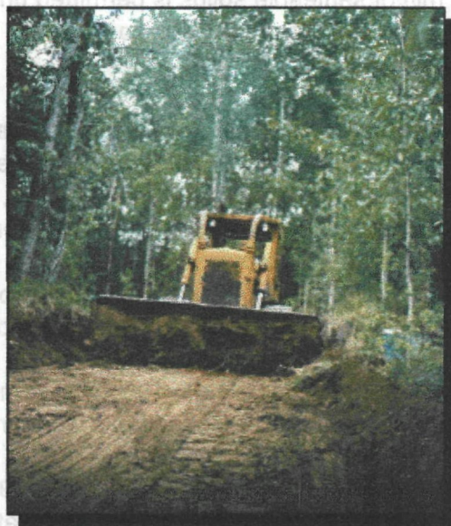
Preparing an access ramp
