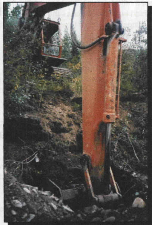
Trenching with the excavator
