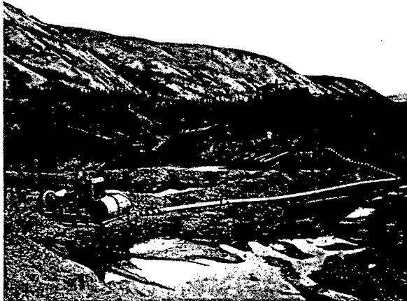
Sky Dawn Mining sluicing a contained cut along the left limit of the Indian River.
