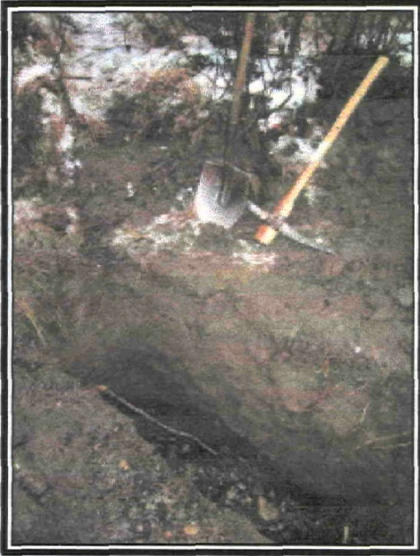
A hand excavated trench in the bank adjacent to the creek channel.
