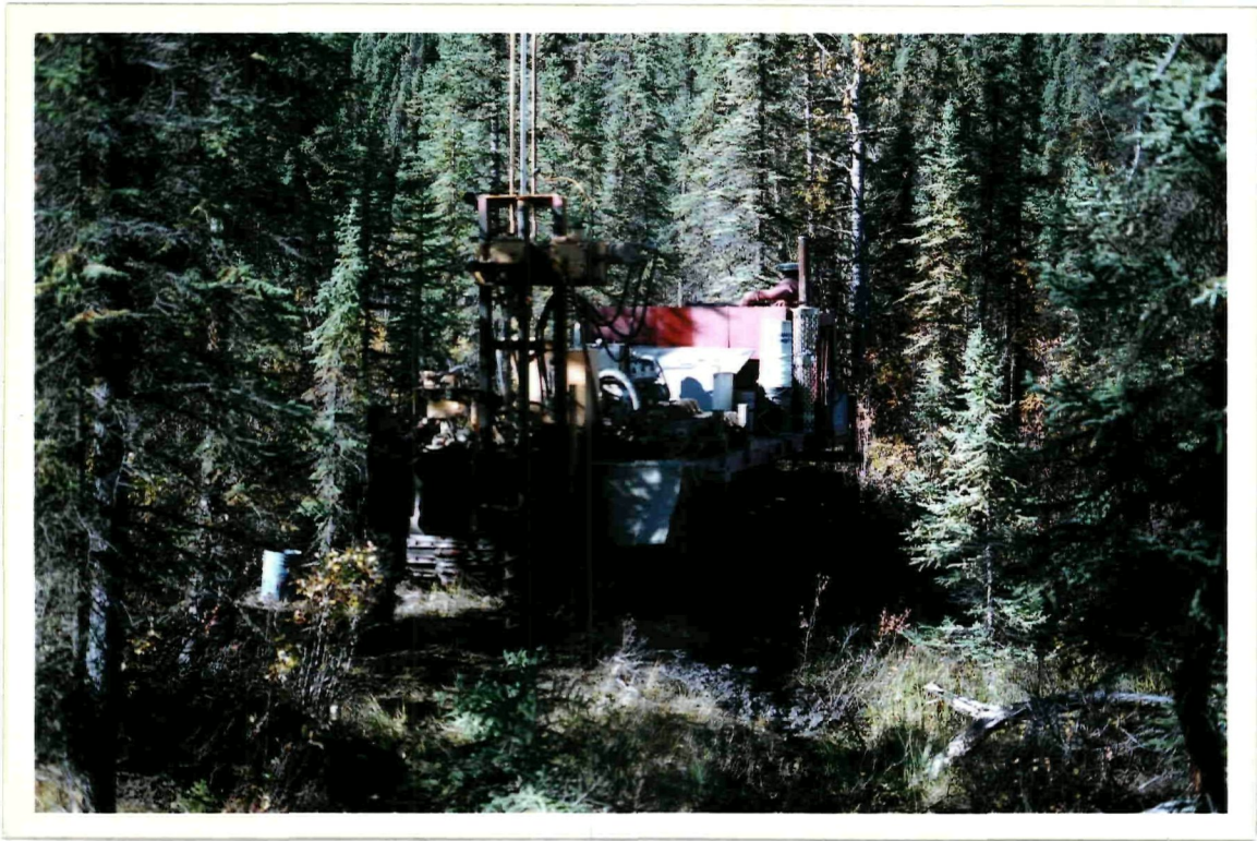
DRILLING HOLE #2 , GORING CK.
