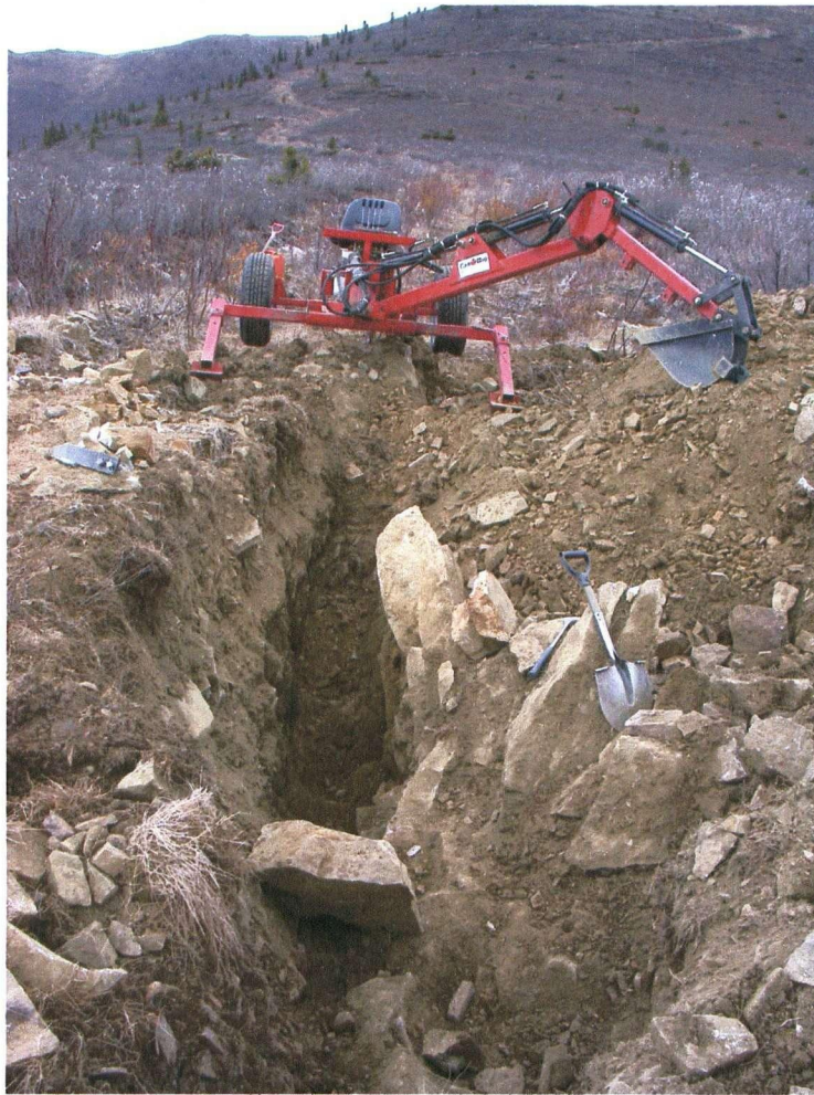
Can Dig Excavator Digging Black Fox Trench
