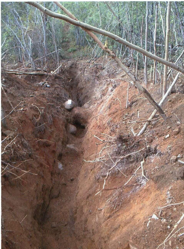
Photo 3. South end of Trench 1.
