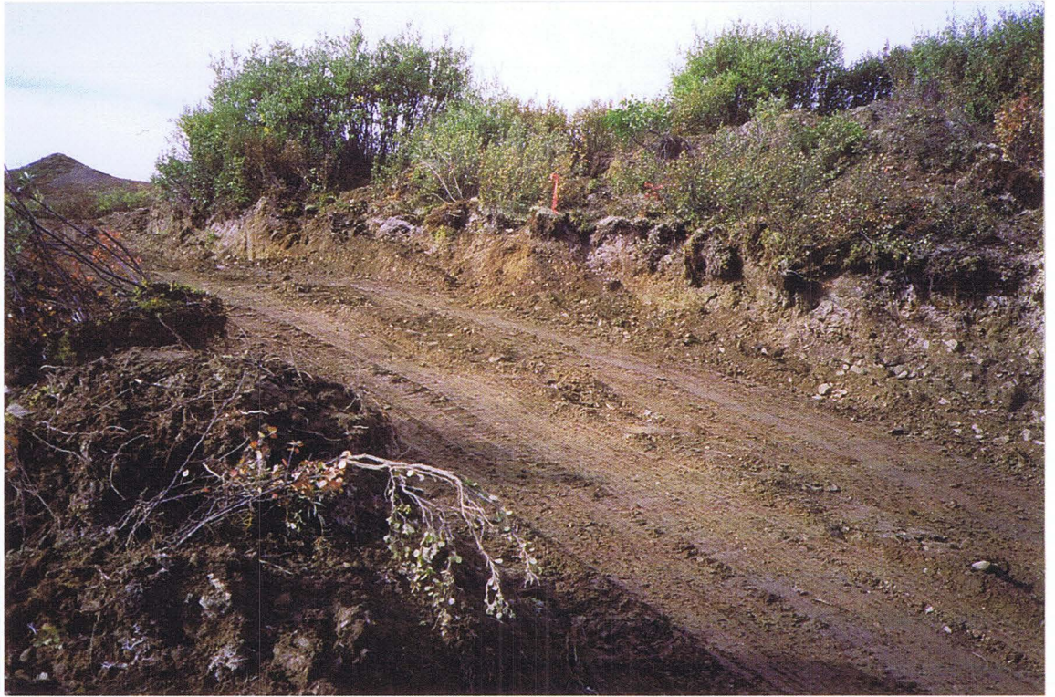
TRENCH 11 (bench re-contoured for equipment access)
