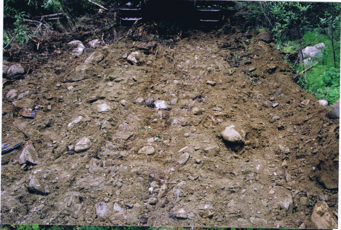
Reclamation done with dozer
