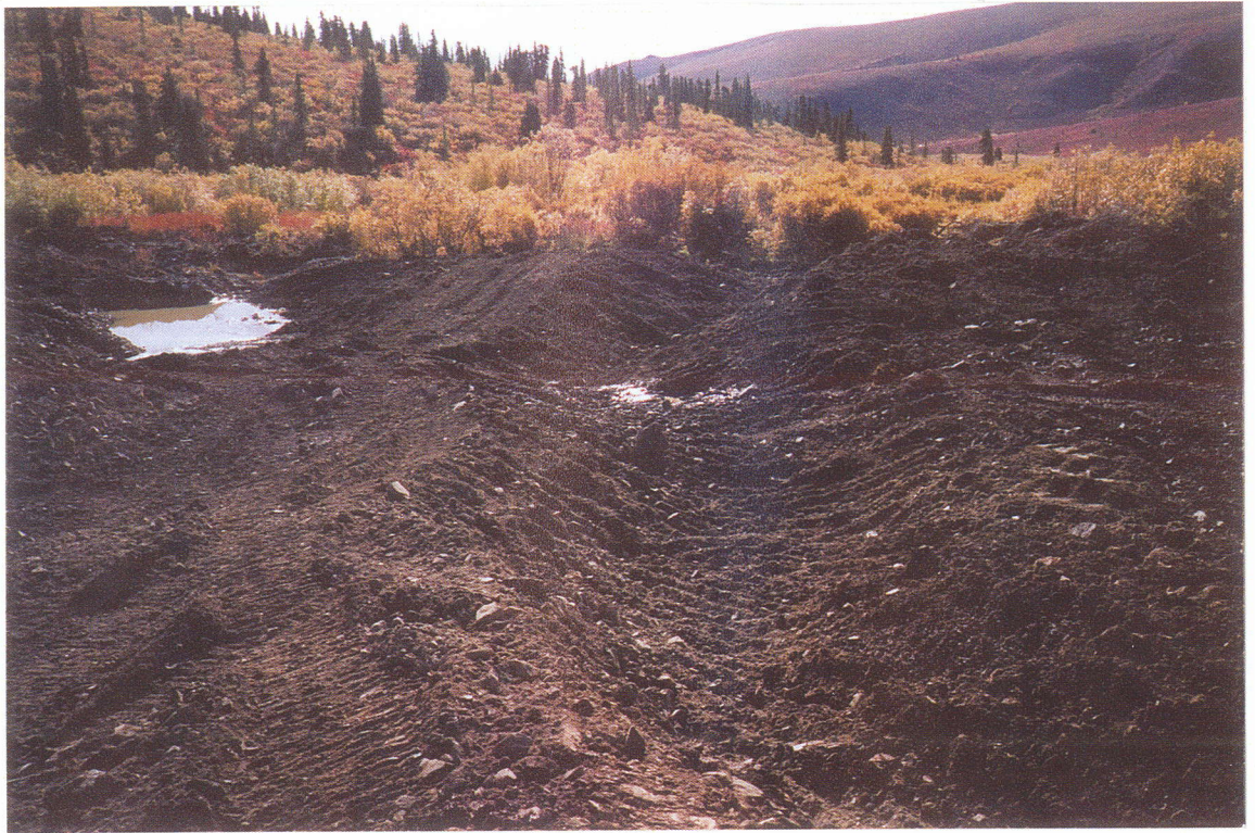
HOLE # 1, LEXIE CREEK CHANNEL and PARTIAL SETTLING POND RECLAMATION AREA
