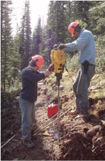
Figure 13. Trenching crew drilling shot holes.
