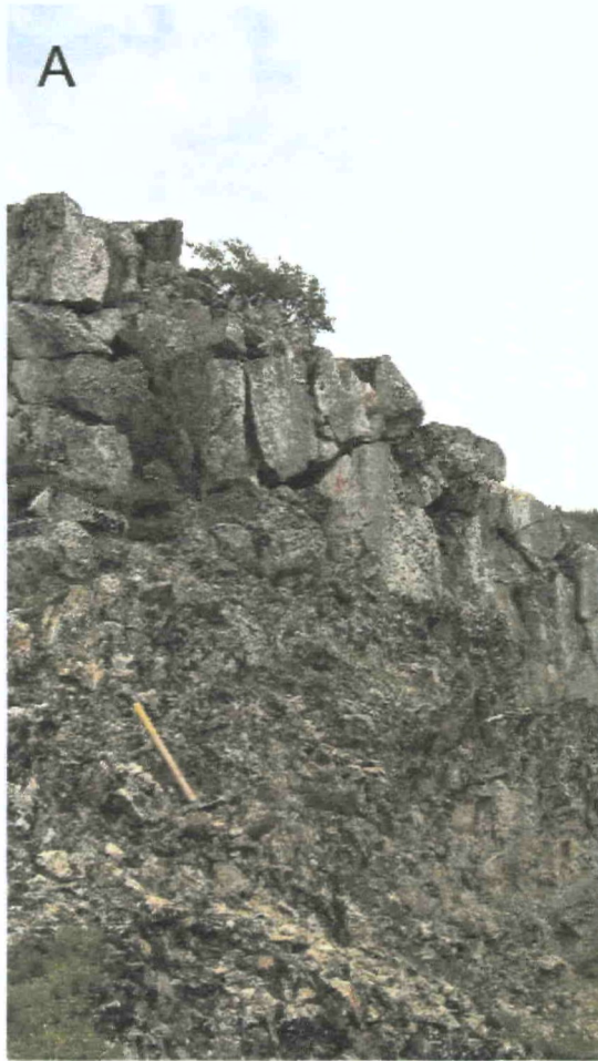
Aplitic granite dyke intruding strongly altered granodiorite unit (foreground). The dyke intrudes at a sub-vertical orientation.
